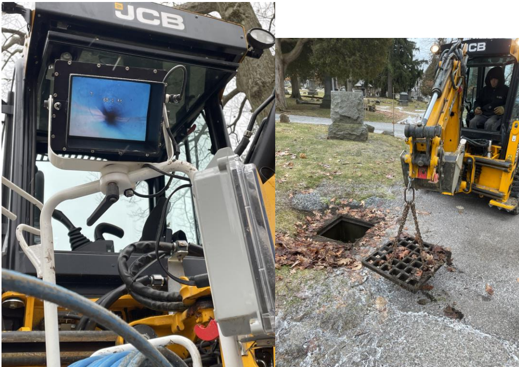
Exploring stormwater lines at Lakeview Cemetery (pictures above)
