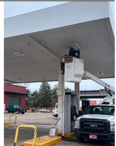
Replacing lights at 645 Pine gas canopy
