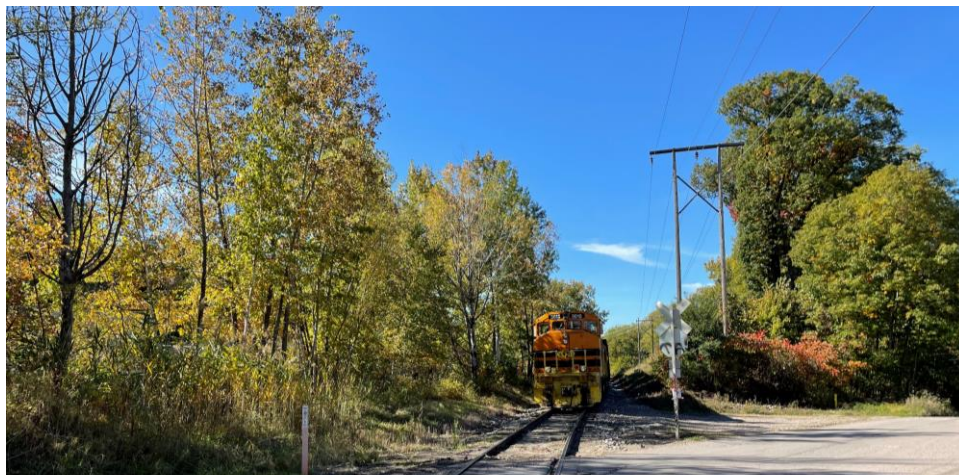
Railroad Crossing Safety Improvements
