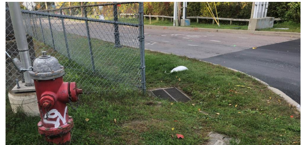
Drainage / Utility Relocation and Improvements
