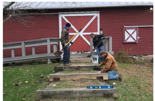
Park Facilities team repairing the steps at Schmanska Park
