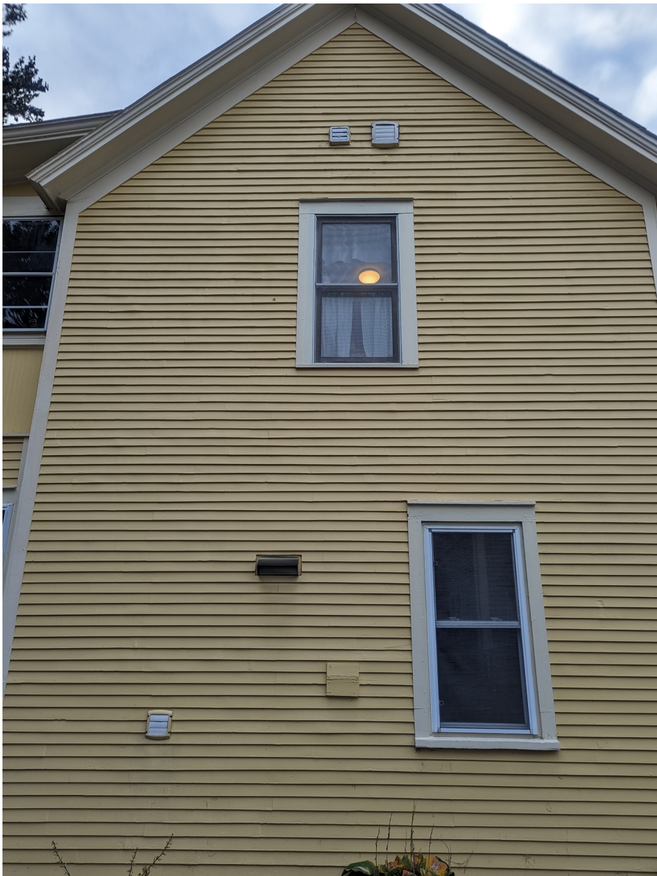
Figure 3:E wall F11Kitchen; F12 Kitchen
