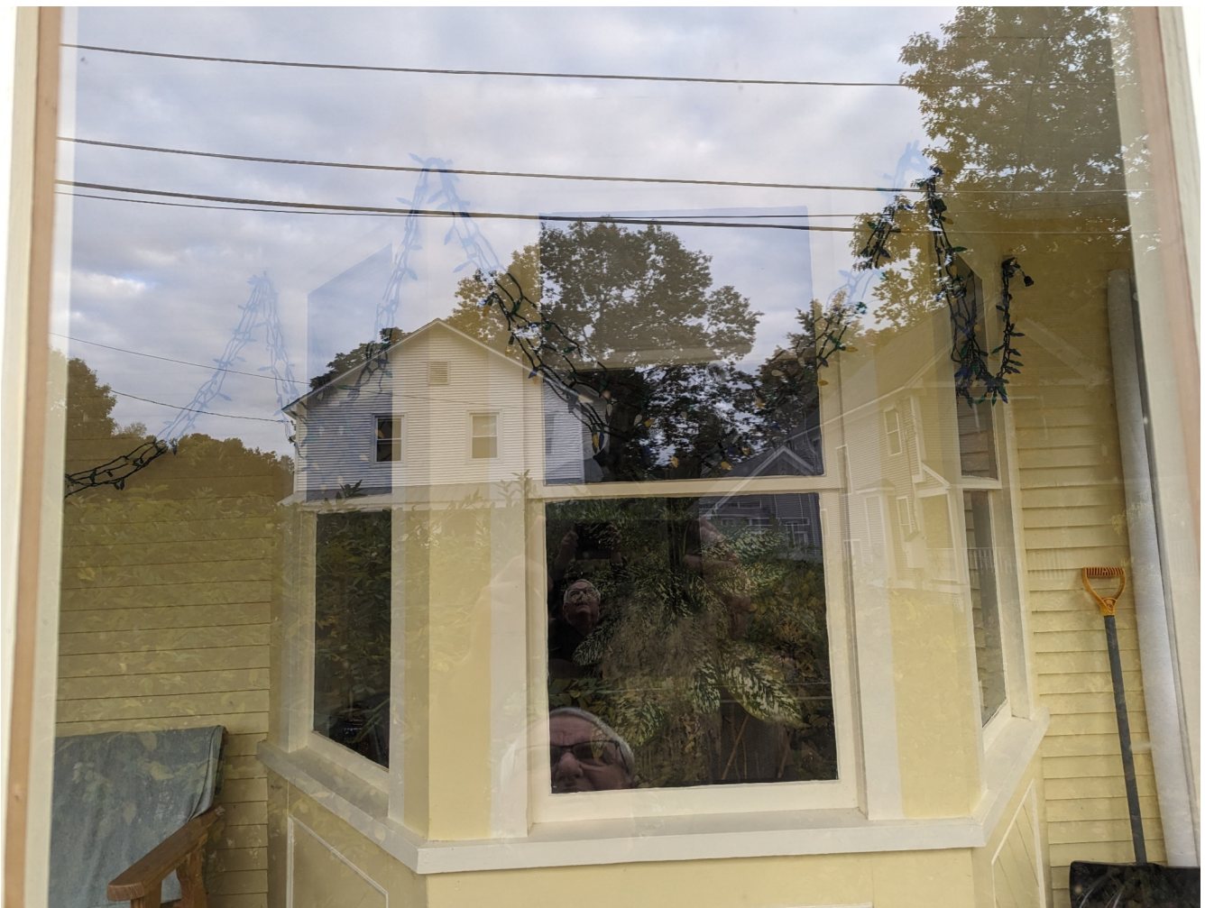
Figure 2: 1st floor N wall Bedroom (3) 1-3
