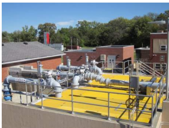
Figure 6: Rushville WWTP Constructed CMF System
