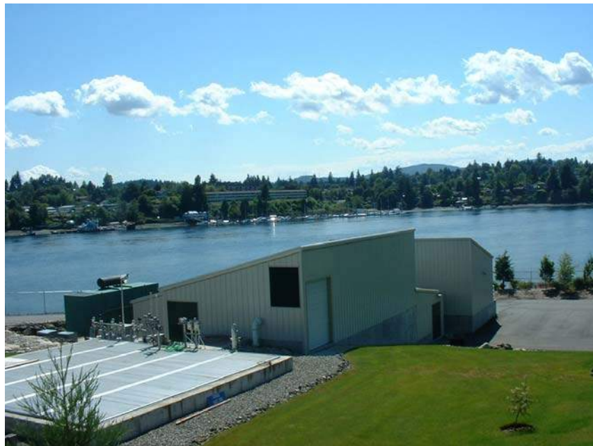
Figure 10. Bremerton East Side Treatment Plant.
