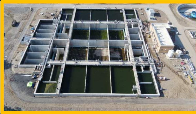
Biological Nutrient Removal S2EBPR + 4-stage Bardenpho
