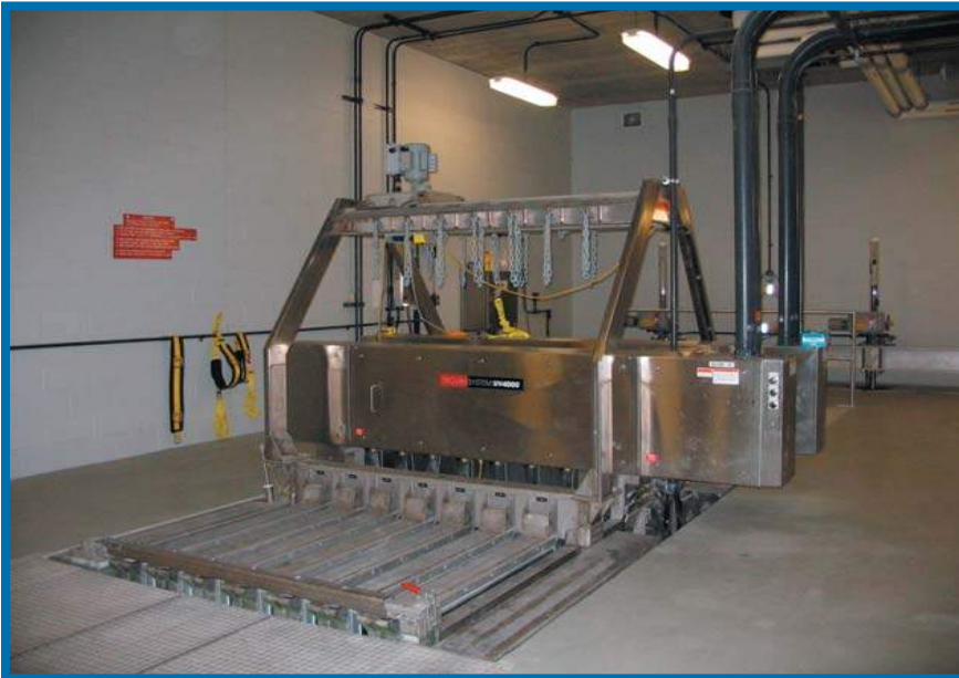
Trojan UV 4000 Disinfection Unit
