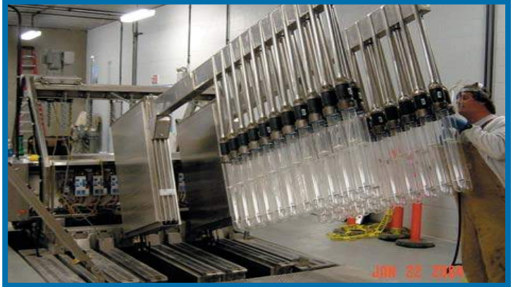
Installation of UV Disinfection Lights
