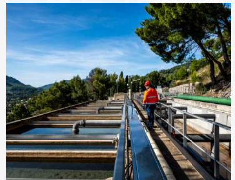
WATER AND WASTEWATER TREATMENT PLANTS
