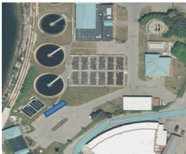
Figure 2. The location of Blue PRO pilot (blue box) at Burlington treatment facility
