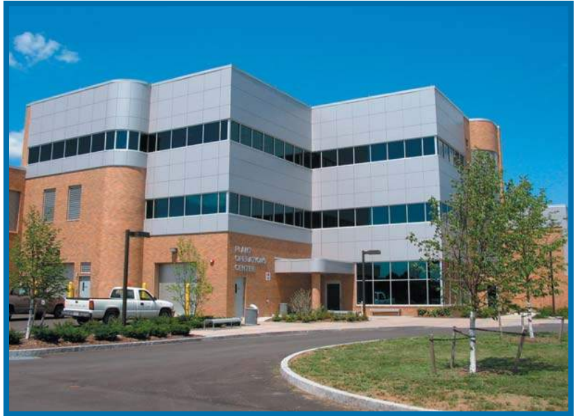
Plant Operations Center
