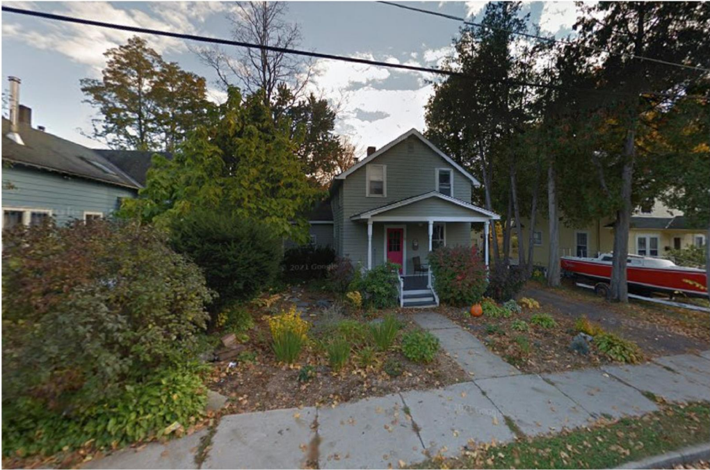
EXISTING NORTH ELEVATION IMAGE
