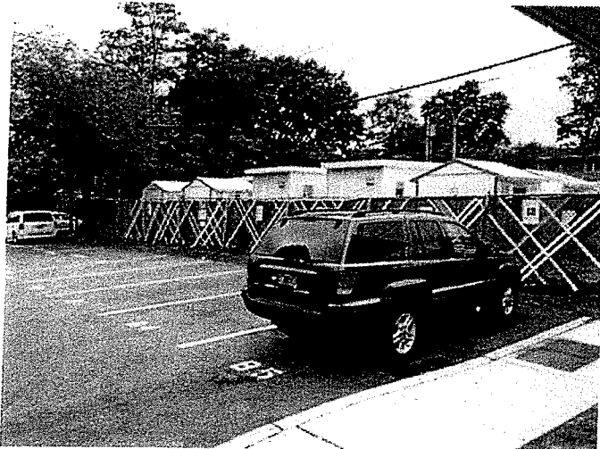
Elmwood Community Shelter (ECS), looking NW
