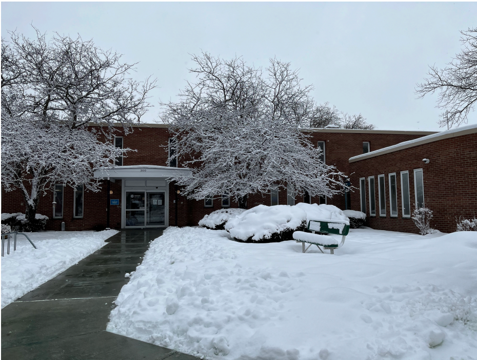
FLYNN AVENUE ENTRANCE
