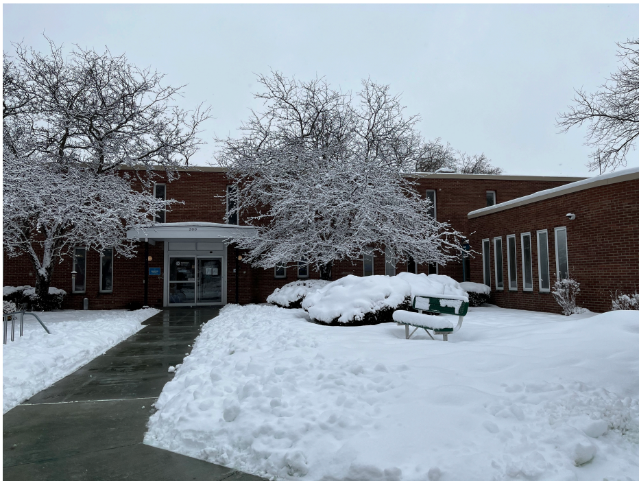
FLYNN AVENUE ENTRANCE
