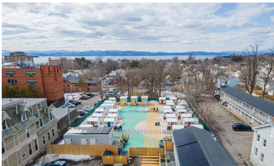
Aerial Image of Elmwood Community Emergency Shelter
