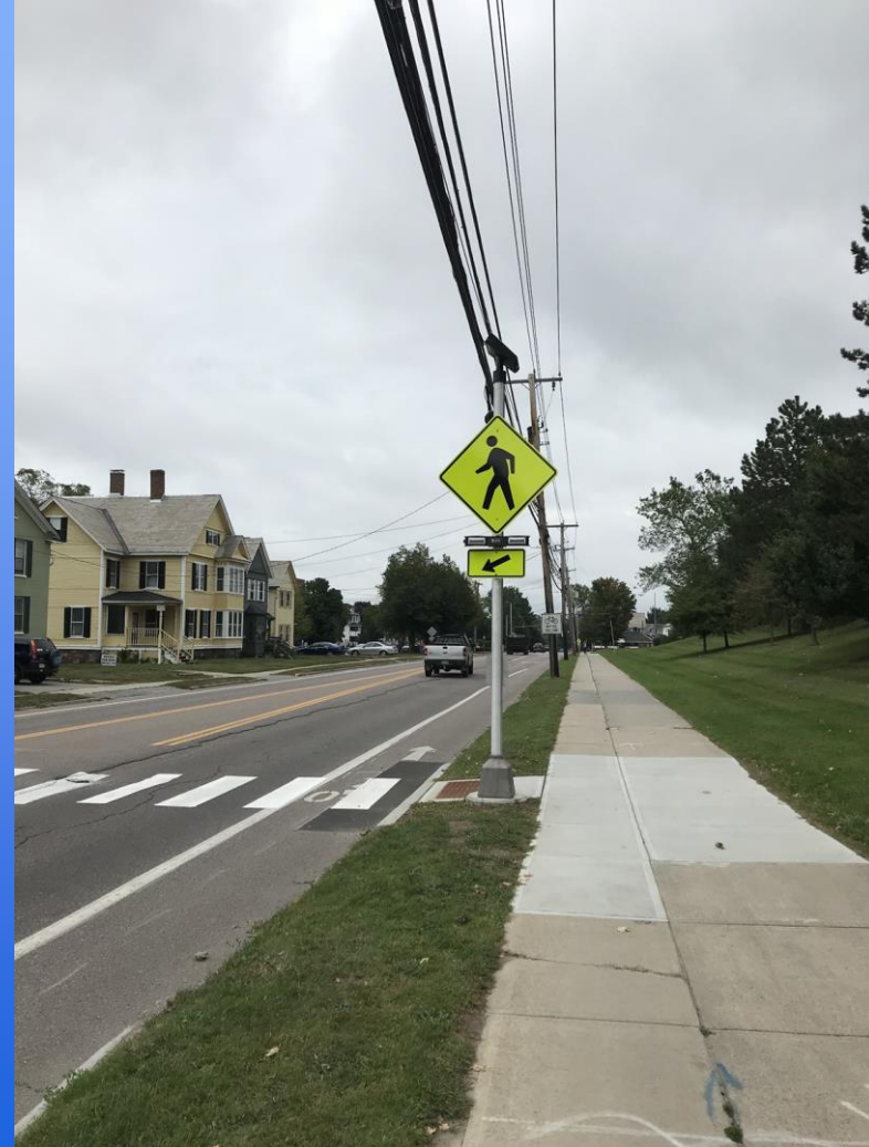
FLETCHER PLACE CROSSWALK W/ RRFB 2018
