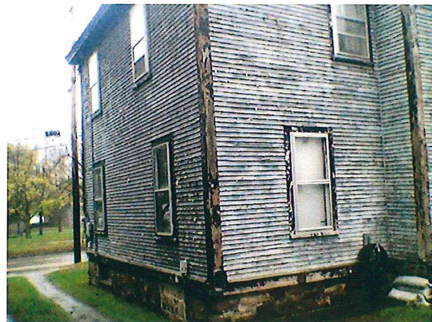
SOUTHEAST VIEW - EXISTING
