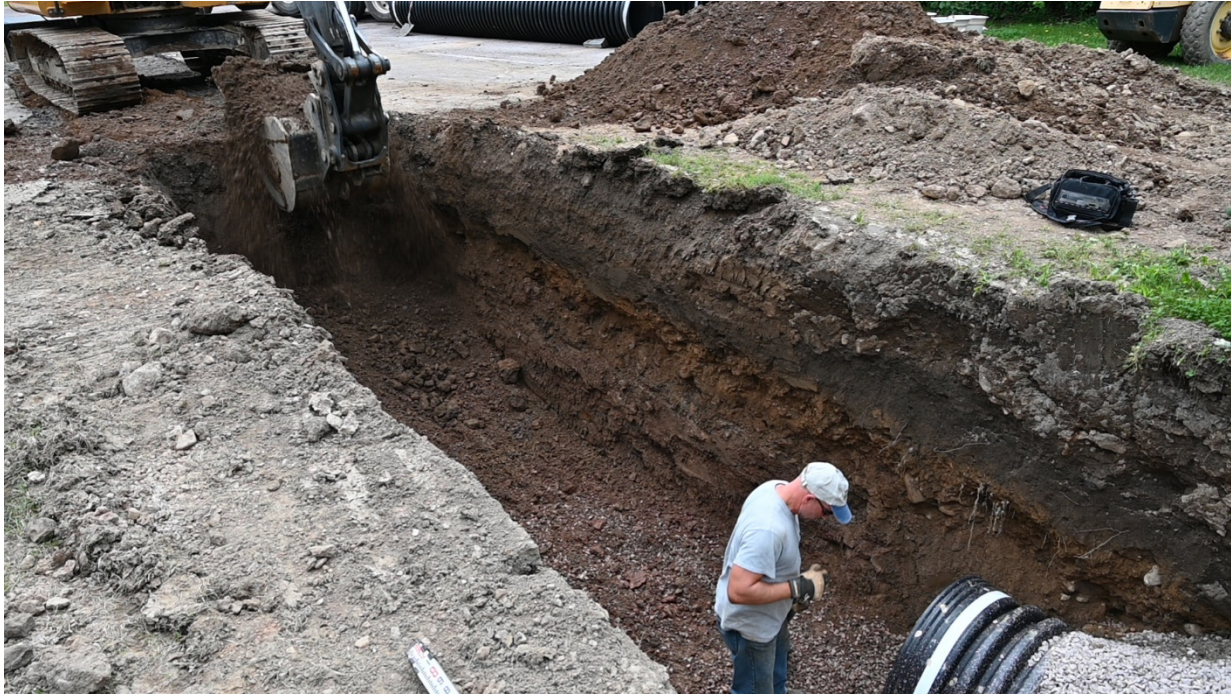
Figure 18. General view of the trench excavation (western end), looking southeast (2021).
