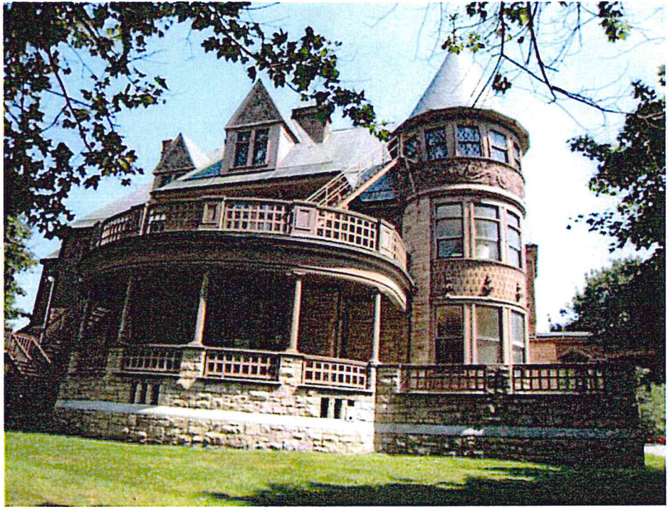
West Elevation, from the south
