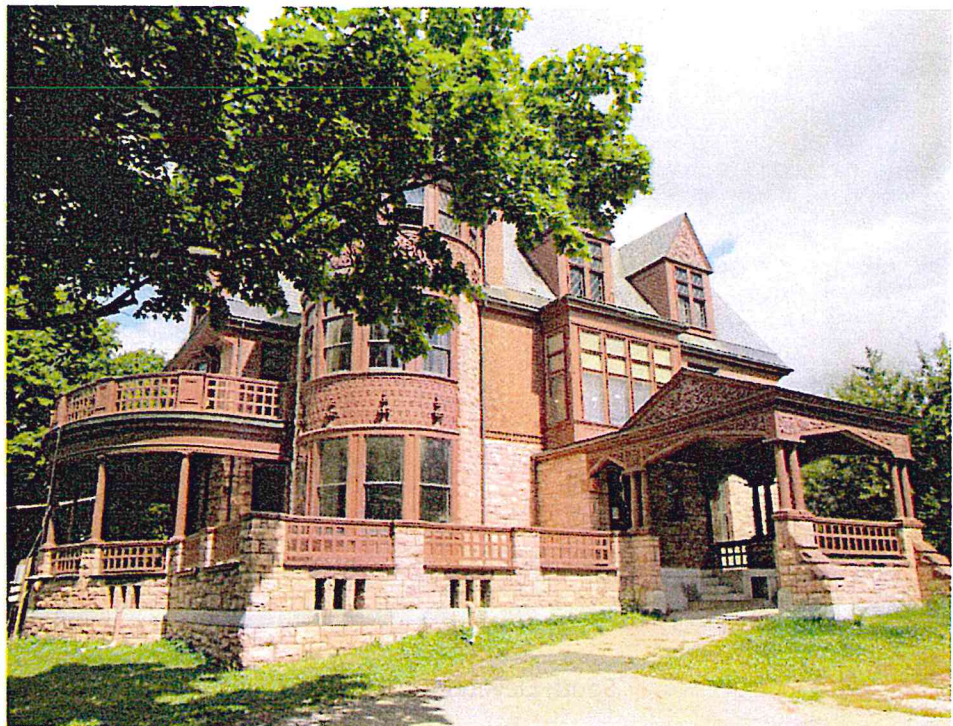
View from the Southwest
