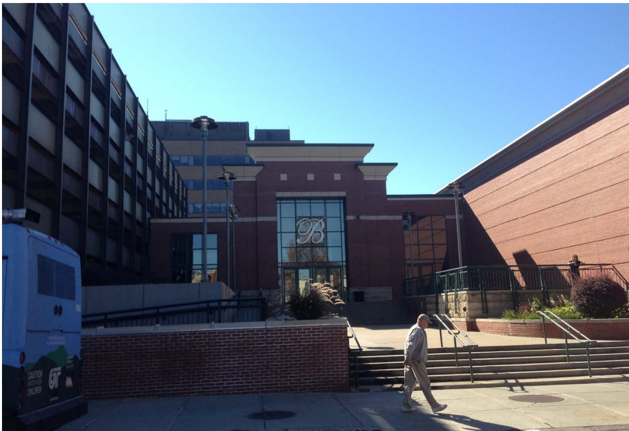
3.8 PINE STREET AT CHERRY STREET - LOOKING SOUTH
