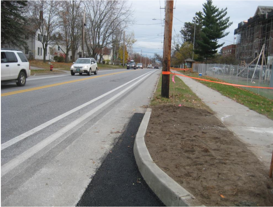
FIGURE 11. LOOKING SOUTH FROM NORTH ROAD EXIT
