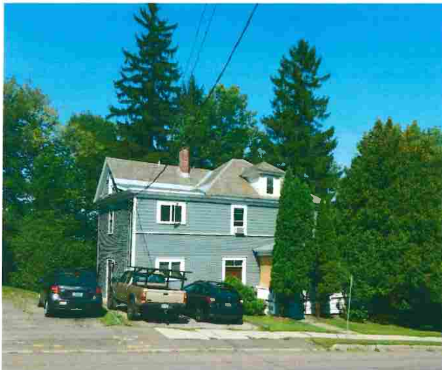
Figure 25. Looking west at 460 Colchester Avenue, 2016.
