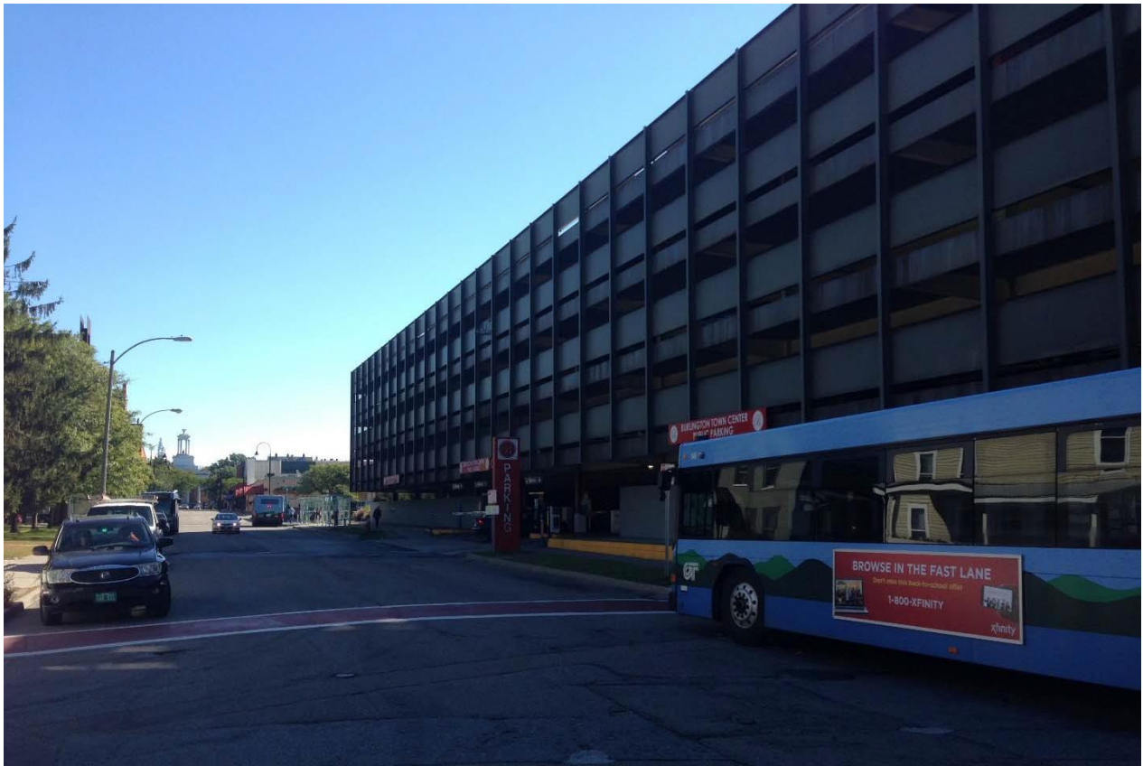
3.7 CHERRY STREET - LOOKING SOUTHEAST
