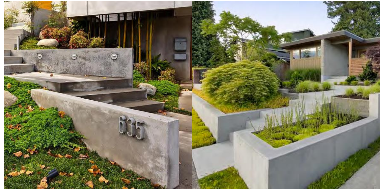
POURED CONCRETE WALL
