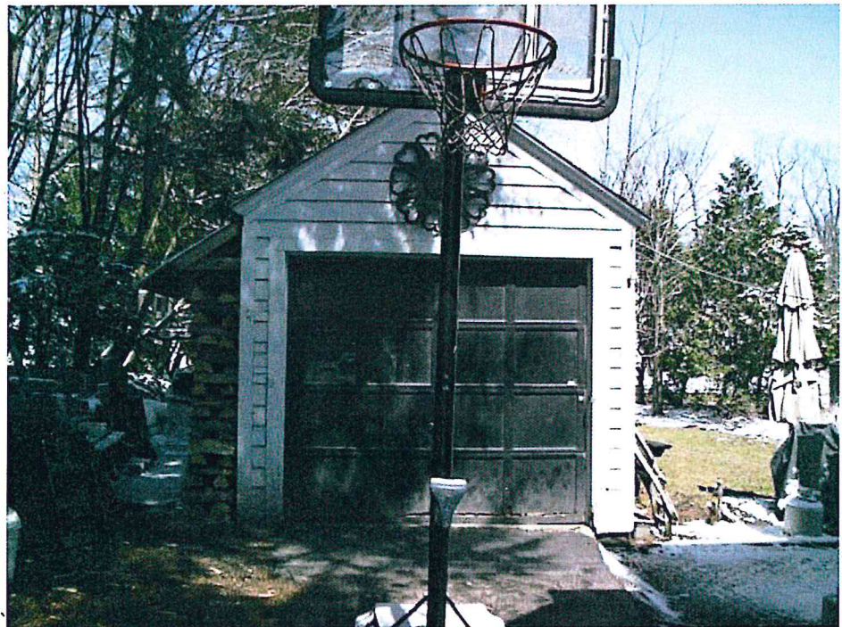
South (Front) Elevation @ Garage looking North
