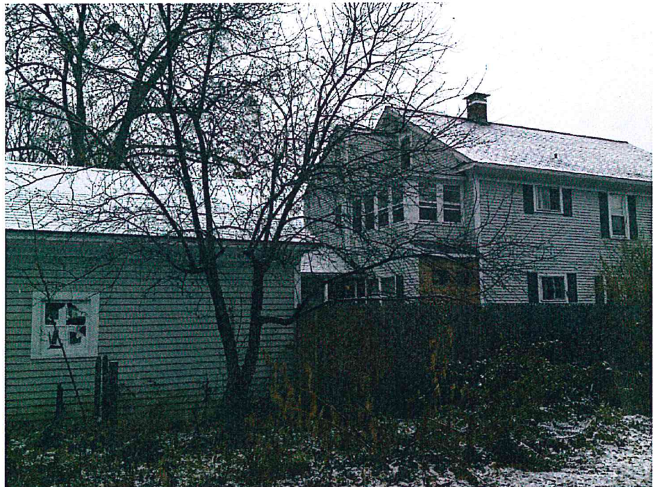
Side Yard looking East
