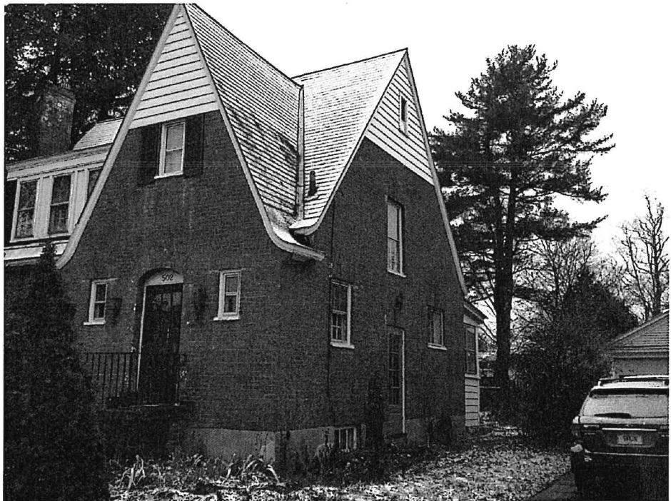
East Elevation Looking Northwest from North Street
