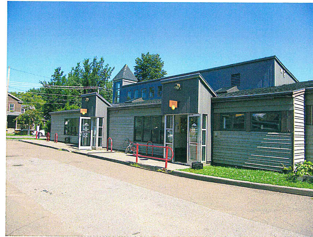
VIEW LOOKING NORTH FROM PARKING LOT
