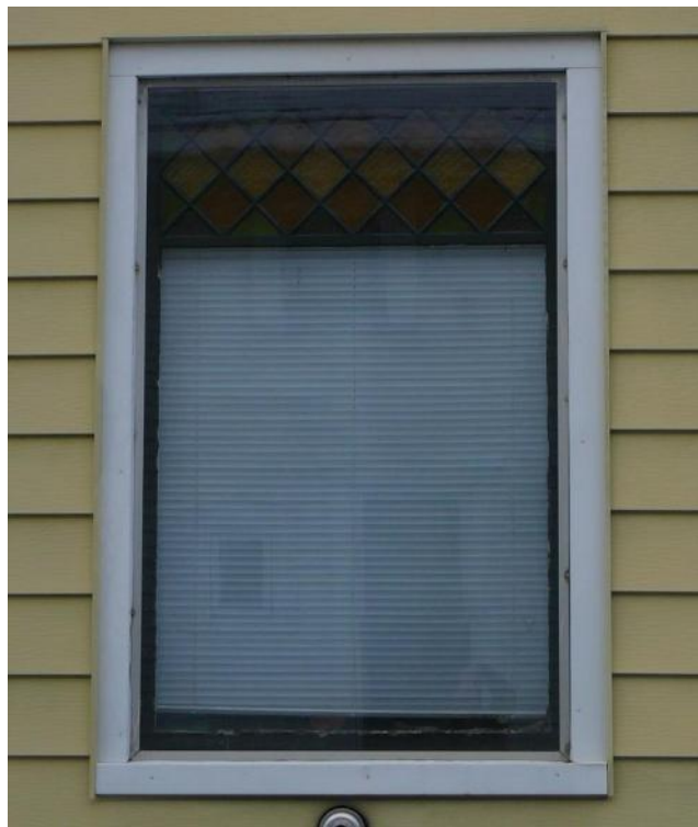
Figure 84. View of window with stained glass transom on tower of south elevation of 19 George Street.
