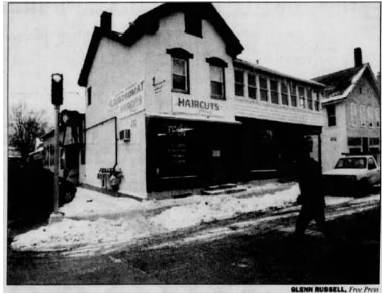
Figure 93. View northeast of the two buildings removed for Victoria Place; #80-82-84 Pearl Street (left) and #86-88-90 Pearl Street (right); note structures extending to the north (behind) #80-82-84 Pearl Street. ( Burlington Free Press January 3, 2001).
