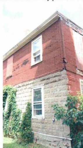
Looking northeast at rear wall of addition.
