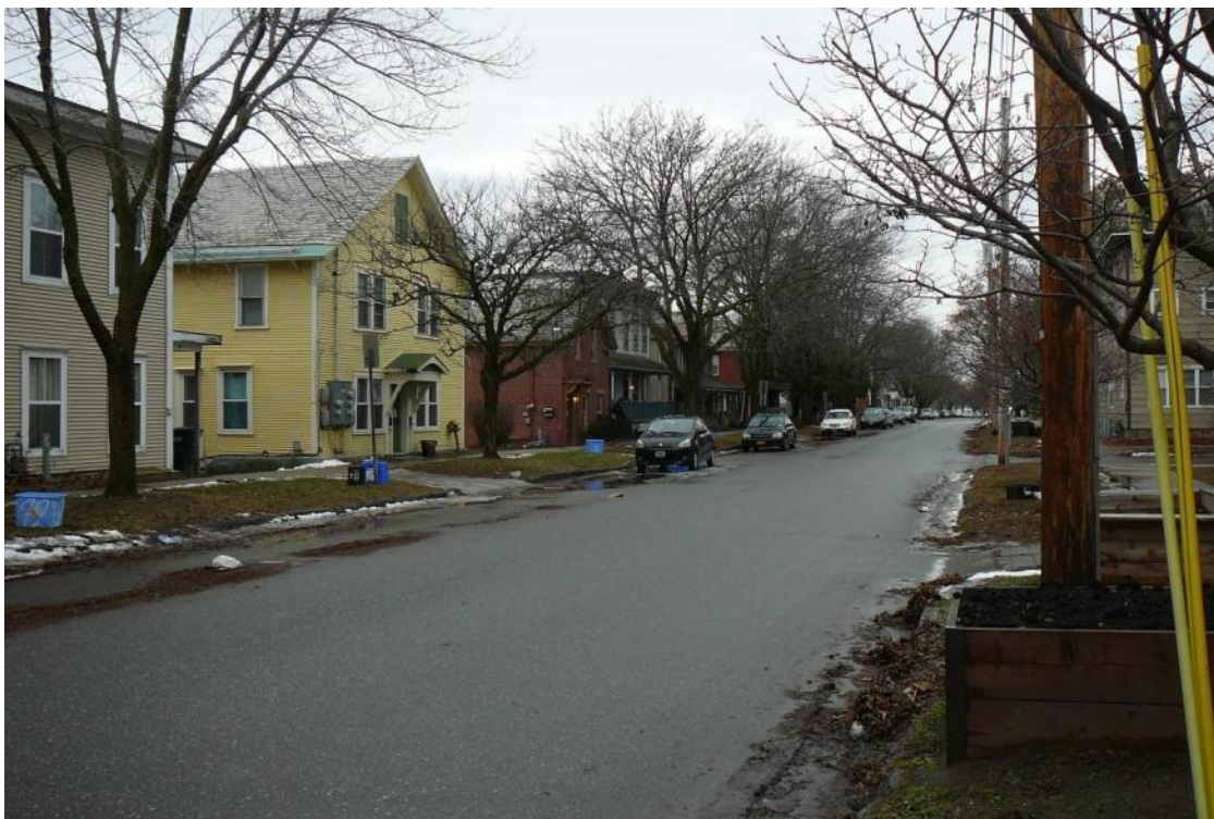
Figure 19. View southwest of buildings along the south side of Monroe Street; (right, foreground to background) 77-79, 73-75, 69, 67 Monroe Street.
