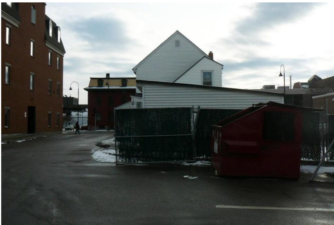
Figure 40. View south of north elevation of 64 Pearl Street.
