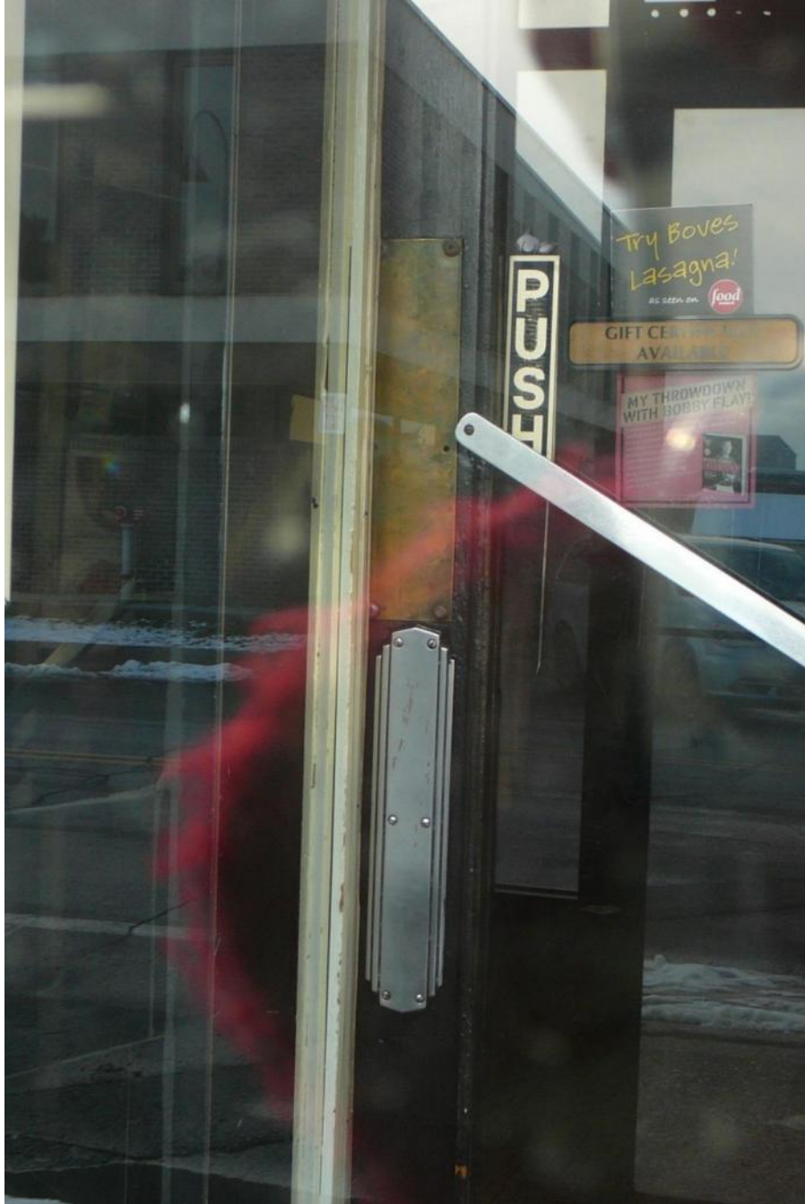
Figure 62. View of hand plates on main (central) entry door within glass enclosure at 64 Pearl Street.
