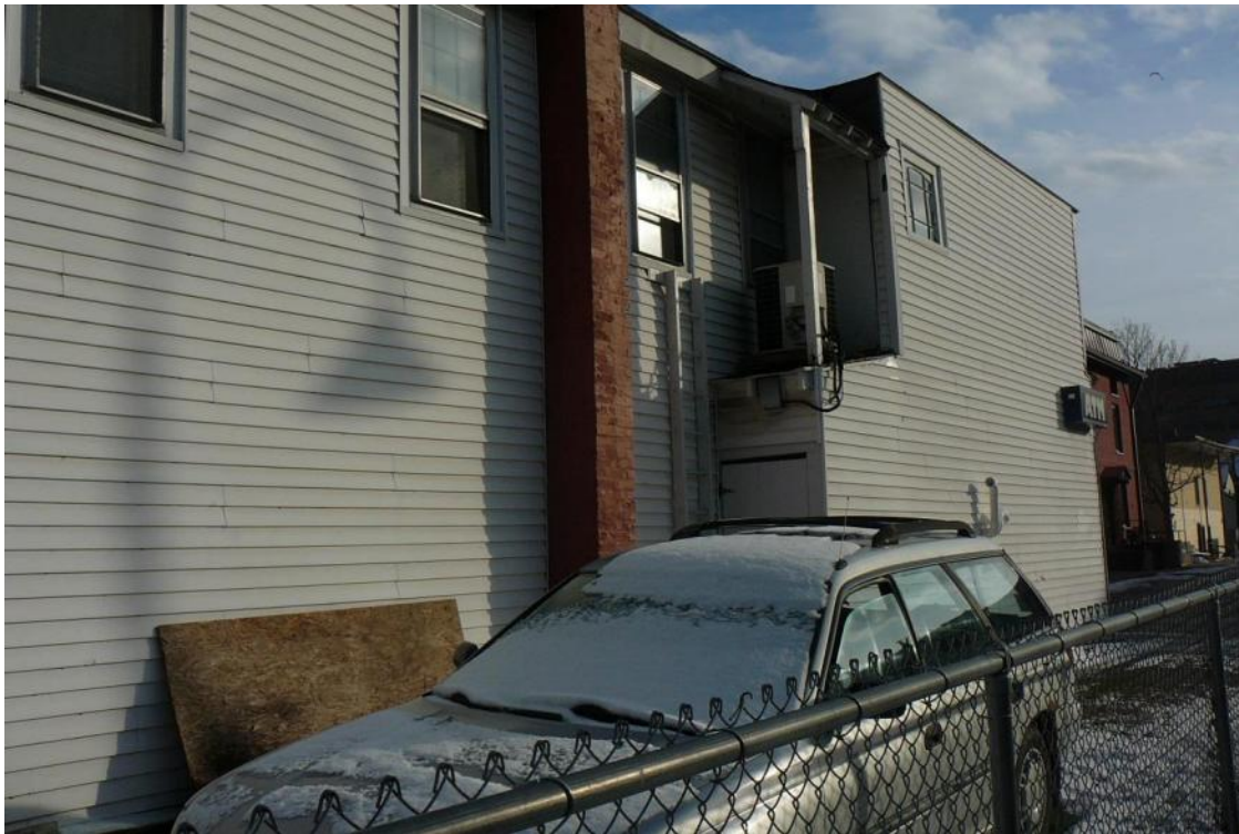
Figure 43. View southeast of west elevation of 64 Pearl Street.
