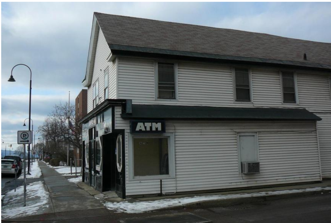
Figure 45. View west of east elevation of 64 Pearl Street.
