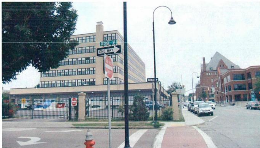
Looking from 3 George across George Street and east on Pearl Street with Federal Building and its parking lot on left and large new building on the corner of St. Paul Street on the right.
