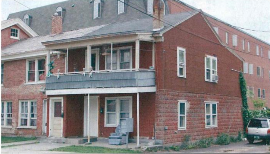
Looking southwest at front and north end of cinder block addition. Front and upper floor have asphalt sheet siding. Porch has wood shingle half wall on second floor and is supported by steel posts. Victoria Place rises above the building.
