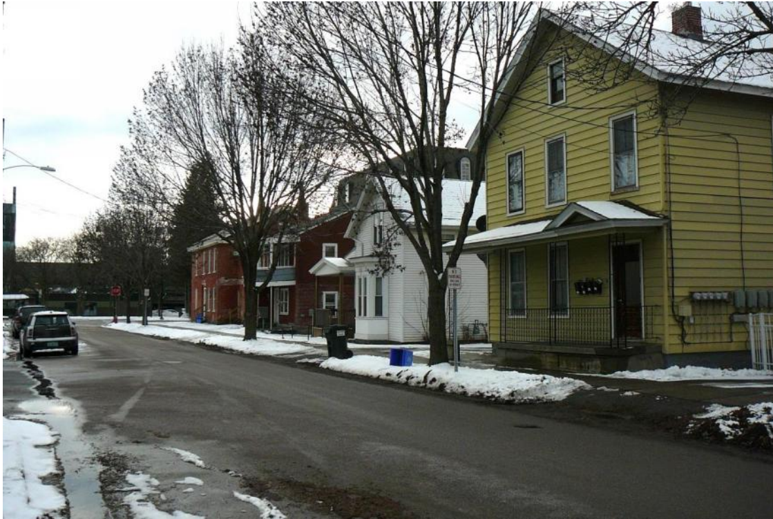
Figure 17. View southwest along George Street; (right to left) 19 George Street, 13 George Street, and 3 George Street (Stannard House).
