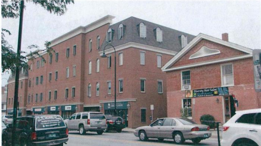
Looking northeast across Pearl Street at Victoria Place (left) and 3 George Street (right).
