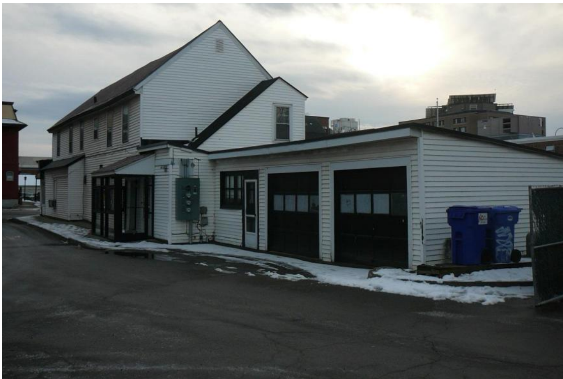
Figure 44. View southwest of east elevation 64 Pearl Street.
