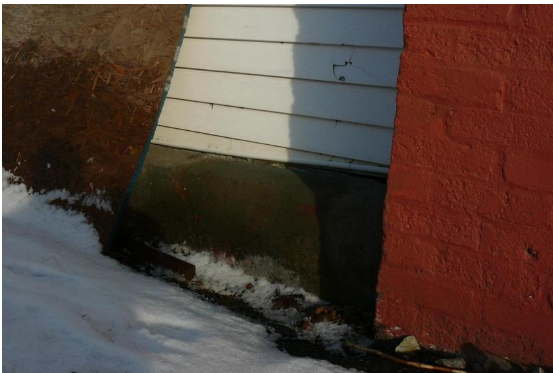
Figure 50. View of foundation under main block of 64 Pearl Street (west side of building).
