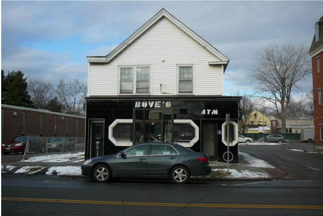
Figure 37. View north of south elevation of 64 Pearl Street.
