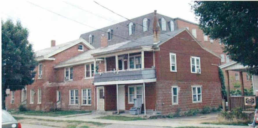
Looking southwest across George Street at 3 George Street with Victoria Place rising over the top of the roofline.
