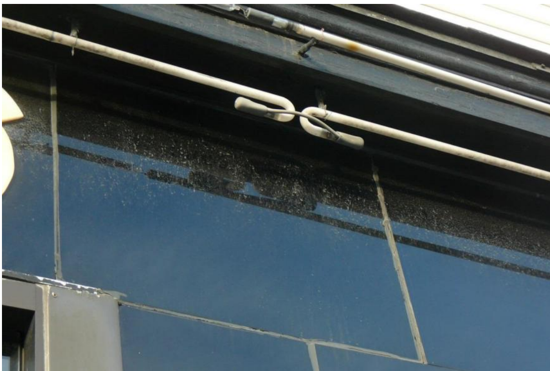
Figure 58. View of top of Carrara glass storefront and neon tubes of 64 Pearl Street.
