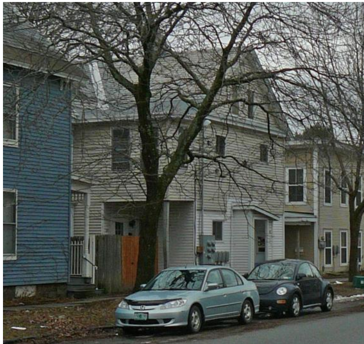
Figure 90. View southwest of 81-83 Monroe Street (center).
