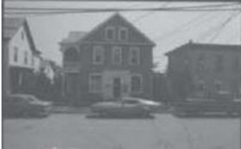
Figure 89. View south of 81-83 Monroe Street in 1978 (VTDHP 1978:81 Monroe).
