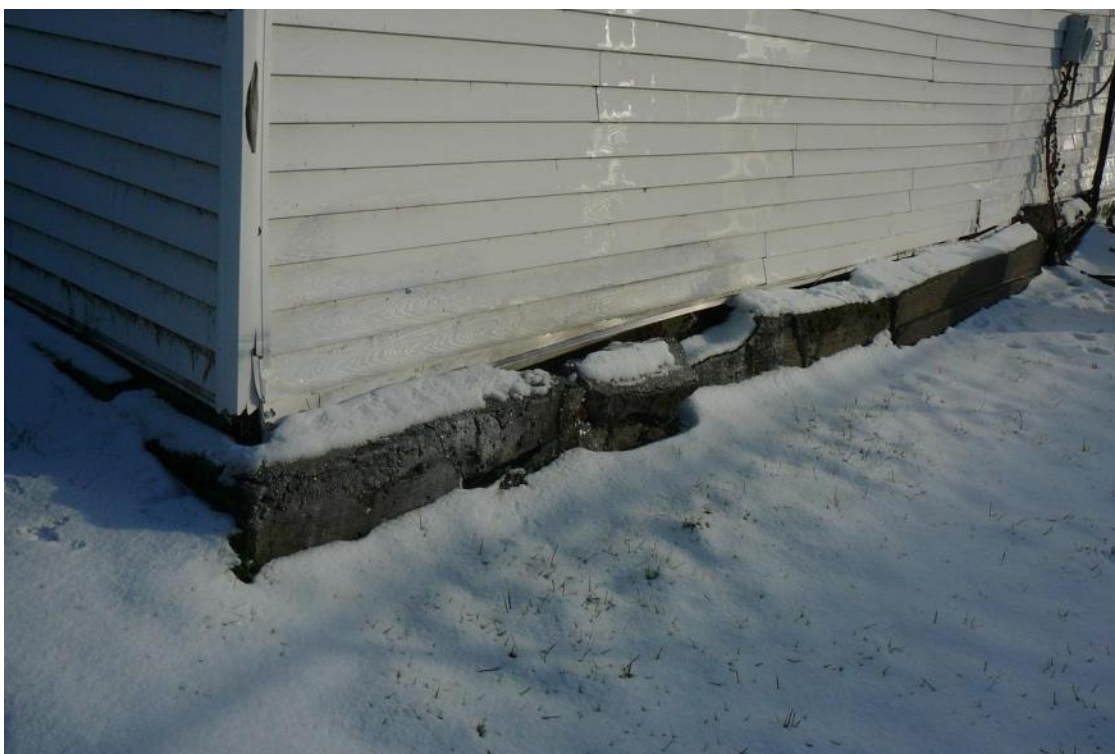
Figure 48. View of foundation under northwest corner of garage wing of 64 Pearl Street.
