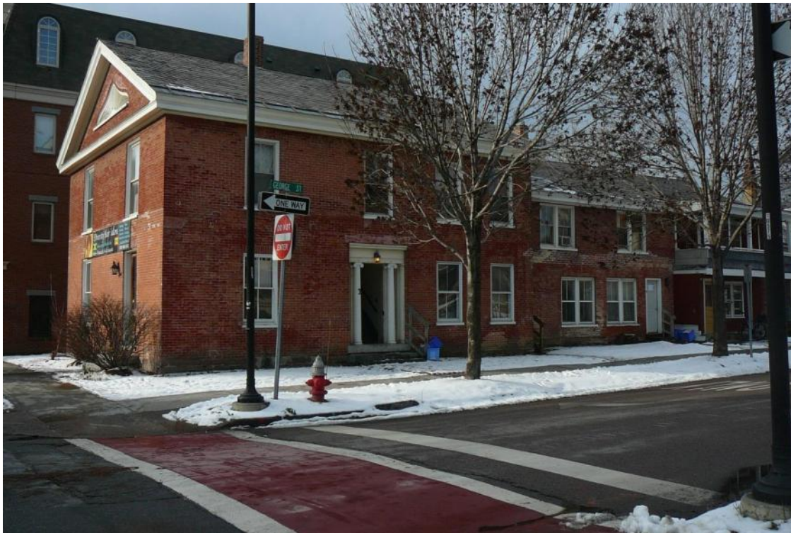
Figure 66. View northwest of east and south elevations of 3 George Street.
