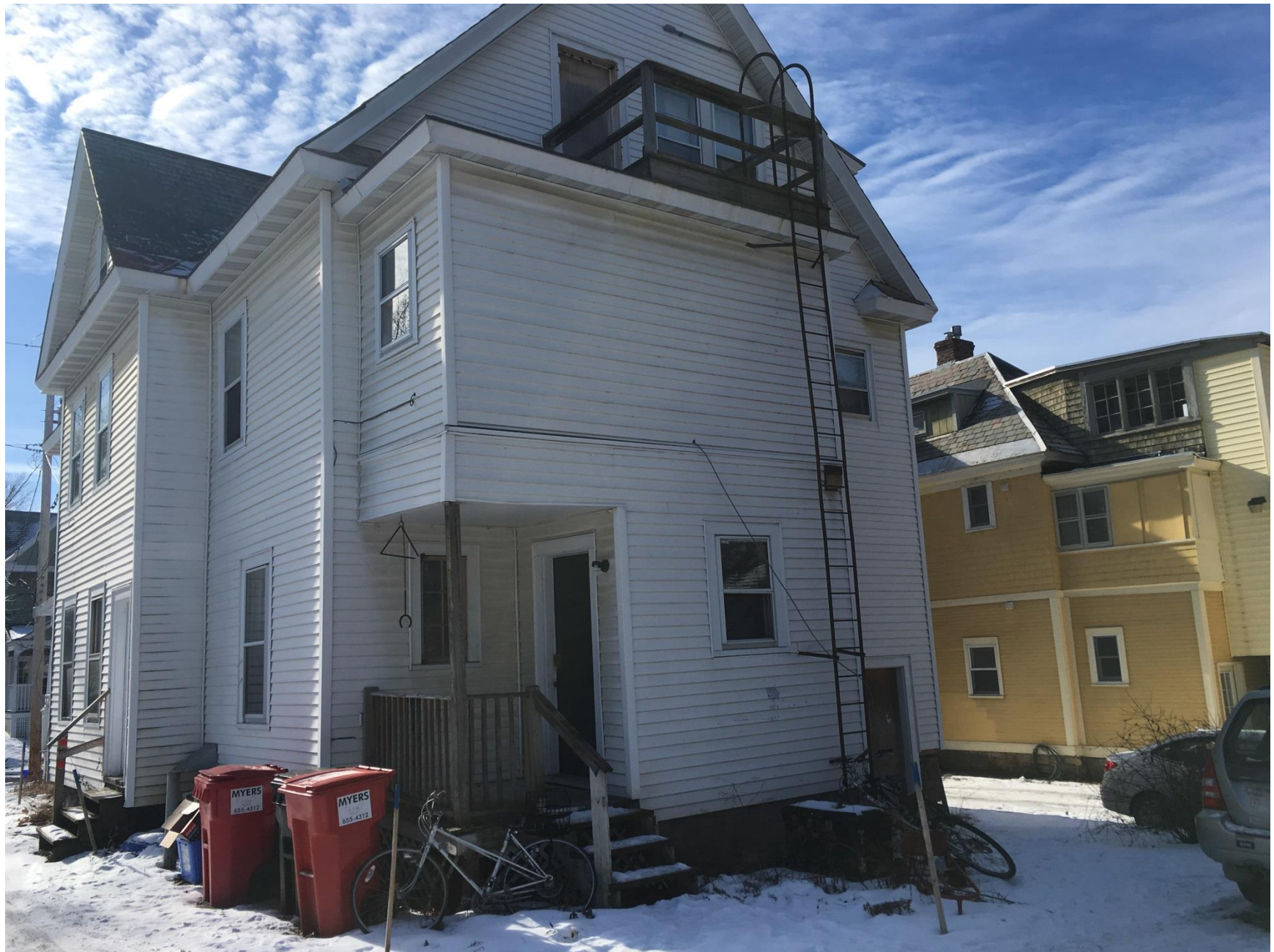
Photo depicts the view from the parking area in the North end of the property looking South toward the rental units at 32 Brookes Avenue 8
