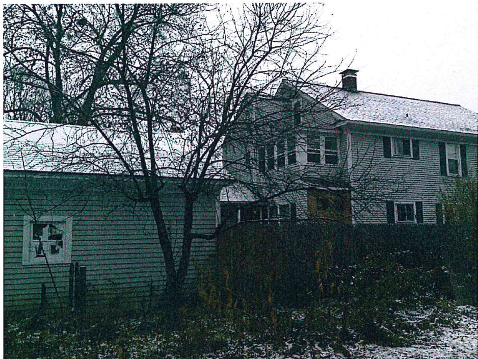
Side Yard looking East
