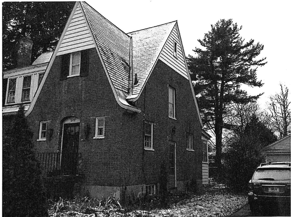
East Elevation Looking Northwest from North Street
