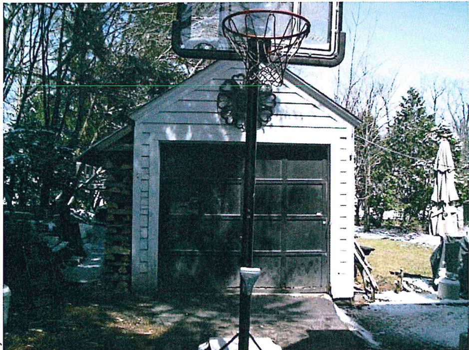
South (Front) Elevation @ Garage looking North
