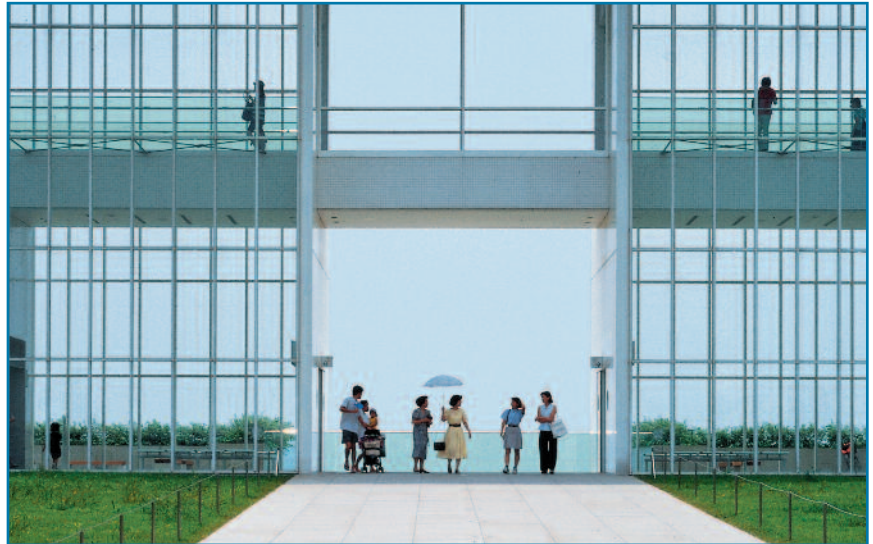
Tokyo Kasai Rinkai Park View Visitors Center
