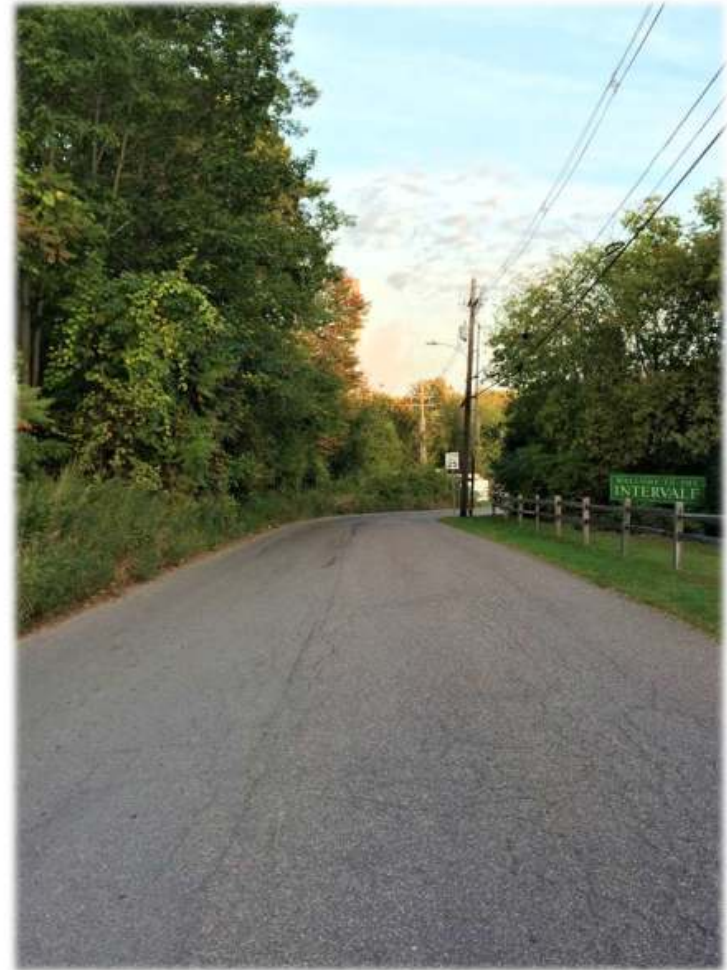
Figure 3: Intervale Road (Looking North from Railroad Tracks)
