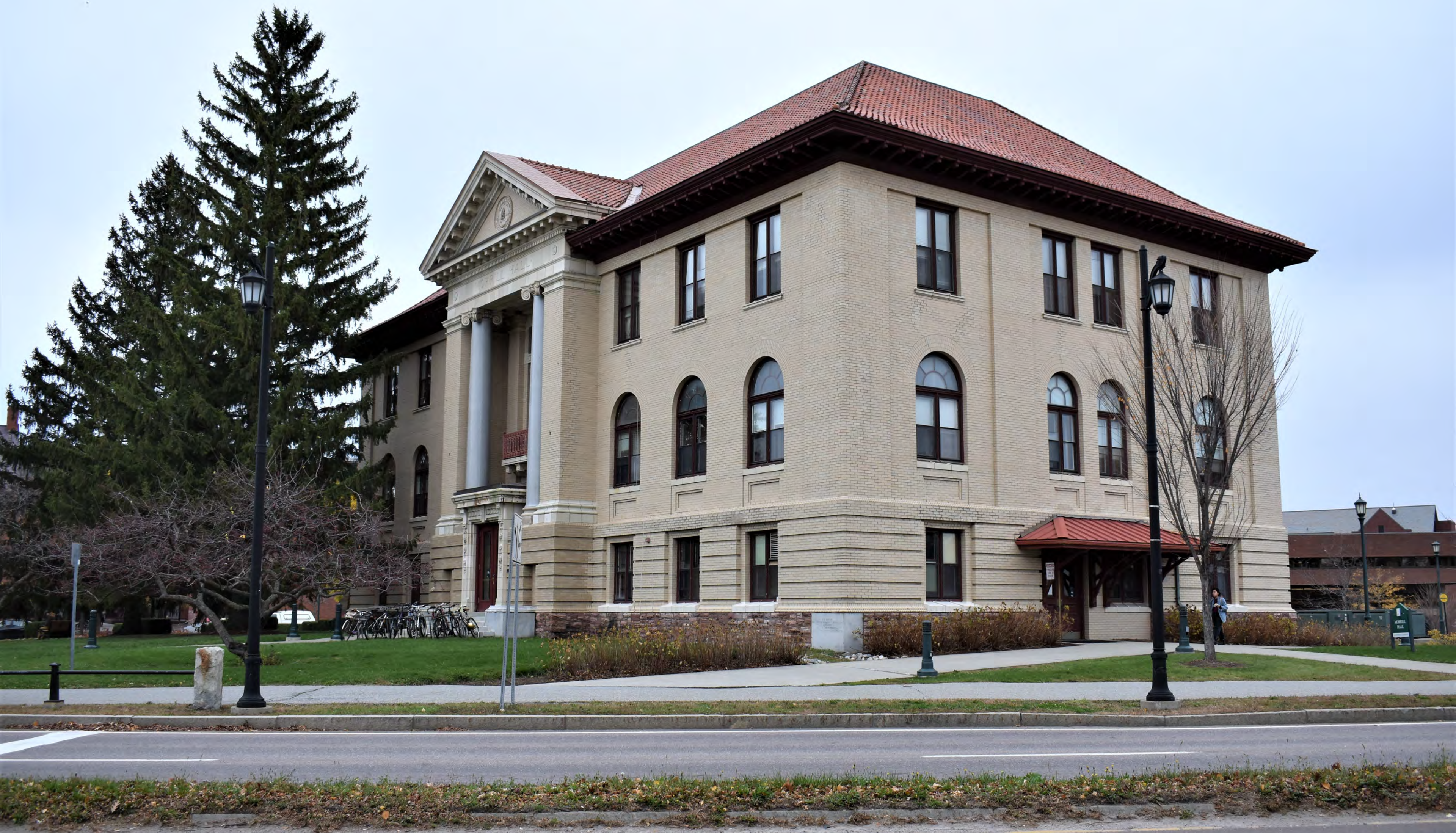
021: Morrill Hall (#11). Looking northeast.
