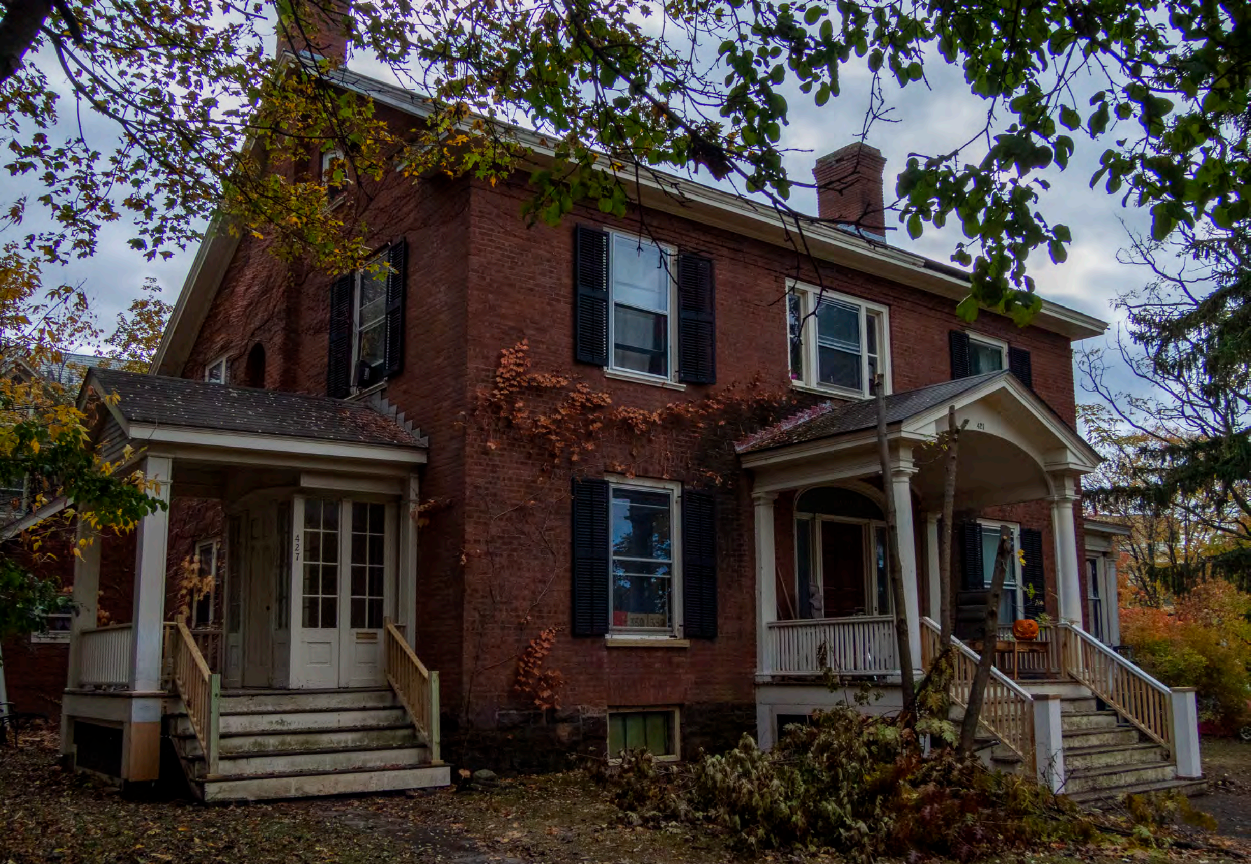
029: 421 Main Street (#20). Looking southwest.
