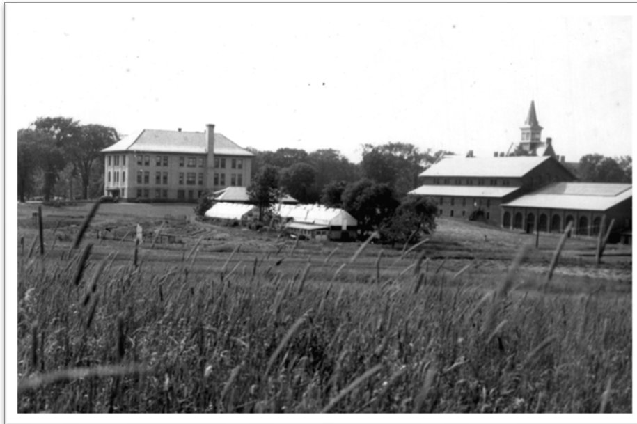
Figure 19: Undated photograph of the rear of Morrill Hall showing the former agricultural complex at the rear of the building. The Royall Tyler Theatre and Central Utility Plant (#9) is at right. UVM Landscape Change Program #LS09700.
