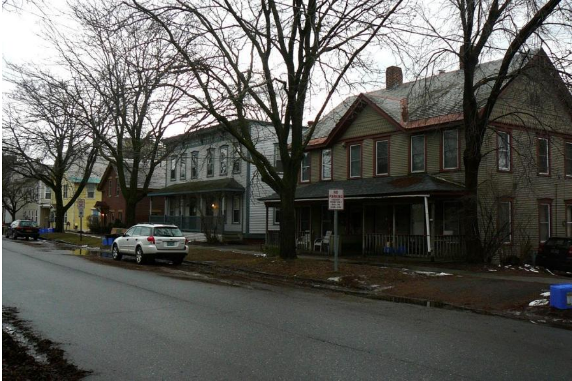
Figure 21. View southeast of buildings along the south side of Monroe Street (right to left) 61-63, 67, 69, 73-75, 77-79 Monroe Street.
