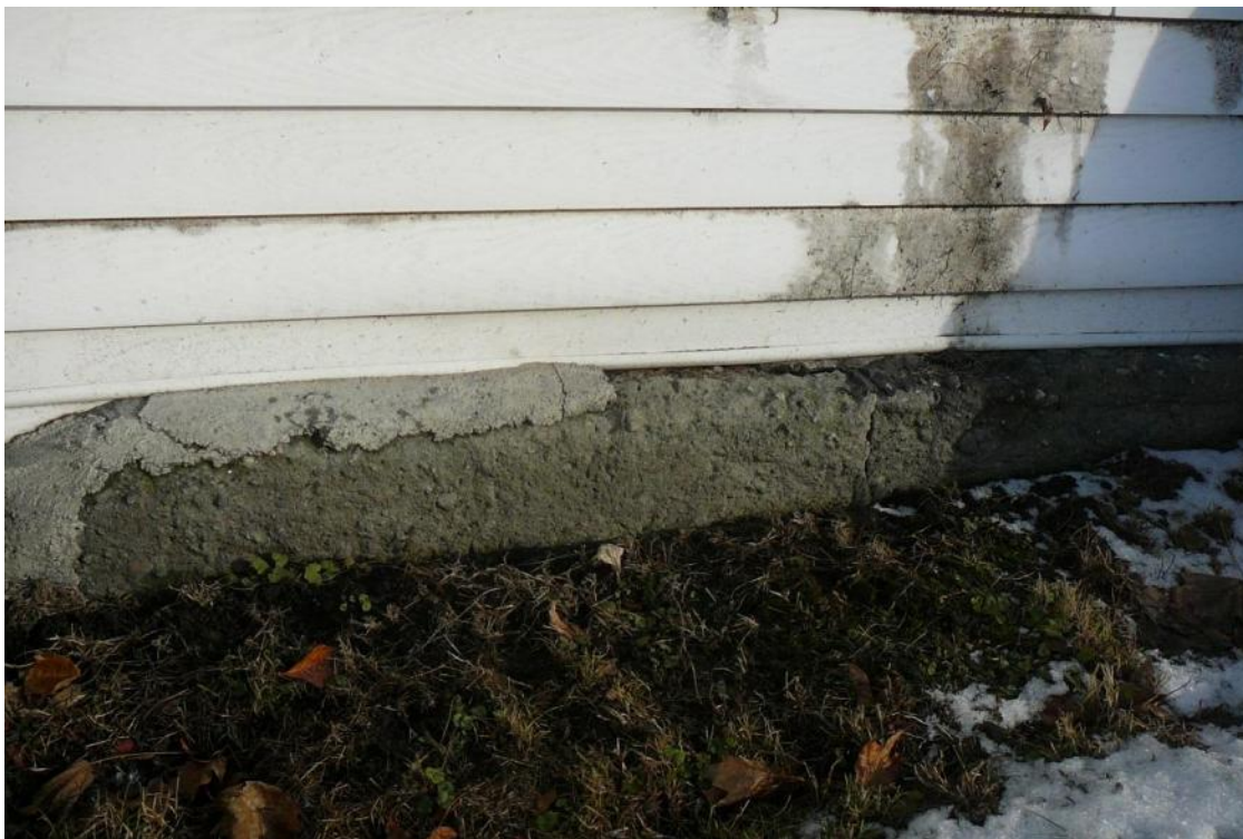
Figure 49. View of foundation under main block of 64 Pearl Street (west side of building).
