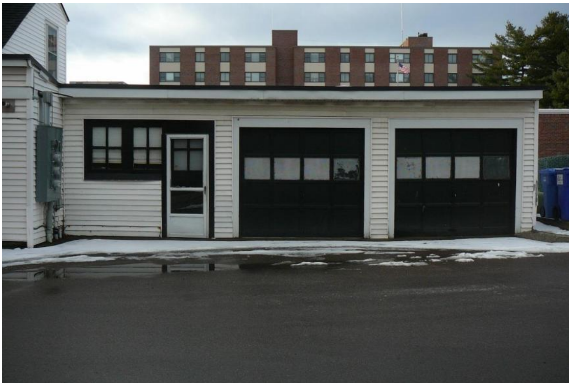
Figure 47. View west of east elevation of garage wing at 64 Pearl Street.
