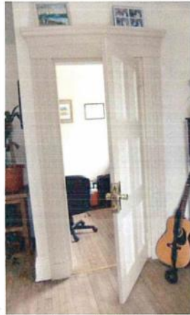
Second floor trim includes peaked window and door lintels and wide molded trim.
