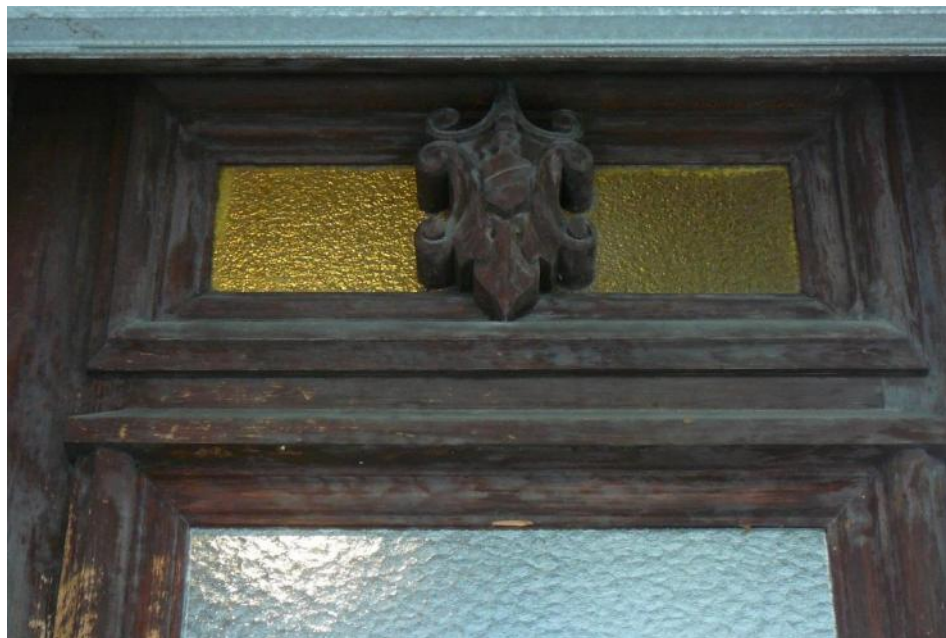
Figure 81. View of detail at top of main entry door under porch on east elevation of 19 George Street.
