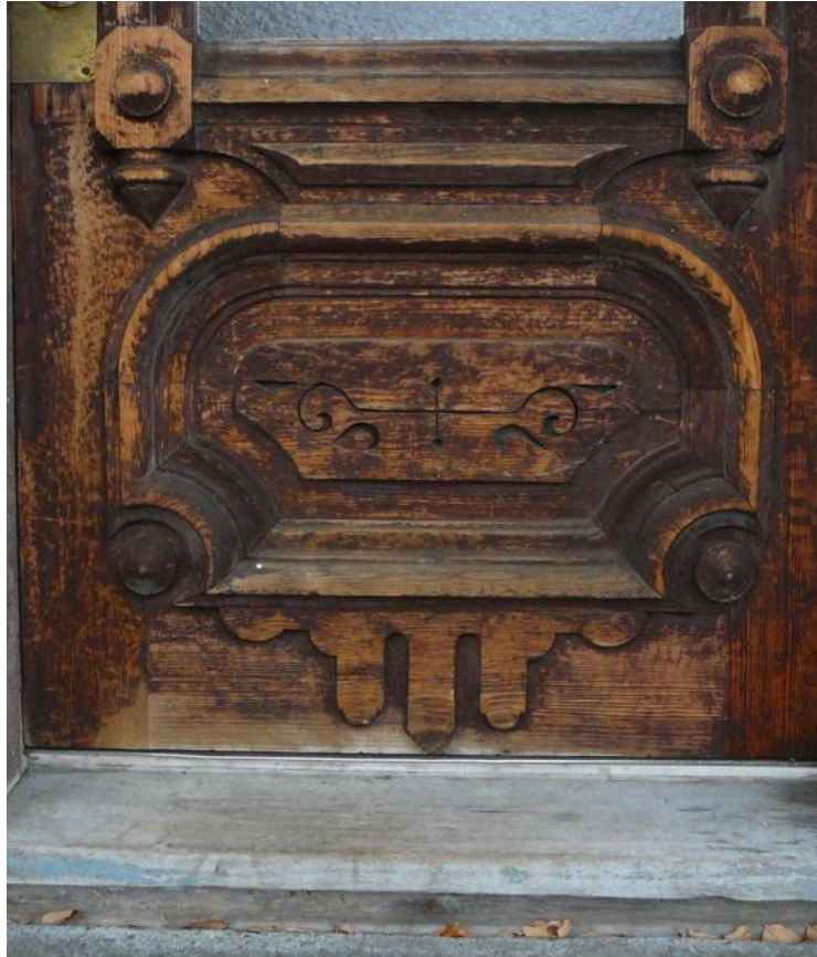
Figure 80. View of detail at bottom of main entry door under porch on east elevation of 19 George Street.
