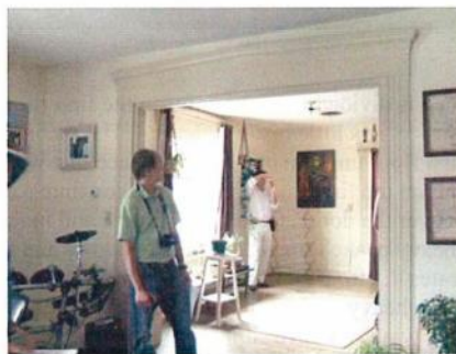
Wide opening between rooms on south end of second floor- peaked lintel and wide molded trim.
