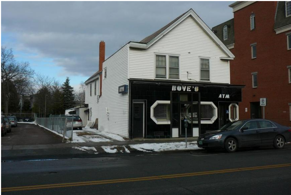
Figure 39. View northeast of south and west elevations of 64 Pearl Street.
