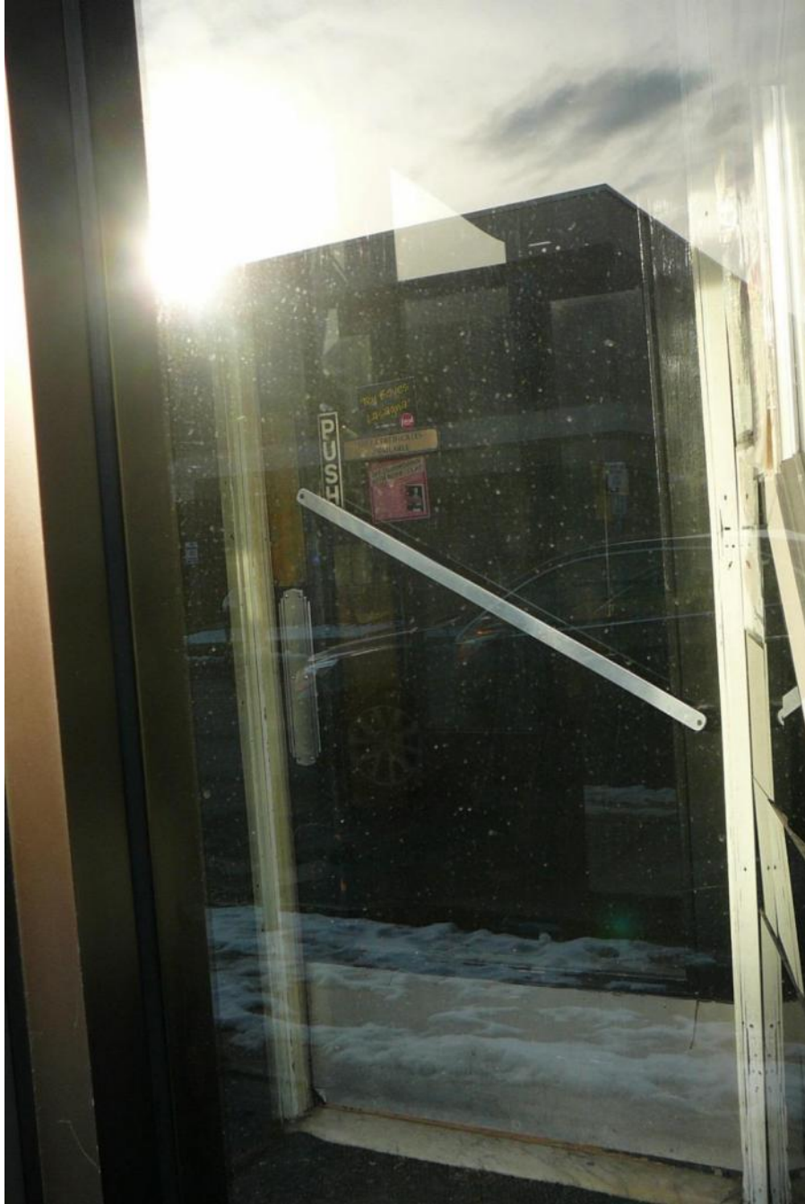
Figure 61. View of main (central) entry door within glass enclosure at 64 Pearl Street.
