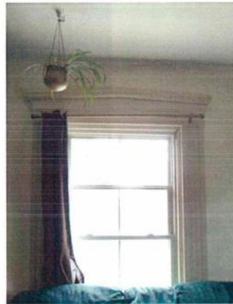
Second floor trim includes peaked window and door lintels and wide molded trim.
