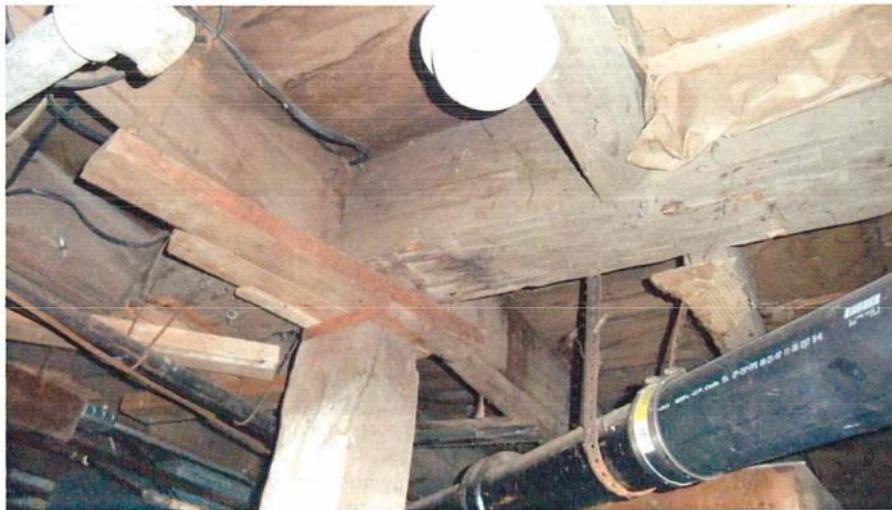
Repairs to first floor framing in basement.
