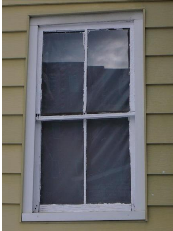
Figure 83. View of typical 2/2 window on westernmost shed wing of 19 George Street.
