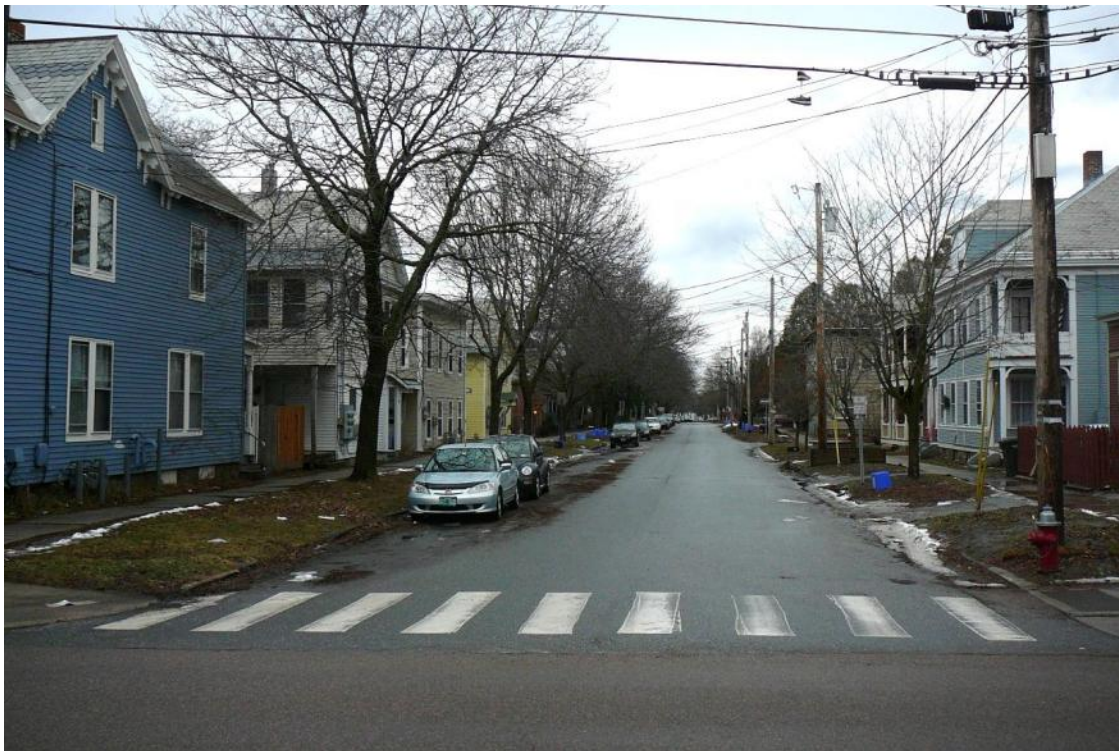
Figure 18. View west of buildings along Monroe Street; (right, foreground to background) 31 George Street, 81-83, 77-79, 73-75 Monroe Street.
