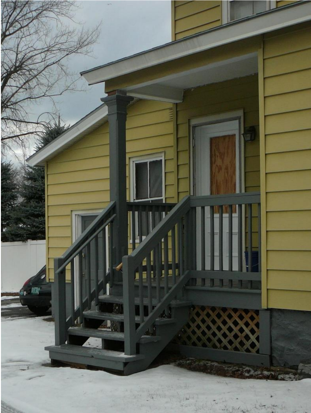
Figure 77. View northwest of porch on south elevation of wing of 19 George Street.
