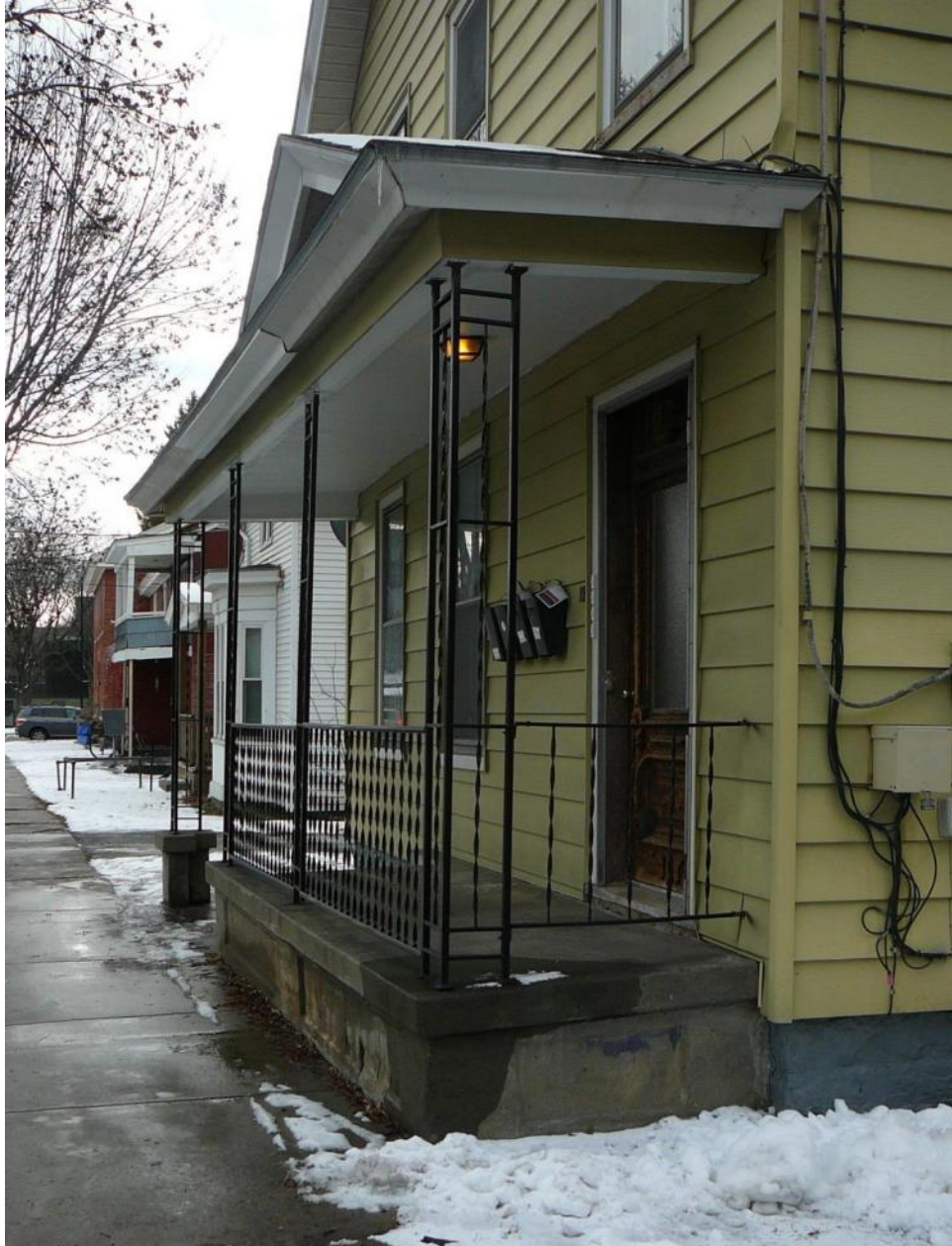
Figure 76. View southwest of porch on east elevation of 19 George Street.
