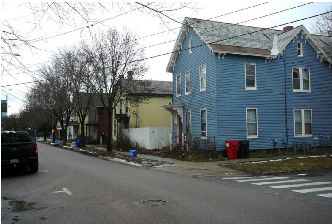
Figure 16. View southwest along George Street; (right to left) 31, 27, 23 and 19 George Street.
