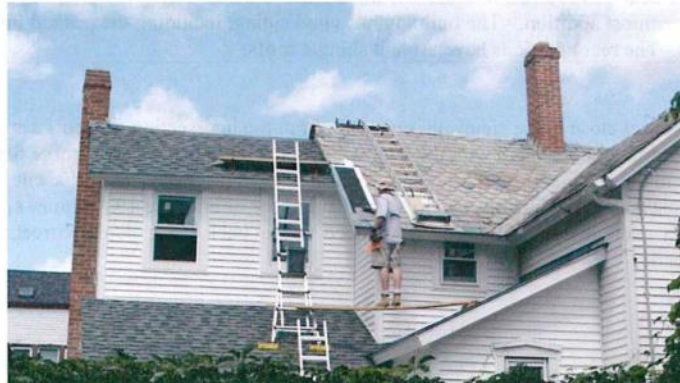
Looking north at rear additions and slate roof of main block.
