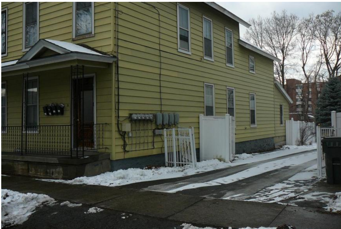
Figure 73. View southwest of north elevation of 19 George Street.
