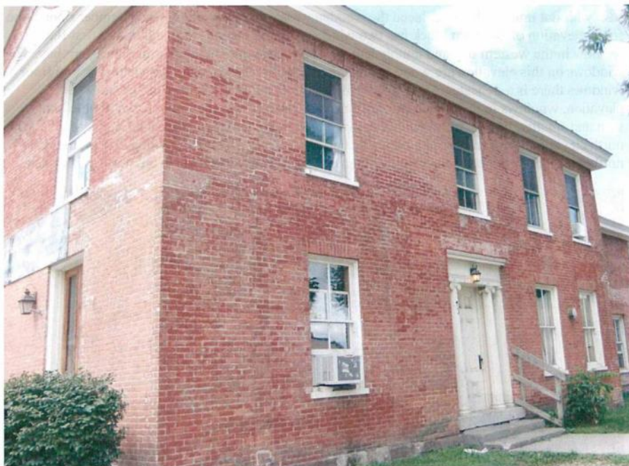
Front (east) elevation of main block with molded cornice, jack arches, replacement windows on second floor, variety of bricks and mortar- some bricks with remnant paint, redstone foundation, ghosts of former additions.
