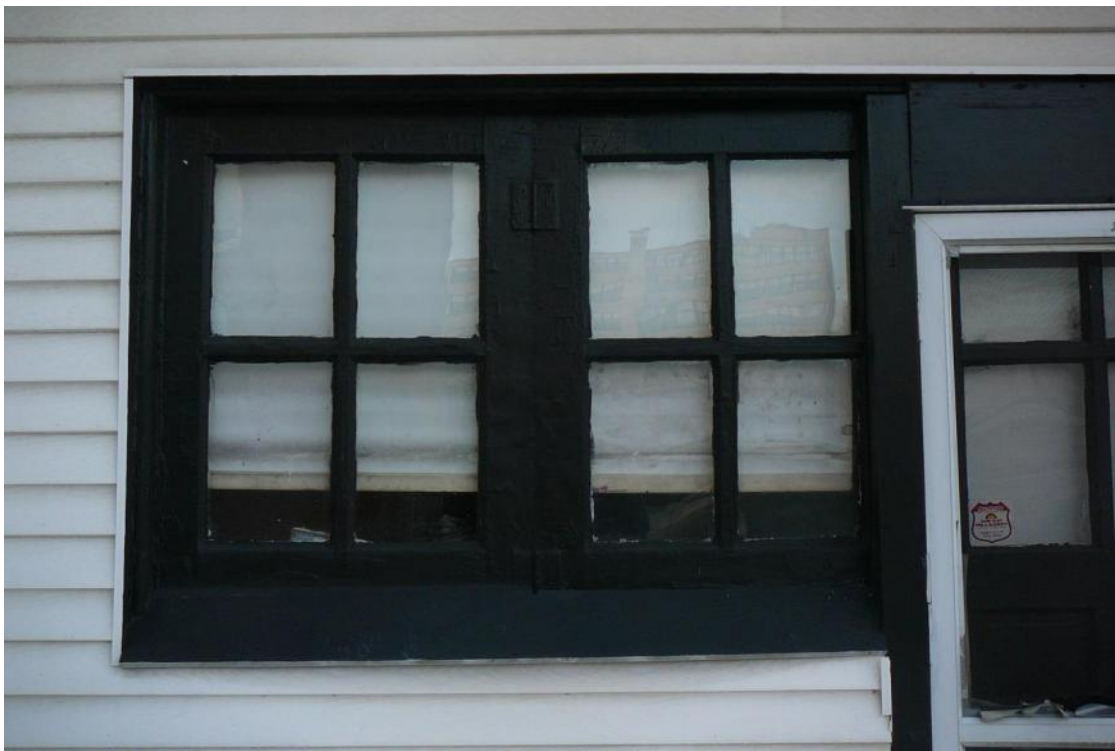
Figure 53. View of windows on garage wing of 64 Pearl Street.
