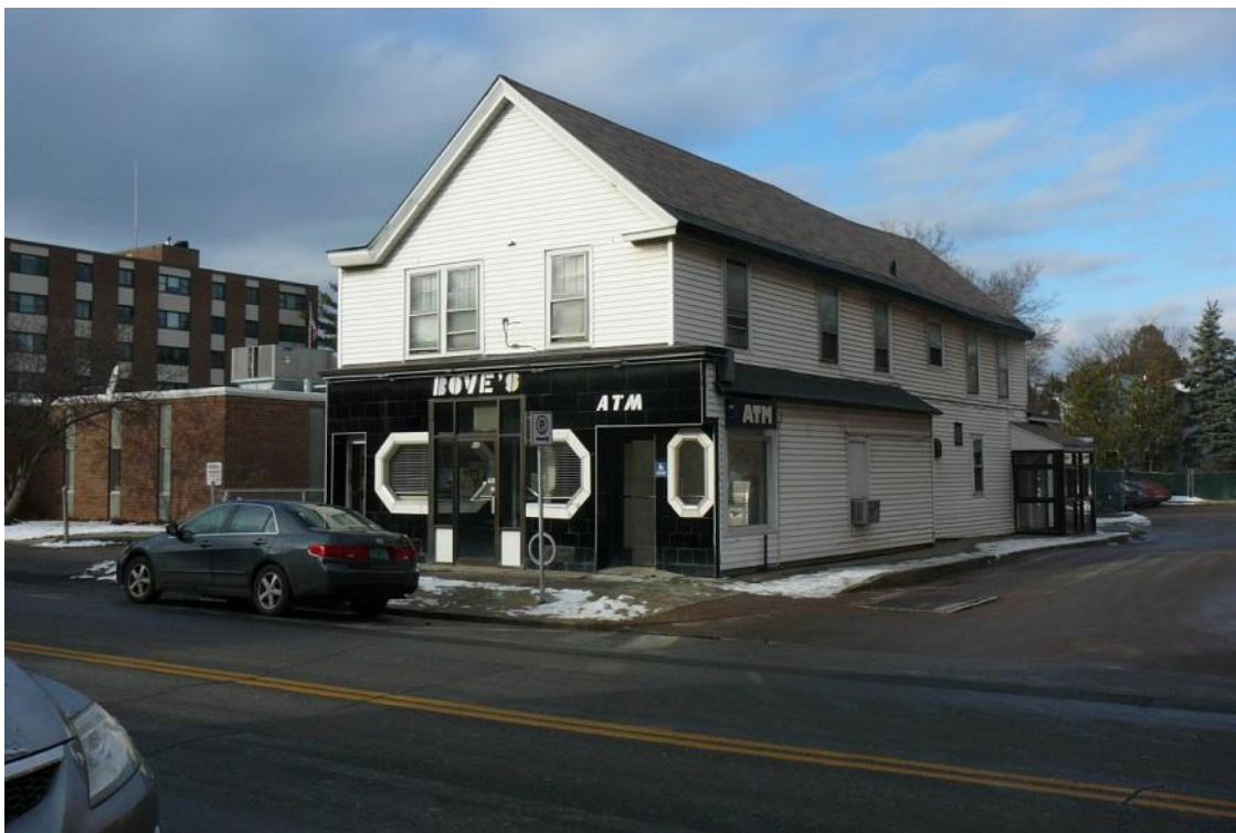
Figure 38. View northwest of south and east elevations of 64 Pearl Street.
