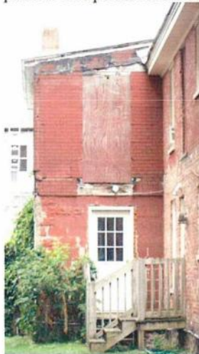
Looking north at south end of addition
