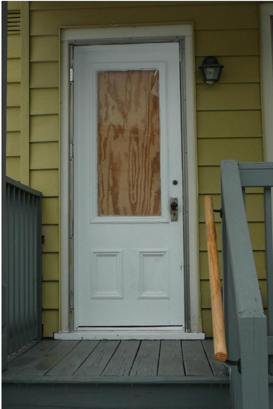
Figure 82. View of door under porch on south elevation of wing of 19 George Street.
