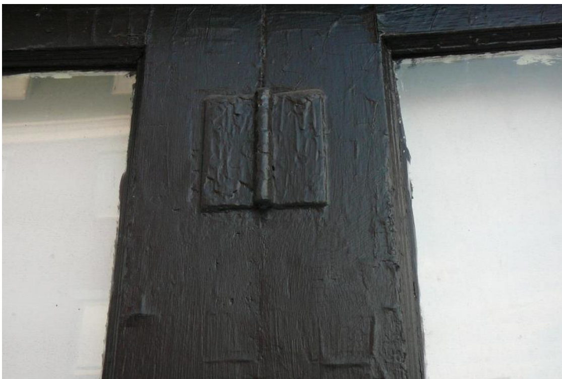
Figure 54. View of hinge between windows on garage wing of 64 Pearl Street.
