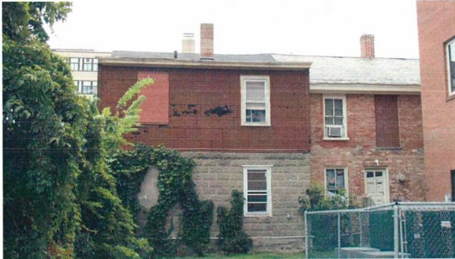
Looking east from parking lot behind Victoria Place at rear wall of cinder block addition and rear wall of wing.
