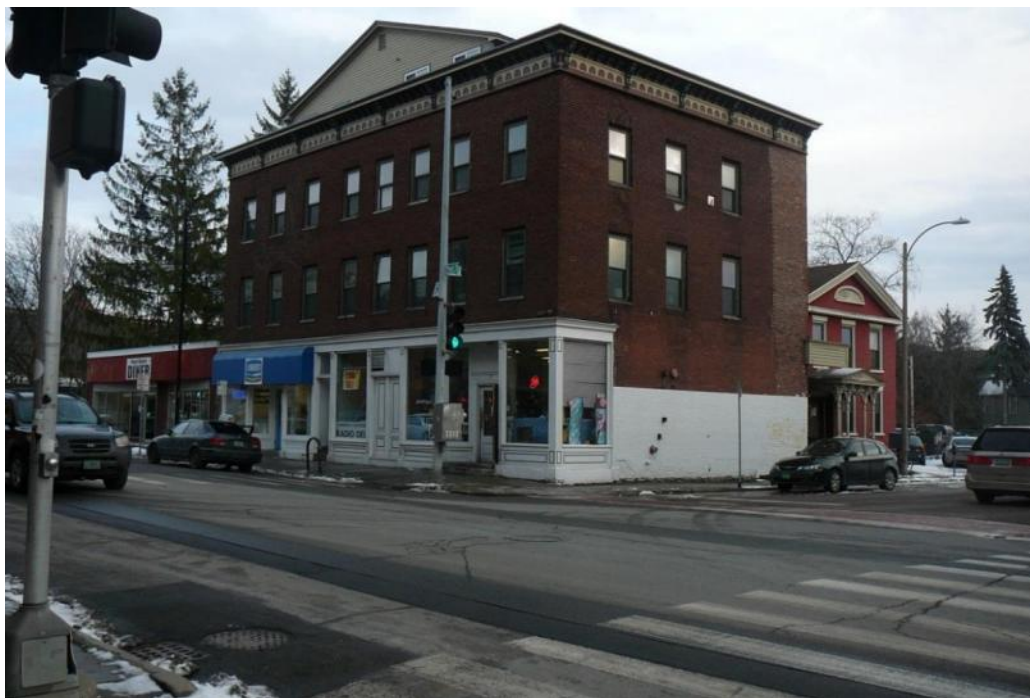
Figure 87. View southeast of 77 Pearl Street.
