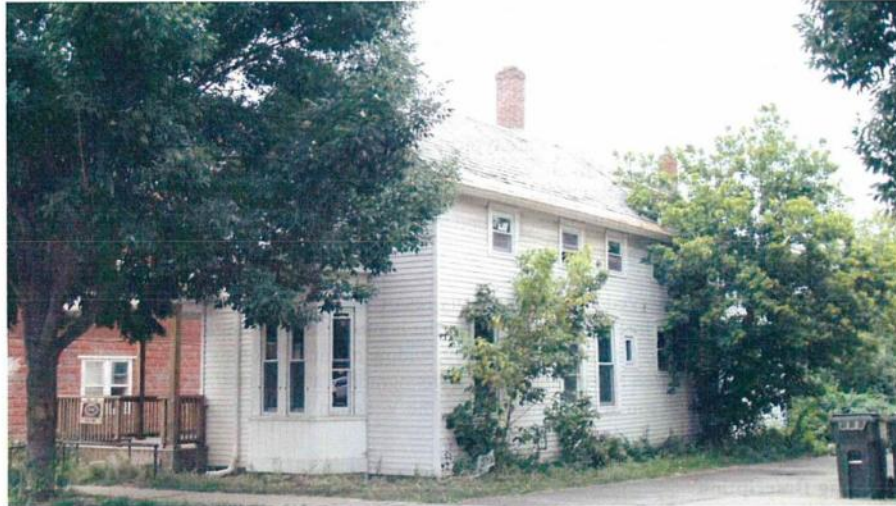
Looking west at front (east) and north sides, with vinyl windows and attic windows at eaves.
