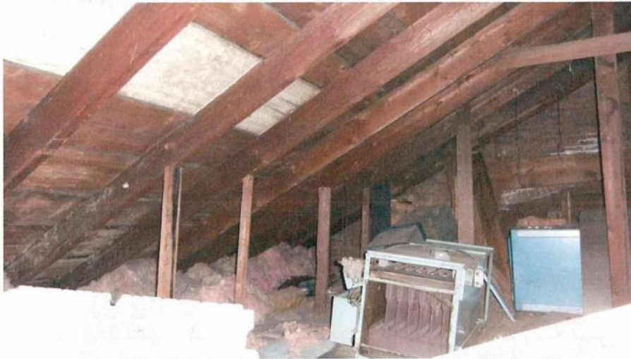
Attic of main block showing roof rafters and brick at gable end on far right.
