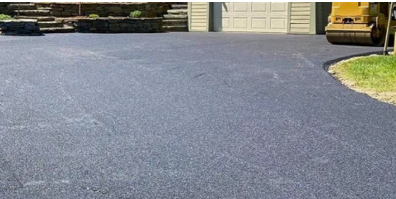
I. Porous Asphalt Vendor: S.T. Paving
