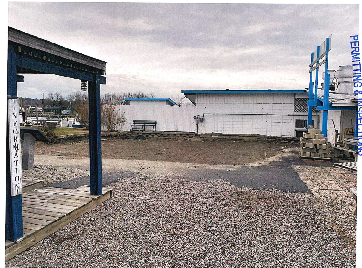
PHOTO 4: VIEW FROM NORTH LOOKING SOUTH TOWARDS EXISTING BUILDING & WHERE NEW BATHROOM PAVILION TO BE BUILT
