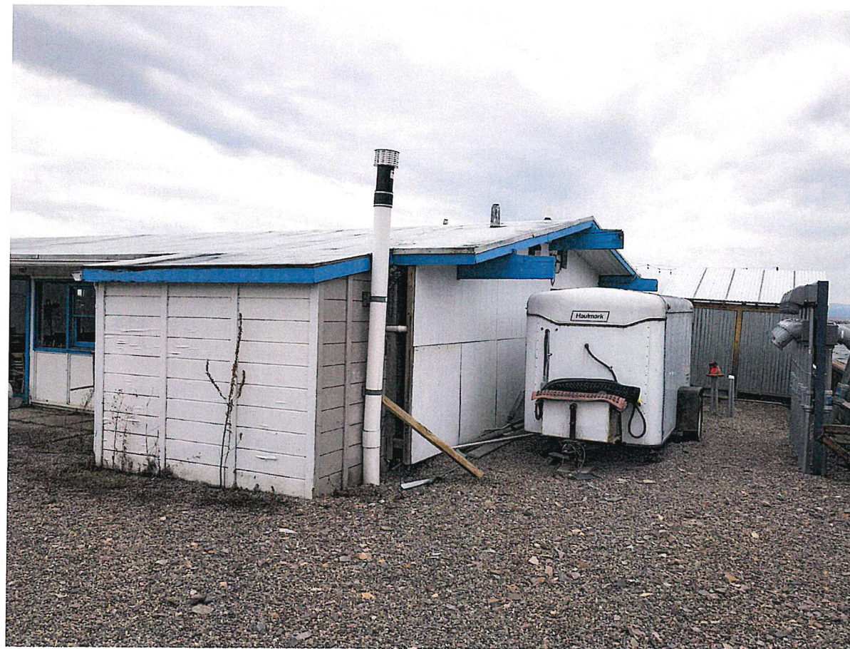
PHOTO 3: VIEW FROM NORTHEAST LOOKING SOUTHWEST TOWARDS EXISTING BATHROOMS TO BE DEMOLISHED & REPLACED W/ BAR EXTENSION
