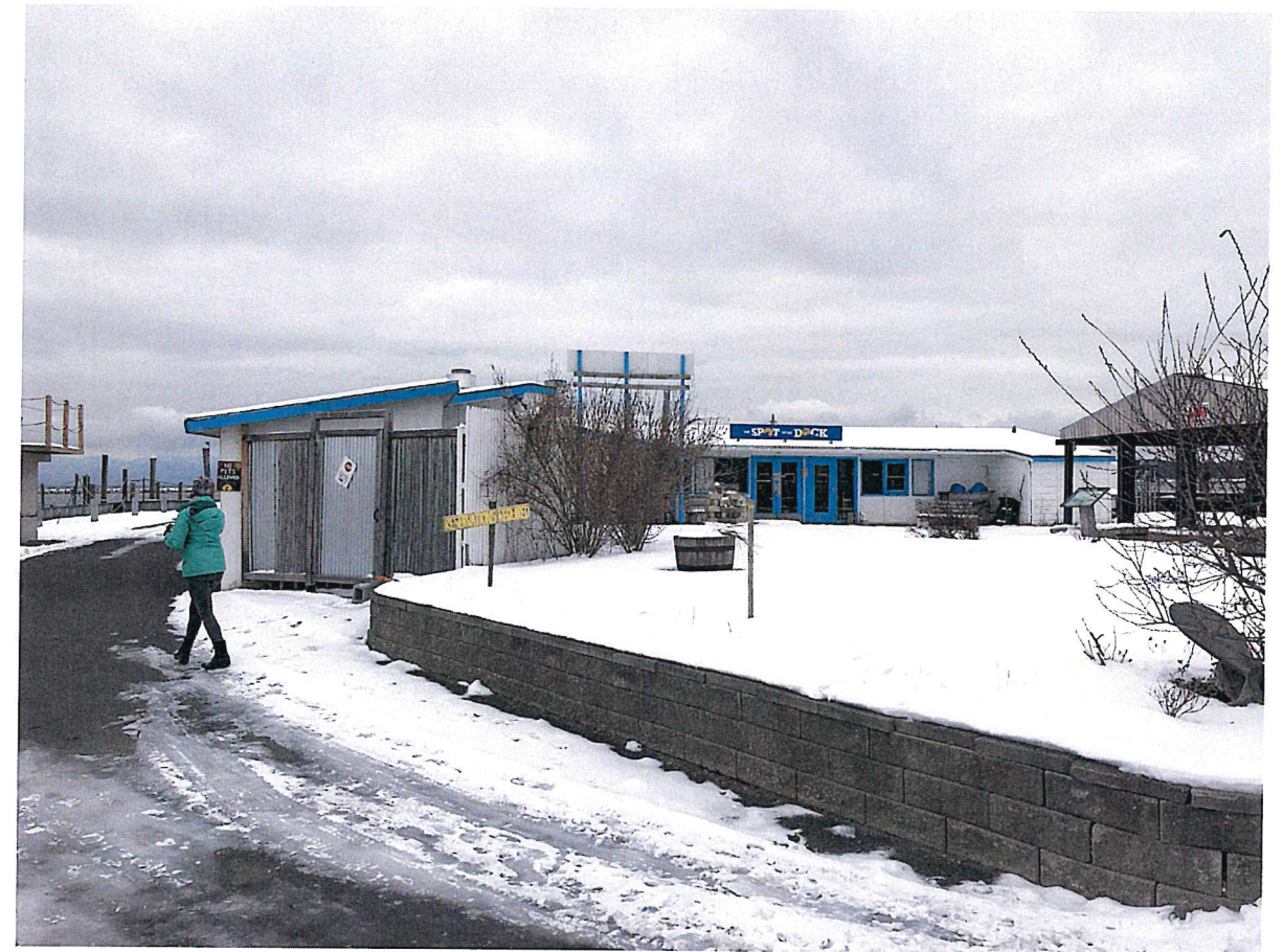
PHOTO 2: VIEW FROM EAST LOOKING WEST TOWARDS SERVICE/STAFF ENTRY
