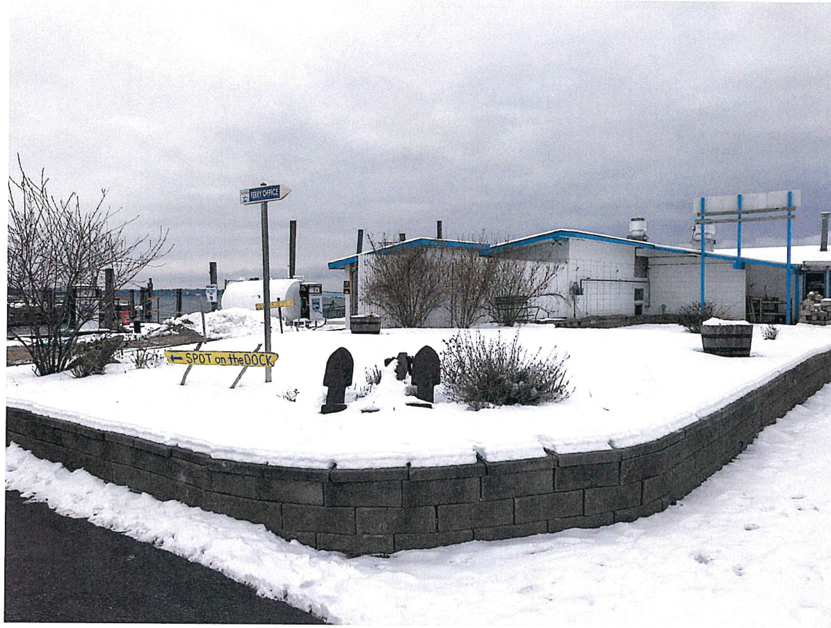
PHOTO 1: VIEW FROM EAST LOOKING SOUTHWEST TOWARDS RESTAURANT PUBLIC ENTRY
