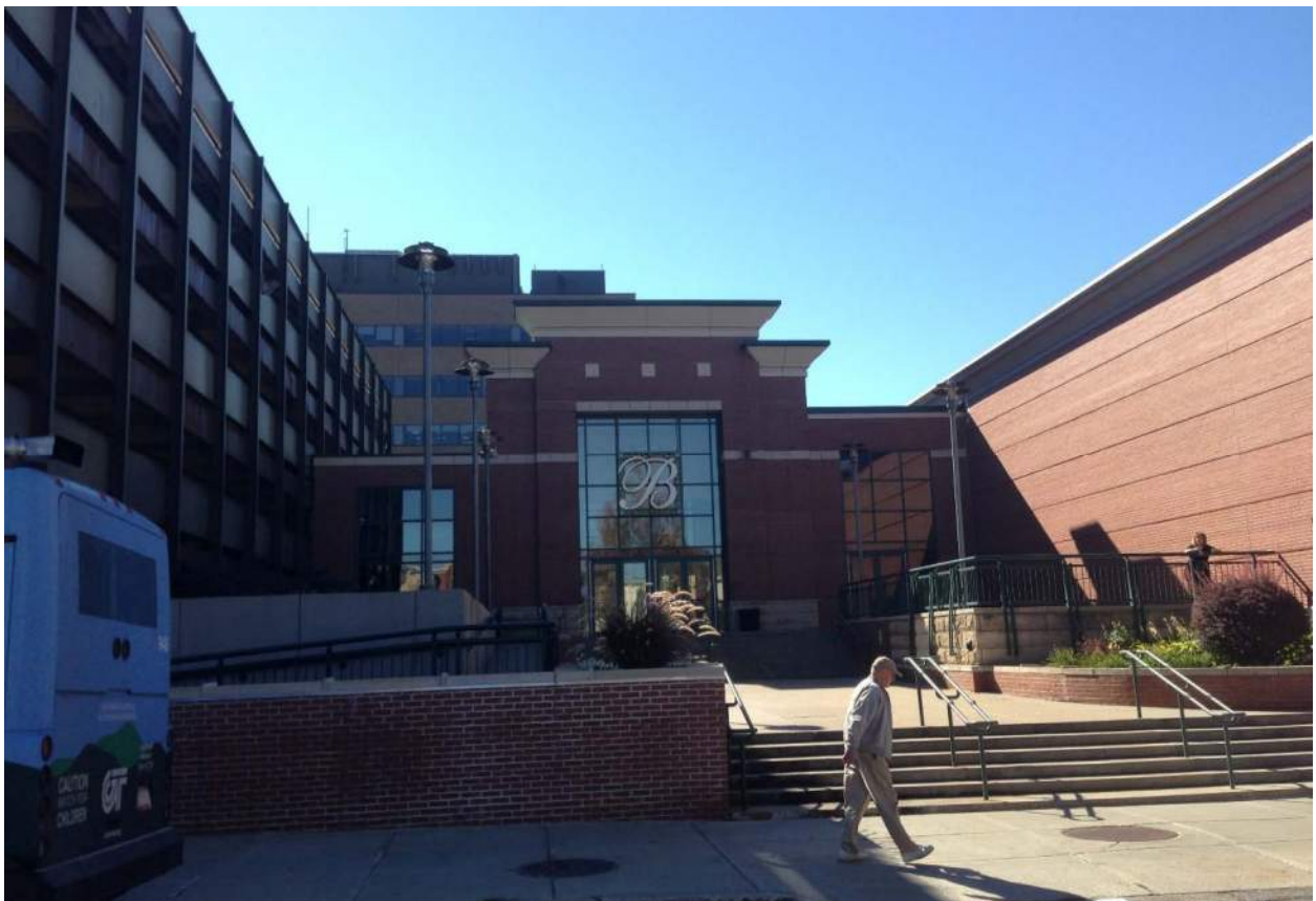
3.8 PINE STREET AT CHERRY STREET - LOOKING SOUTH
