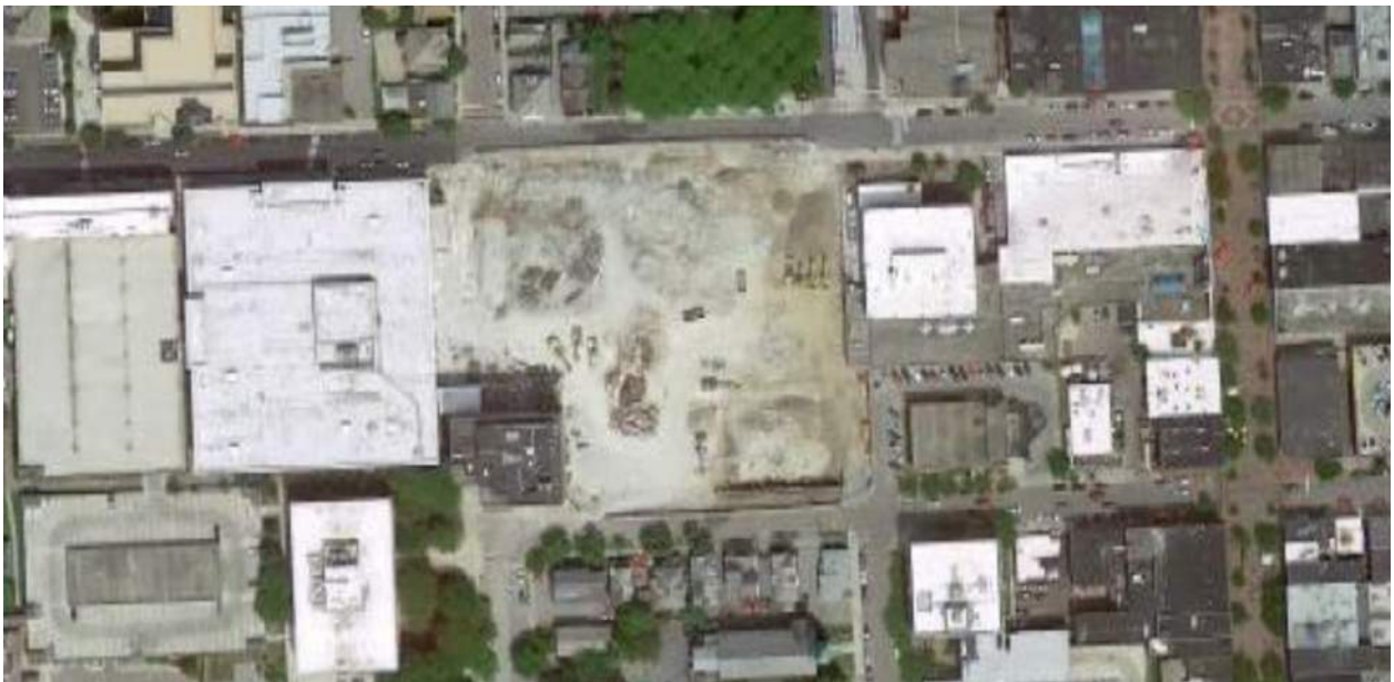
3.2- AERIAL VIEW- CURRENT CONDITION AT TIME OF AMENDED APPLICATION
