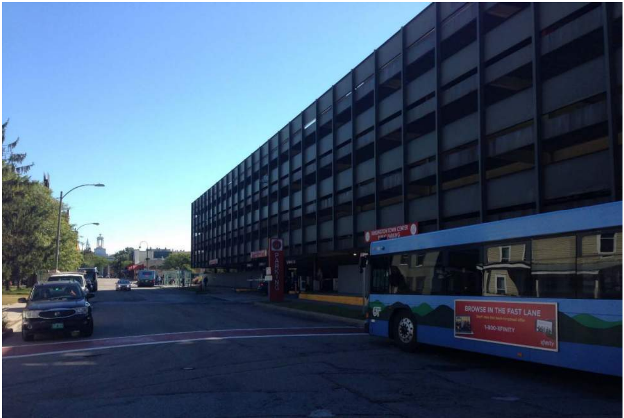
3.7 CHERRY STREET - LOOKING SOUTHEAST
