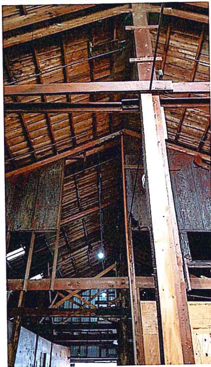
RED WAREHOUSE INTERIOR SHOWING ORIGINAL EAST SIDE SIDING
