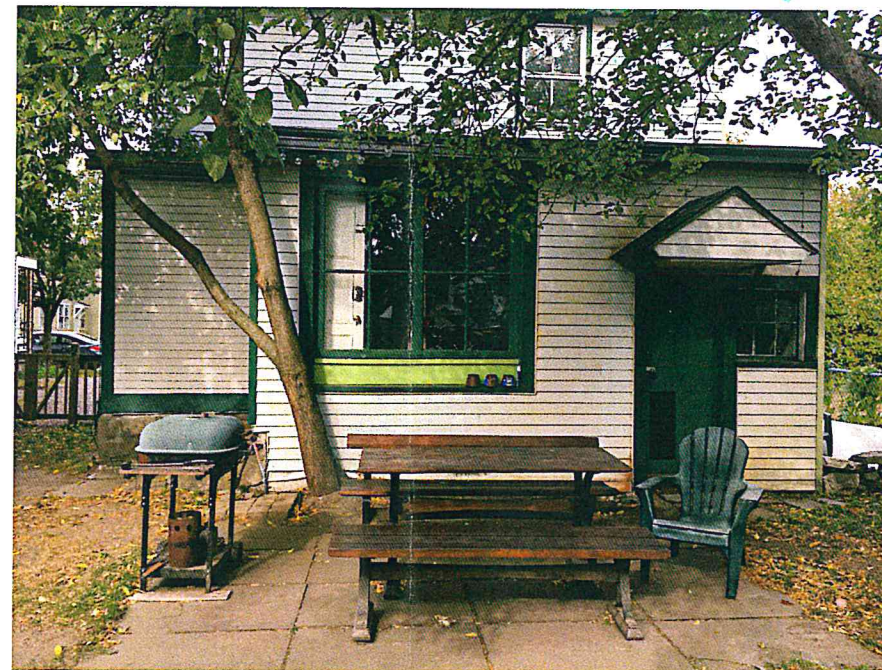
VIEW OF BUILDING FROM BACK YARD
