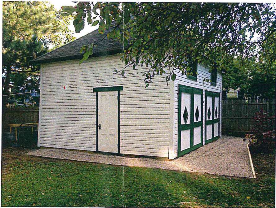
CARRIAGE HOUSE AFTER RENOVATION FROM NORTH
