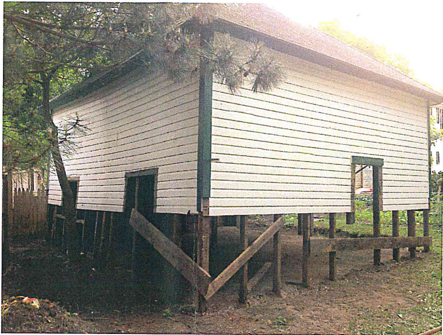
CARRIAGE HOUSE DEMO WORK
