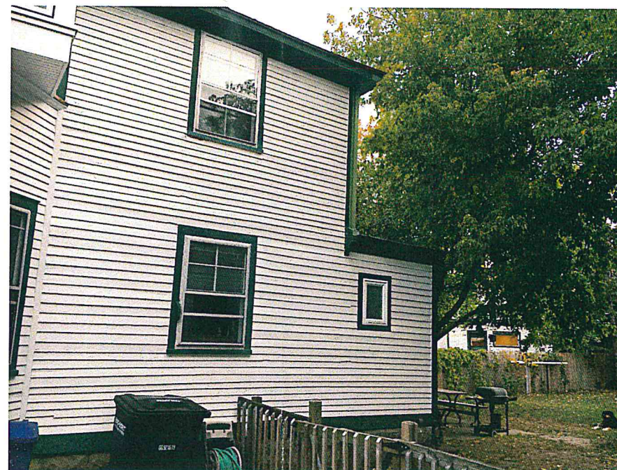
VIEW OF SOUTH WEST ELEVATION FROM DRIVE WAY
