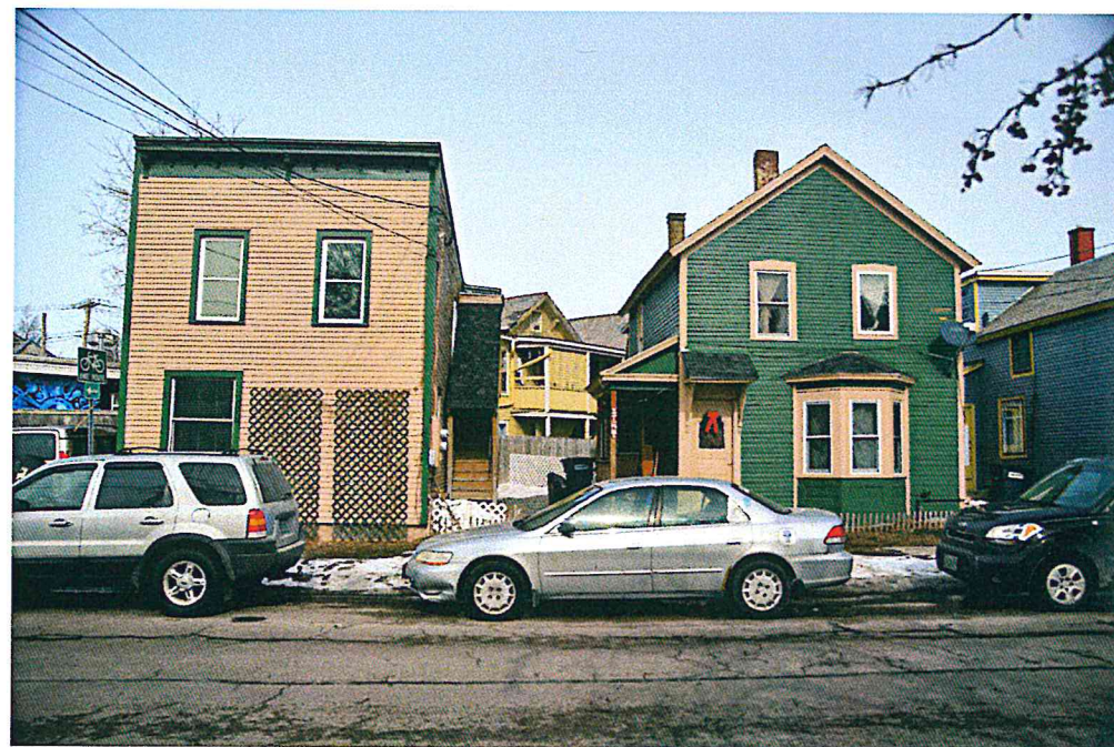
MIX OF FLAT AND GABLE ROOFS
