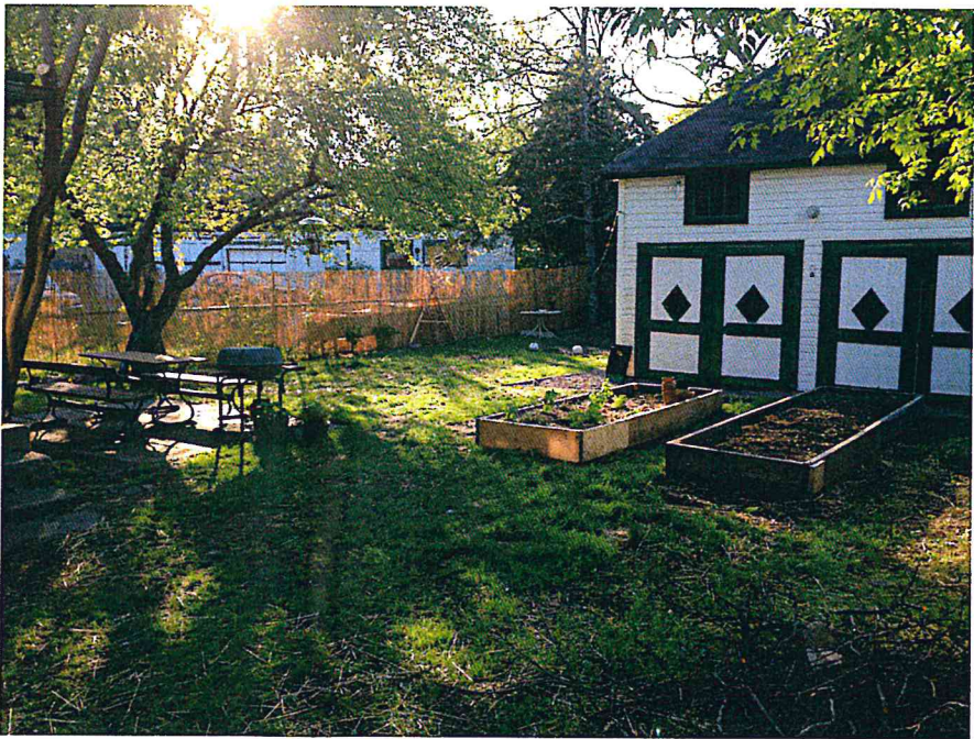
CARRIAGE HOUSE AFTER RENOVATION FROM SOUTH WEST
