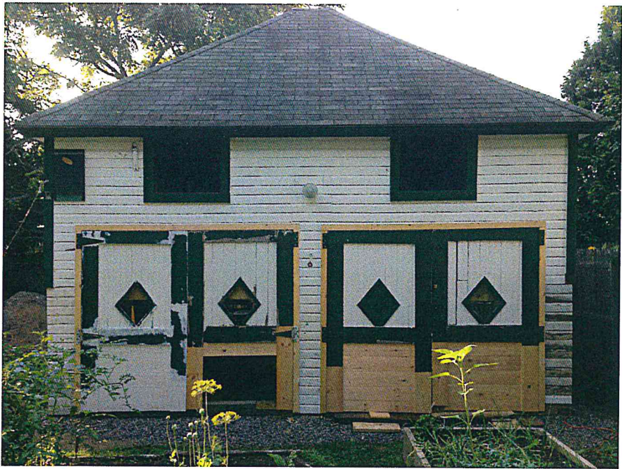
CARRIAGE HOUSE NEW DOORS, TRIM AND SIDING
