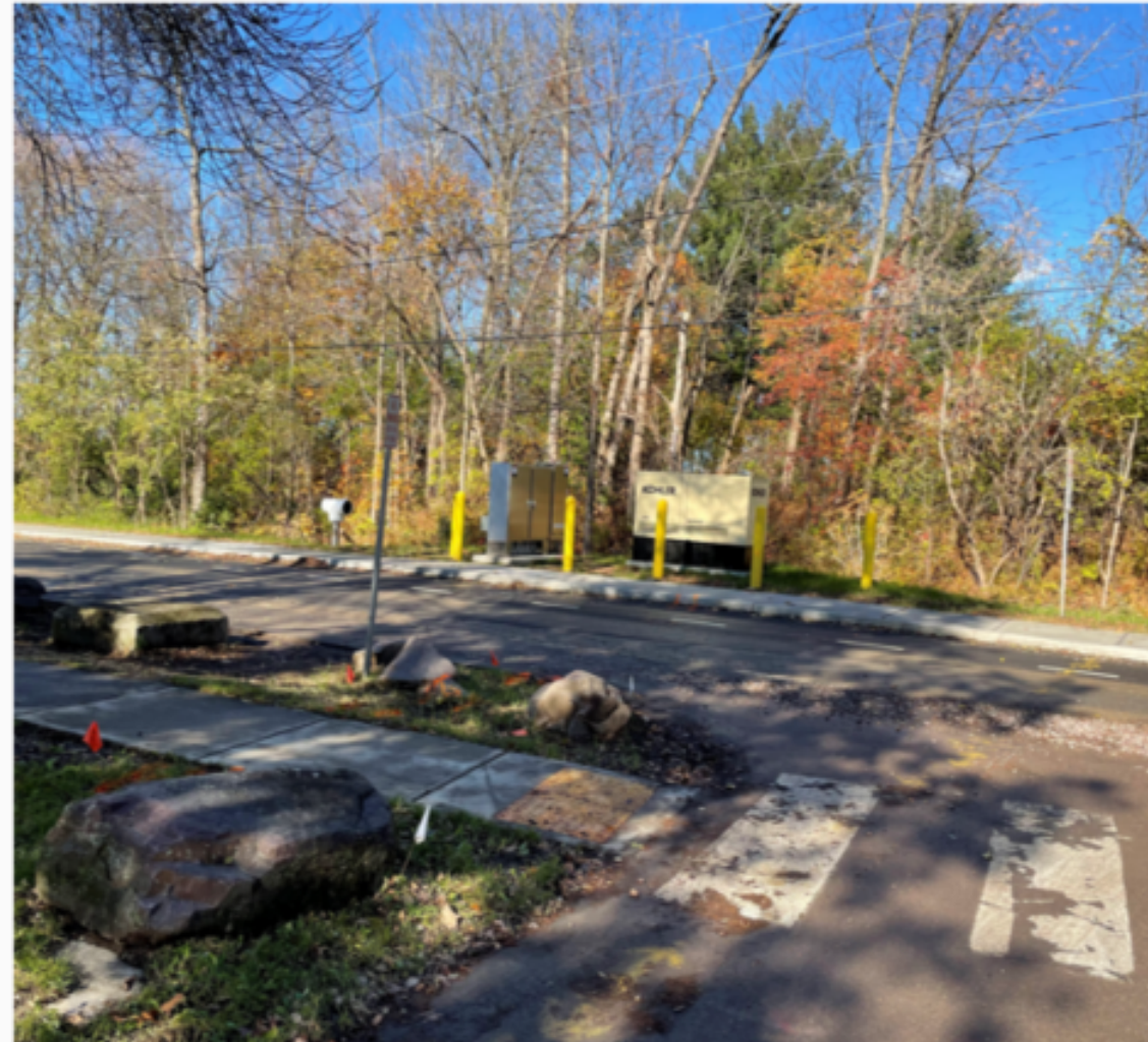
Flynn Ave Pump Station
