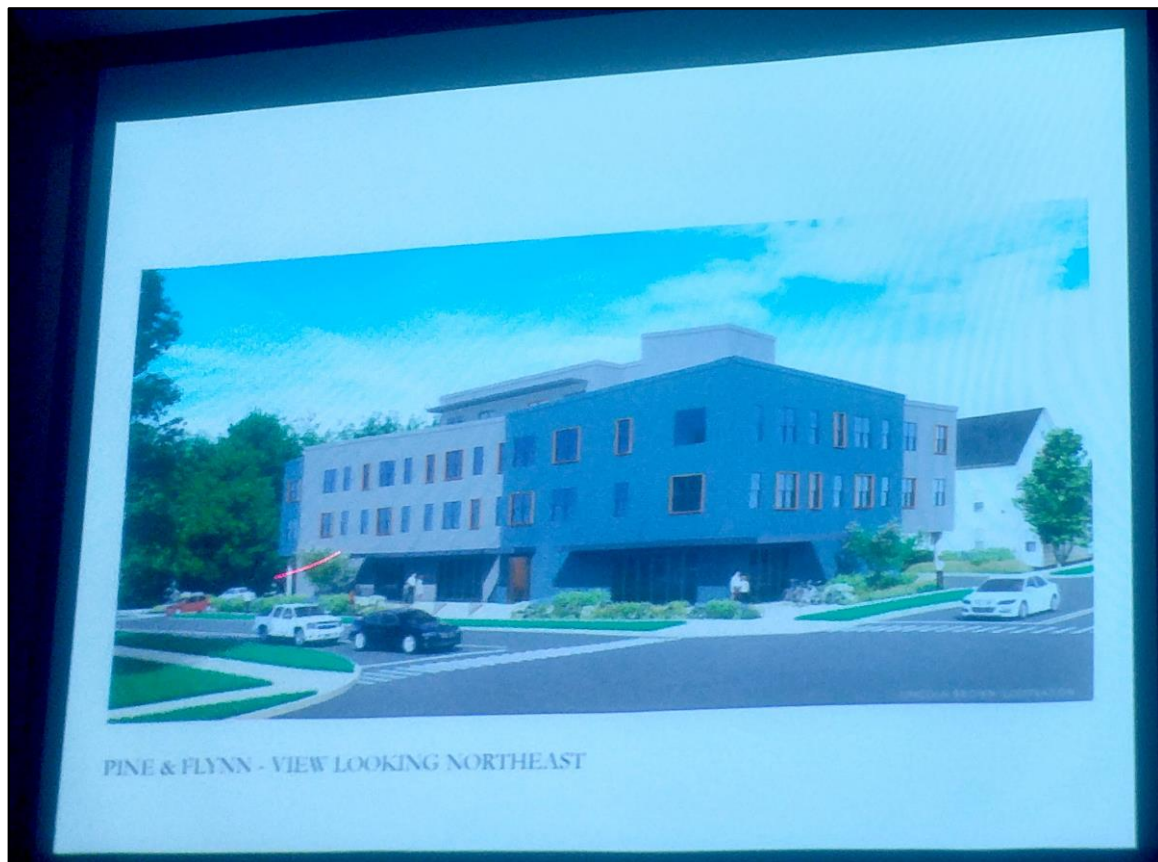
Pine Street Deli redevelopment – Pine & Flynn – View looking northeast
