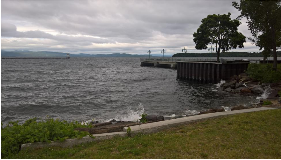
DOCK ACCESS POINT
