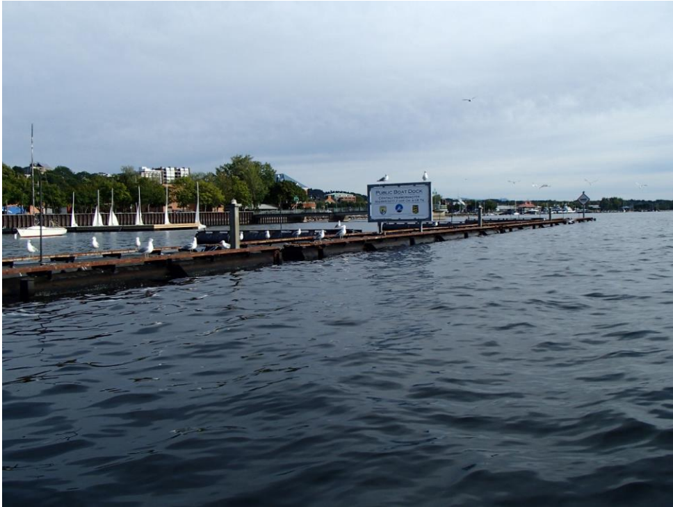
ADJACENT FLOATING ATTENUATOR AT COMMUNITY SAILING CENTER
