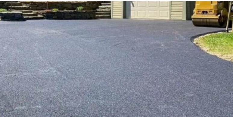
I. Porous Asphalt Vendor: S.T. Paving
