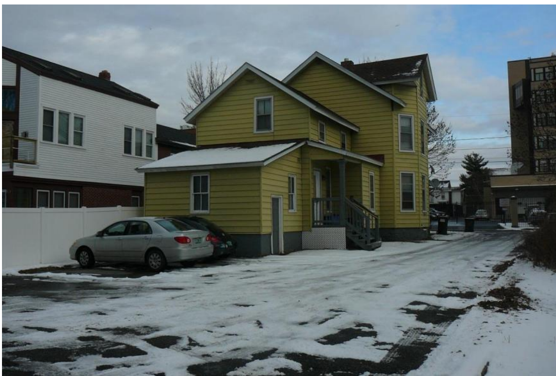
Figure 75. View northeast of west and south elevations of 19 George Street.
