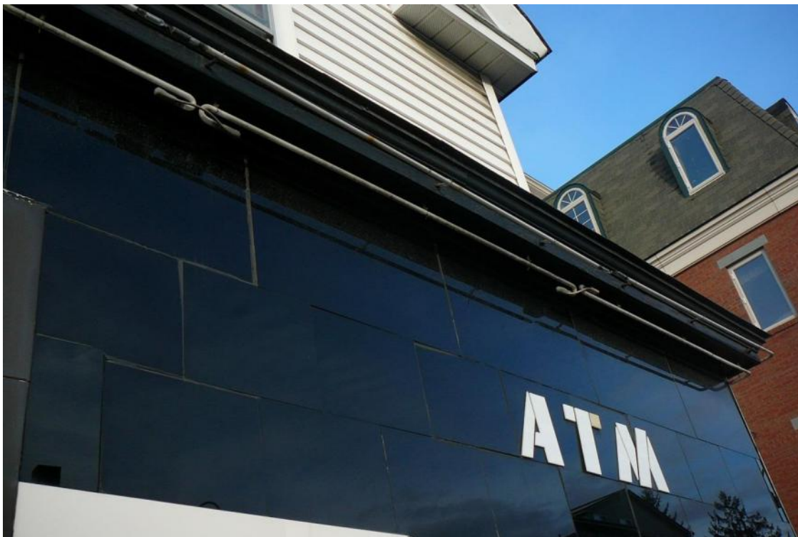
Figure 57. View of top of Carrara glass storefront of 64 Pearl Street.
