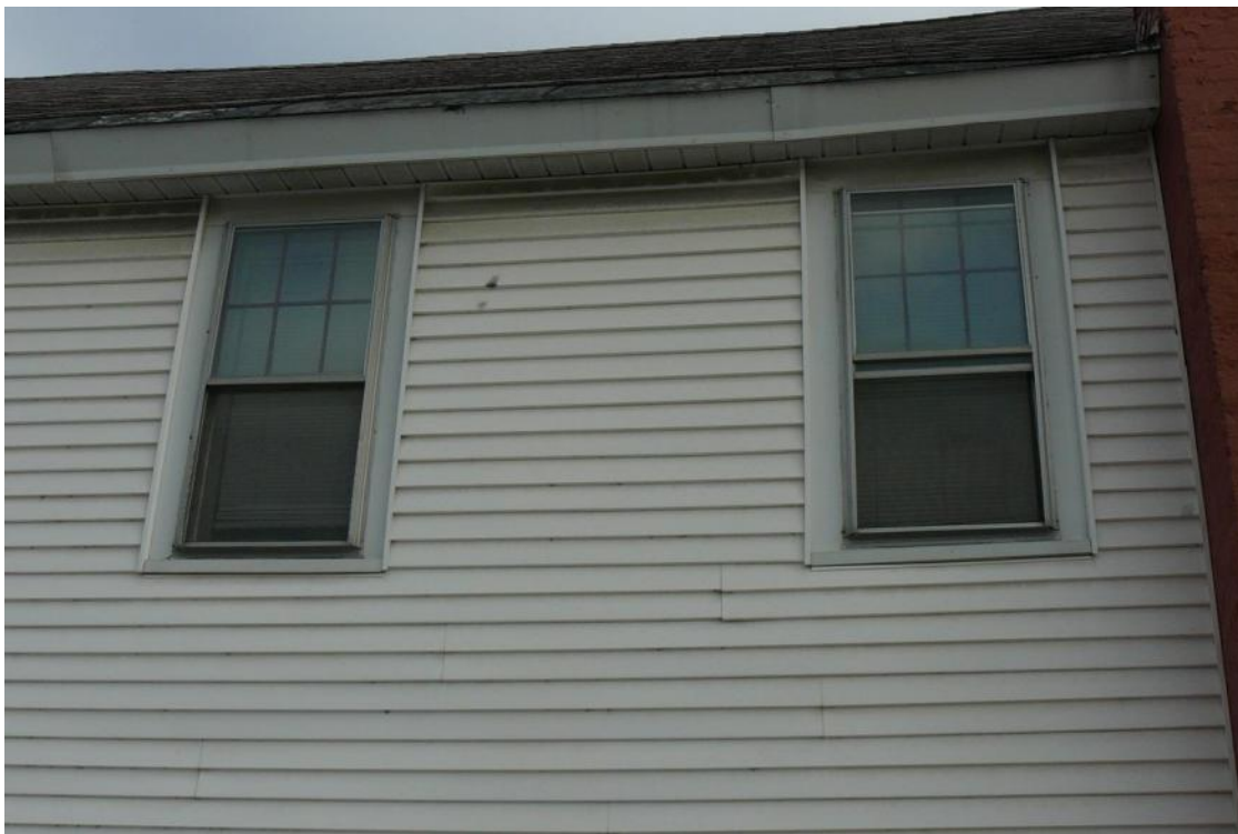
Figure 51. View of typical 6/1 windows at second story on west side of 64 Pearl Street.
