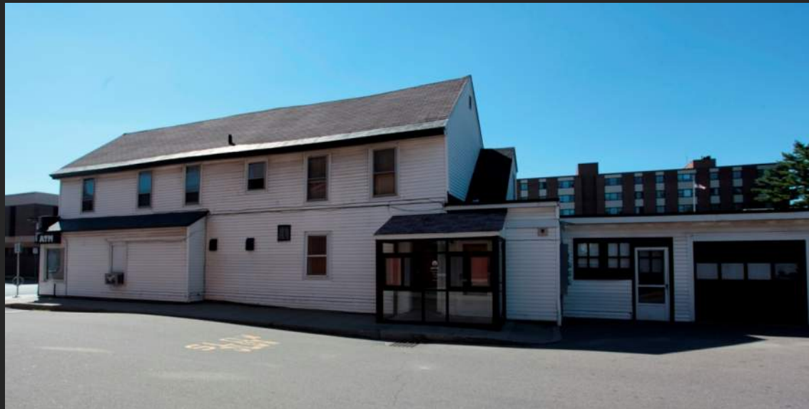
Existing Conditions – Pearl St.
