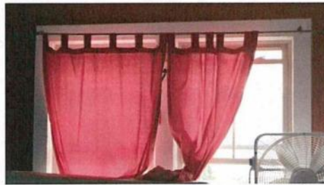
Second floor front windows with simple trim typical of trim in wing.
