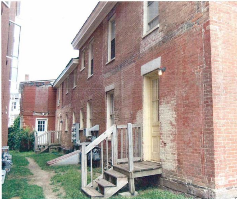
Rear (west) side of main block and wing and south side of cinder block addition. Redstone foundation, smaller added windows, ghosts of former porches visible. Note proximity of east wall of Victoria Place on far right.
