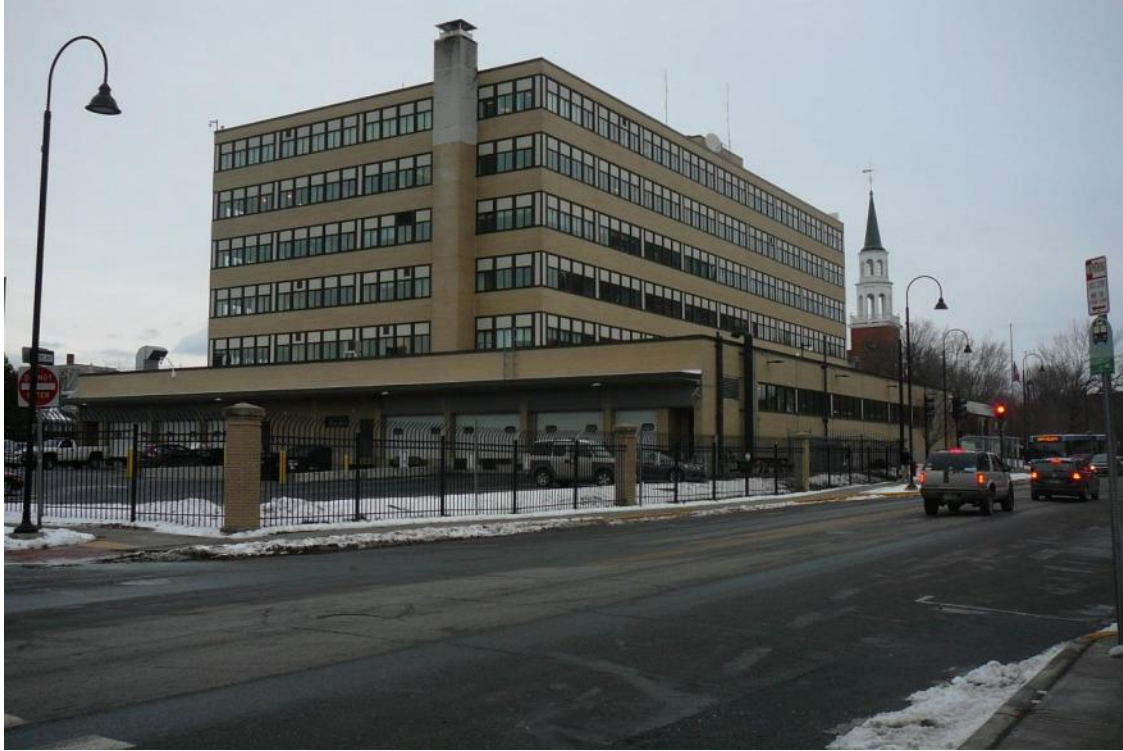
Figure 13. View northeast of building immediately east of project area at the corner of Pearl and George streets.
