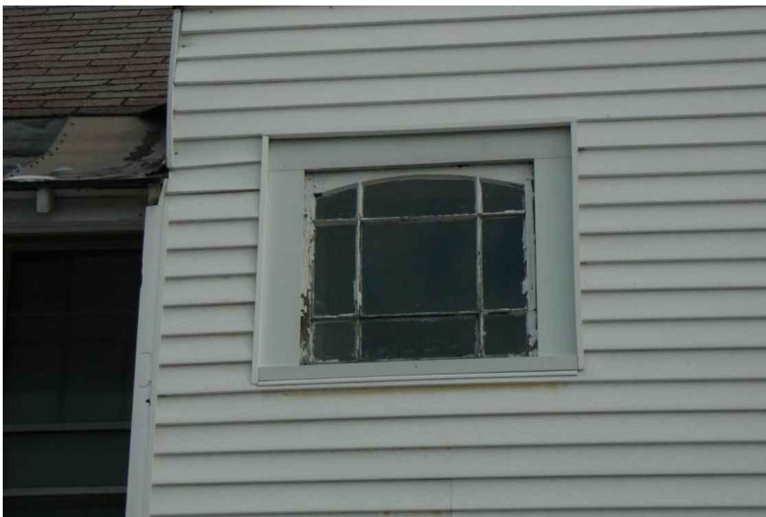
Figure 52. View of second story window on west side of 64 Pearl Street (stairwell wing).
