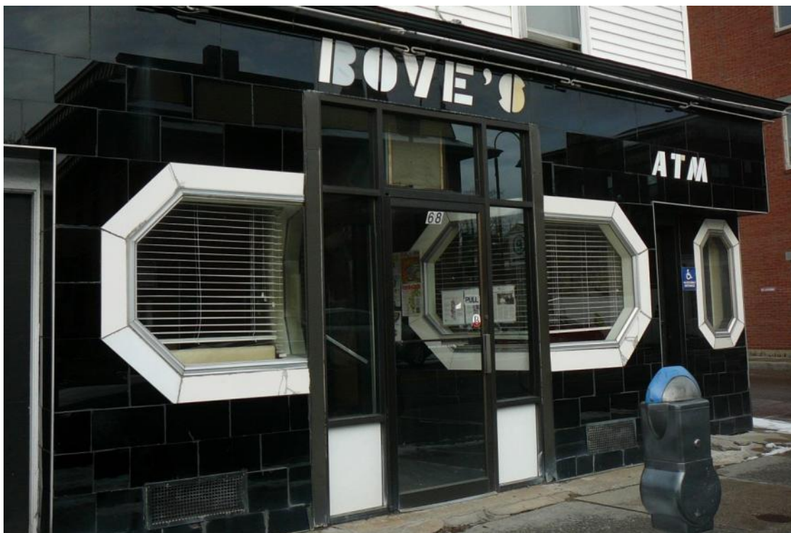
Figure 55. View of Carrara glass storefront of 64 Pearl Street.
