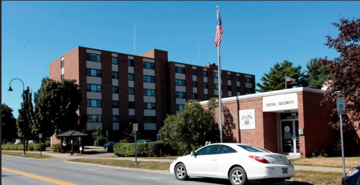
Existing Conditions – Pearl St.
