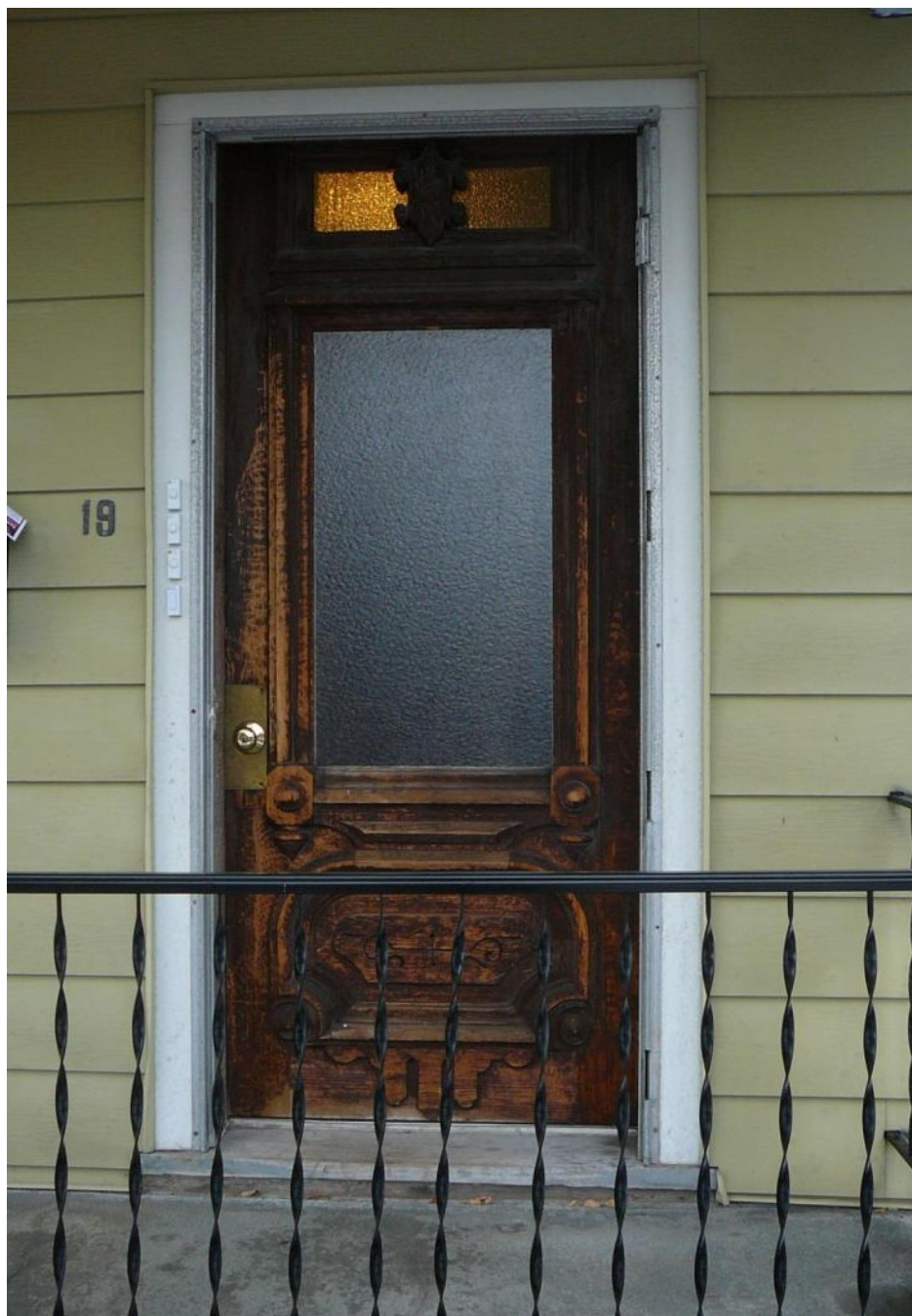
Figure 79. View of main entry door under porch on east elevation of 19 George Street.
