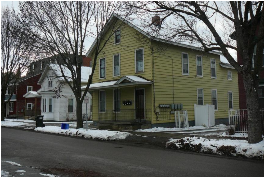
Figure 72. View southwest of east and north elevations of 19 George Street.
