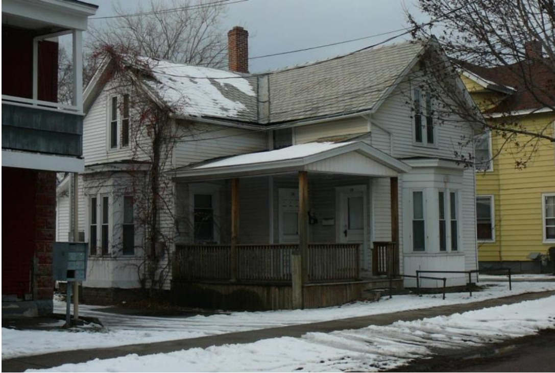
Figure 70. View northwest of east and south elevations of 3 George Street.
