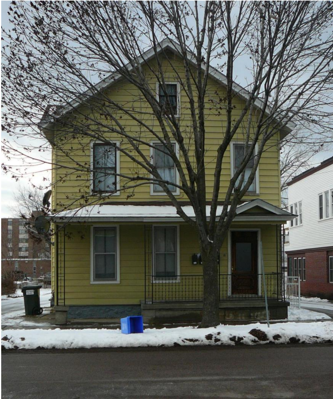
Figure 71. View west of east elevation of 19 George Street.
