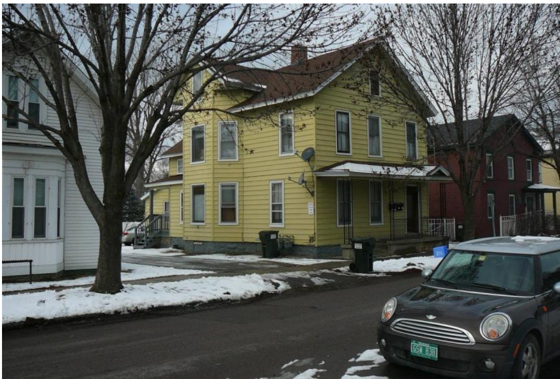
Figure 74. View northwest of east and south elevations of 19 George Street.
