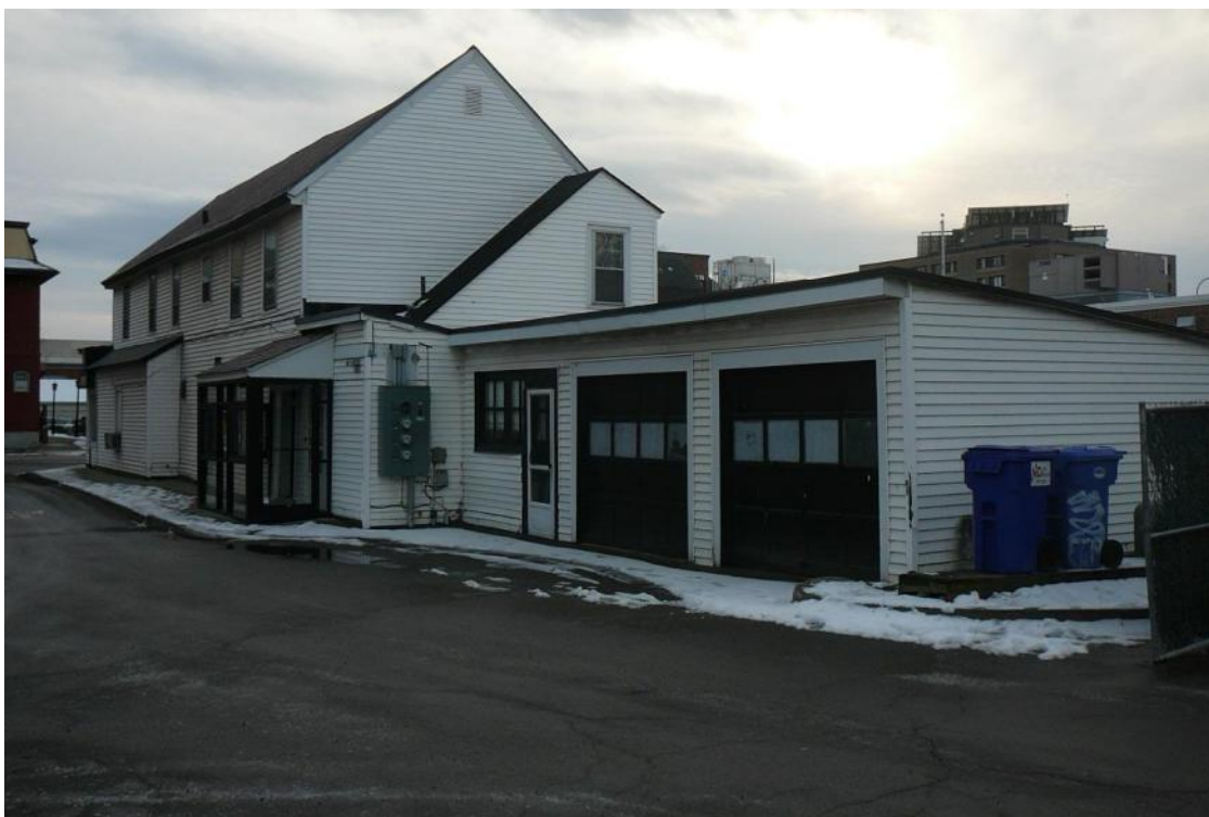
Figure 44. View southwest of east elevation 64 Pearl Street.
