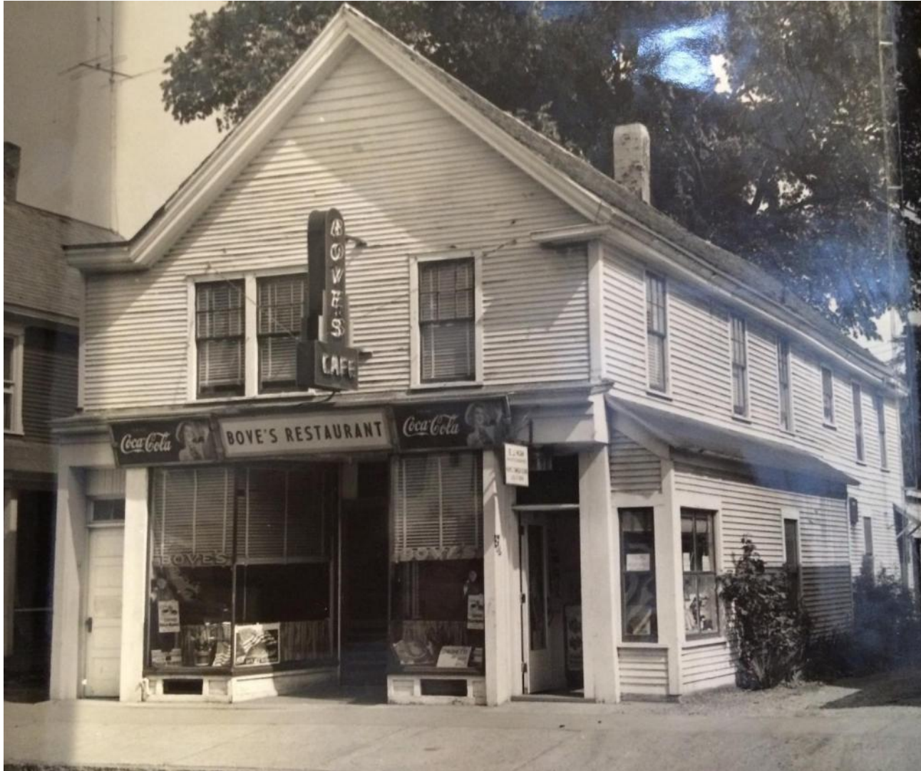
Figure 65. View northwest of 64 Pearl Street in ca. 1942 prior to the addition of the pigmented structural glass storefront (photo on file VTDHP).
