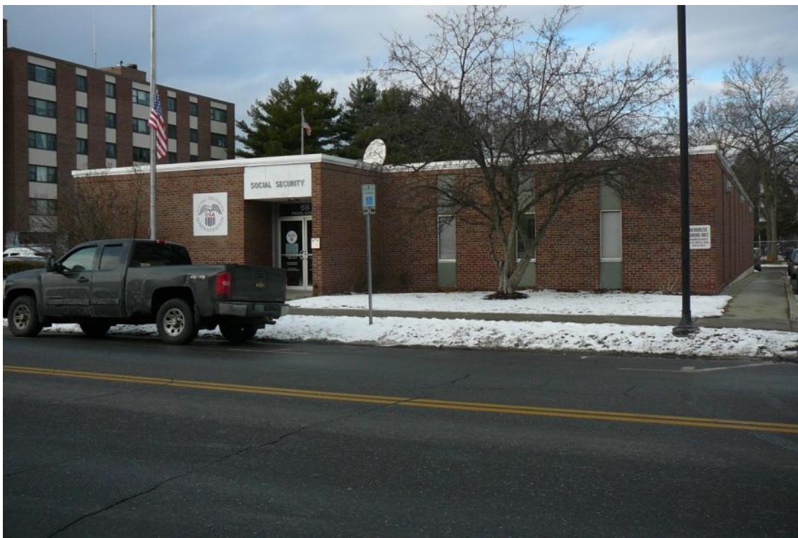
Figure 10. View northwest of buildings immediately west of project area along north side of Pearl Street.
