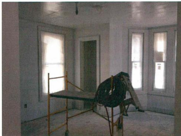
Interior of 13 George with sheetrock walls and flat trim.
