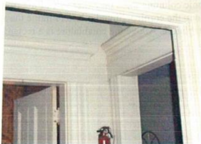
Molded cornices over doors and trim on first floor.
