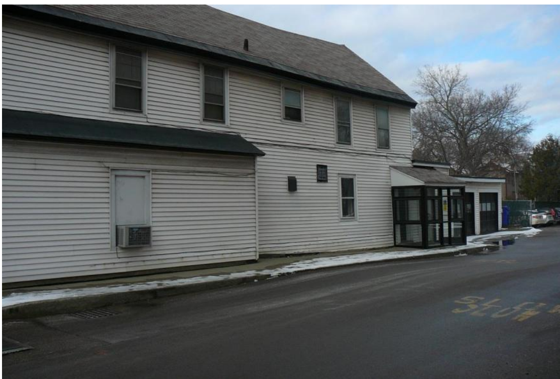
Figure 46. View northwest of east elevation of 64 Pearl Street.
