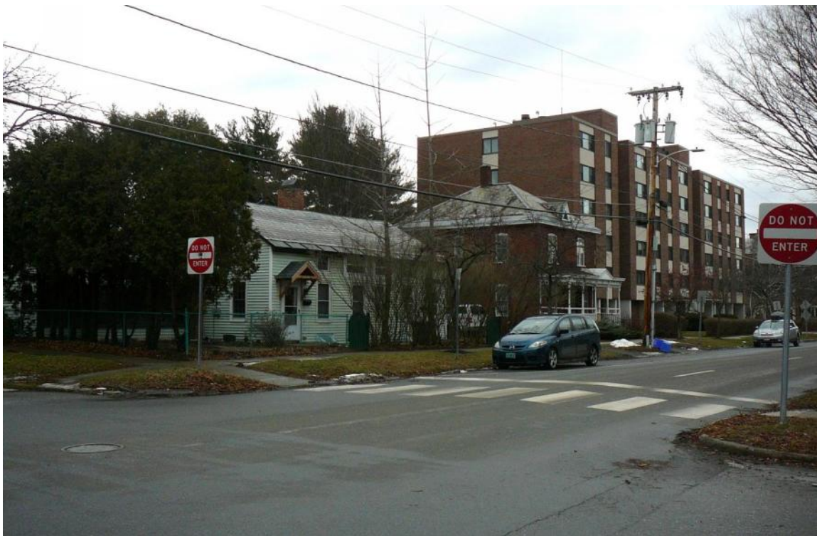
Figure 22. View southeast of buildings along the east side of North Champlain Street (left to right) 30-32, 24 and 10 North Champlain Street.
