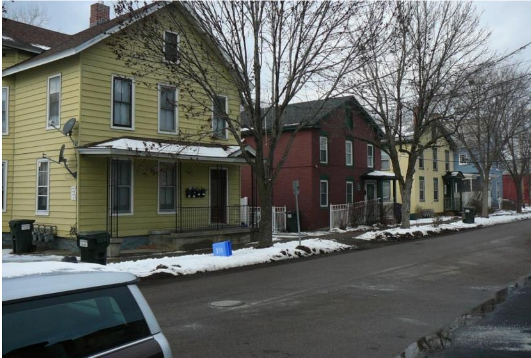
Figure 88. View northwest along George Street; (left to right) 19, 23, 27 and 31 George Street.
