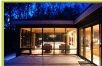
MAFCO HOUSE: This luxurious cottage getaway features Inline Fiberglass 400 Series Commercial Strip with 700 Series operable vents to take advantage of the stunning surroundings.
