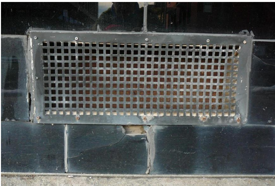
Figure 60. View of grate at base of Carrara glass storefront of 64 Pearl Street.
