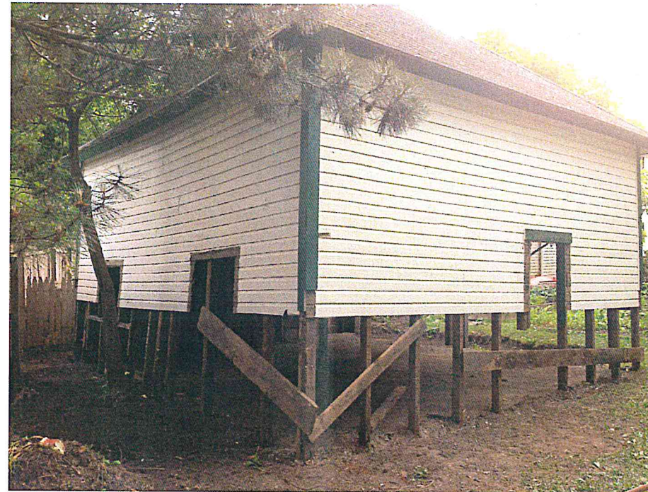
CARRIAGE HOUSE DEMO WORK
