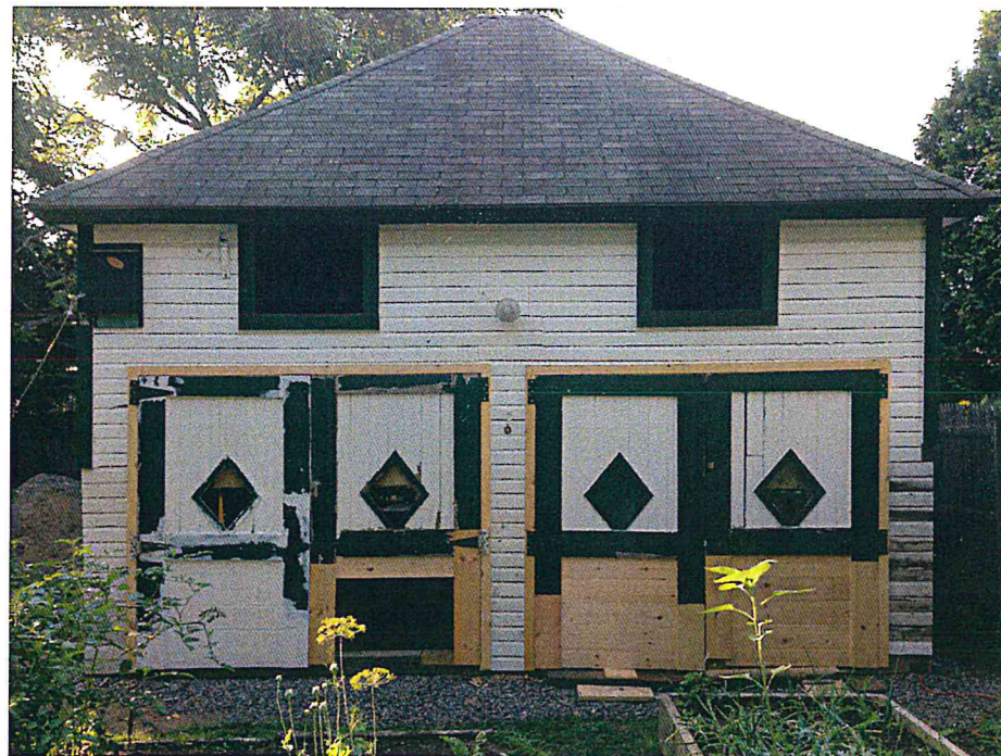
CARRIAGE HOUSE NEW DOORS, TRIM AND SIDING
