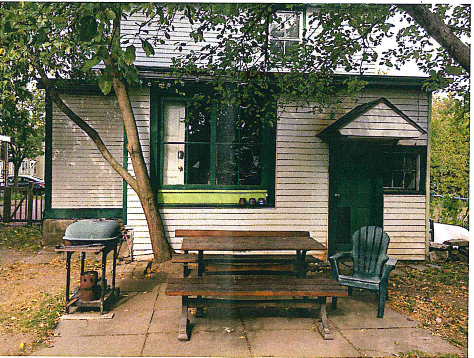
VIEW OF BUILDING FROM BACK YARD
