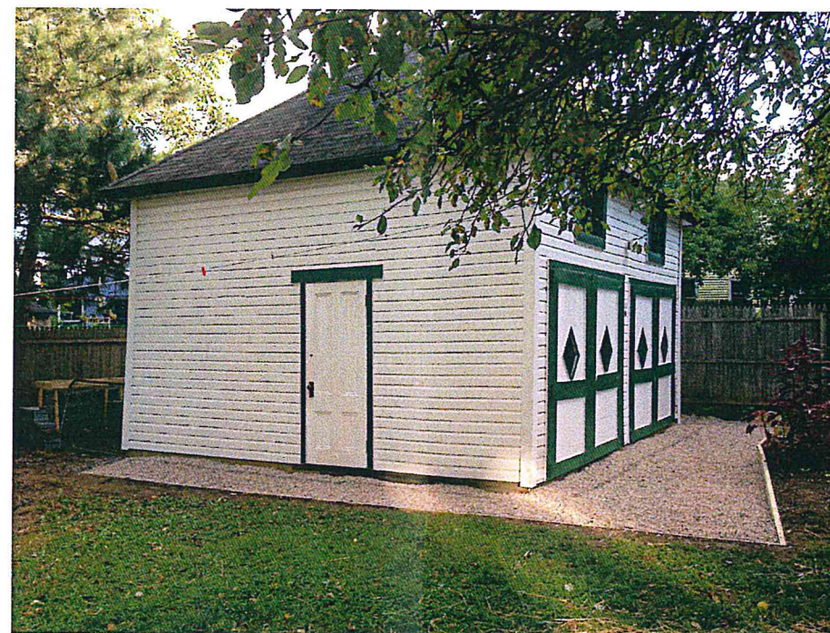
CARRIAGE HOUSE AFTER RENOVATION FROM NORTH
