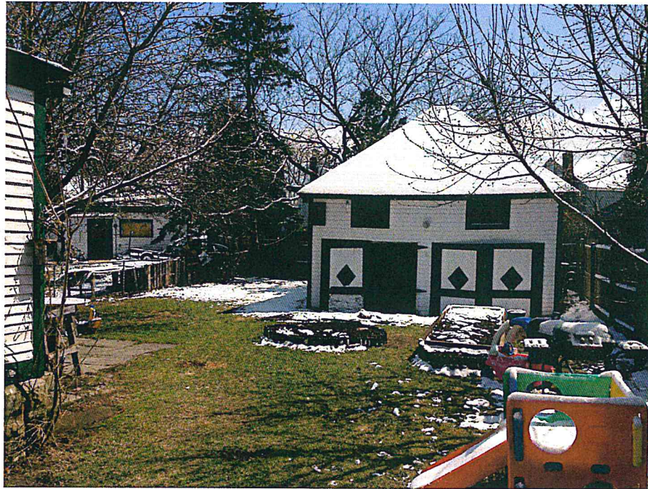
CARRIAGE HOUSE BEFORE RENOVATION
