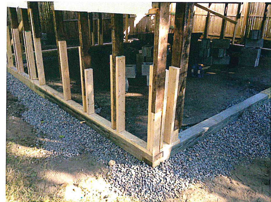
CARRIAGE HOUSE- SISTER EXG STUDS AND ADDING NEW SILL
