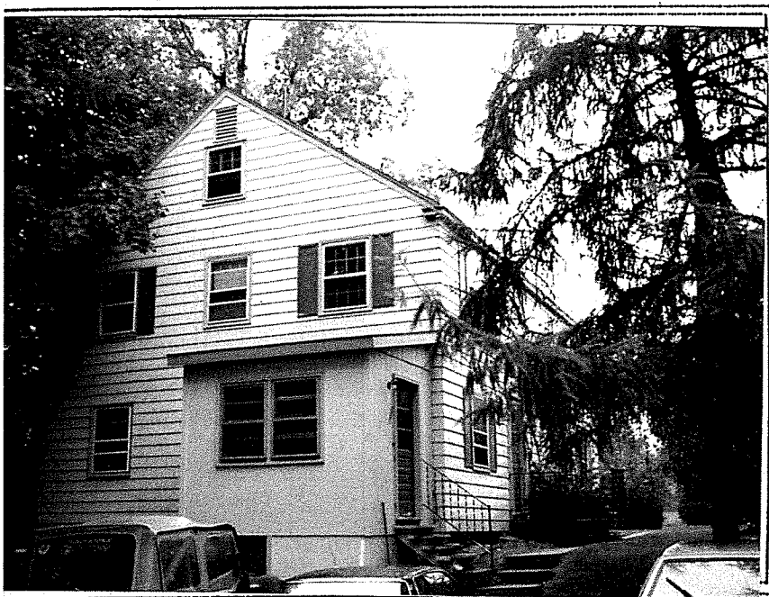
Rear View 201 So. Prospect St. Burlington, VT
