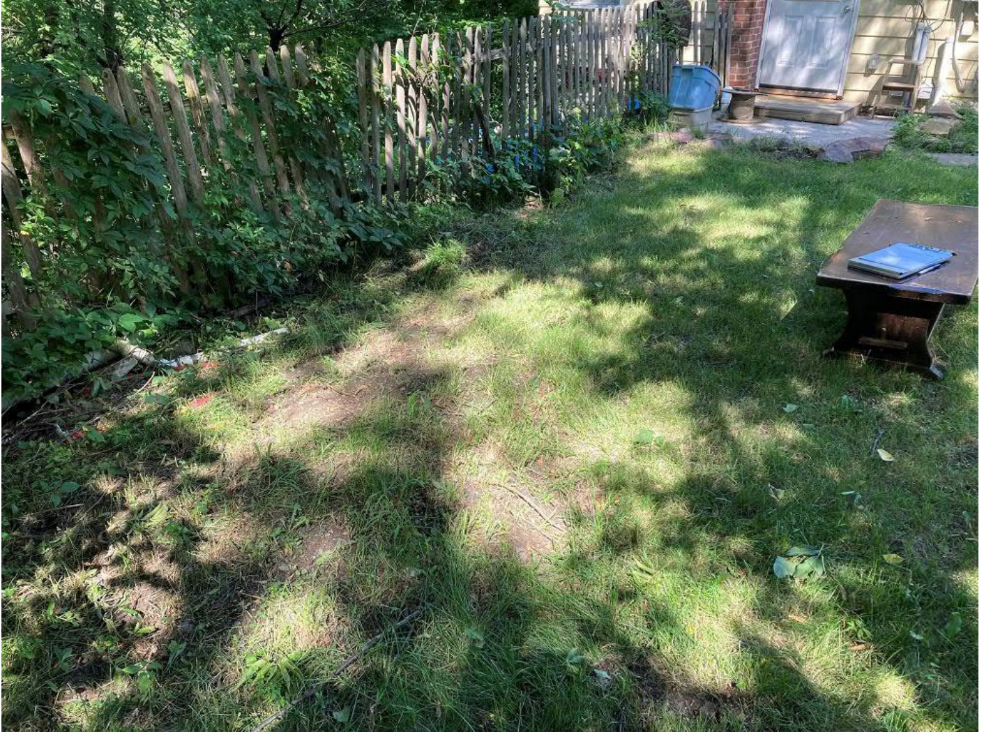
Photograph 11: View to northeast, west of residence, showing incipient slumping at top of slope, left-center of photograph; note disturbed fencing where soil scarp is beginning to form.
