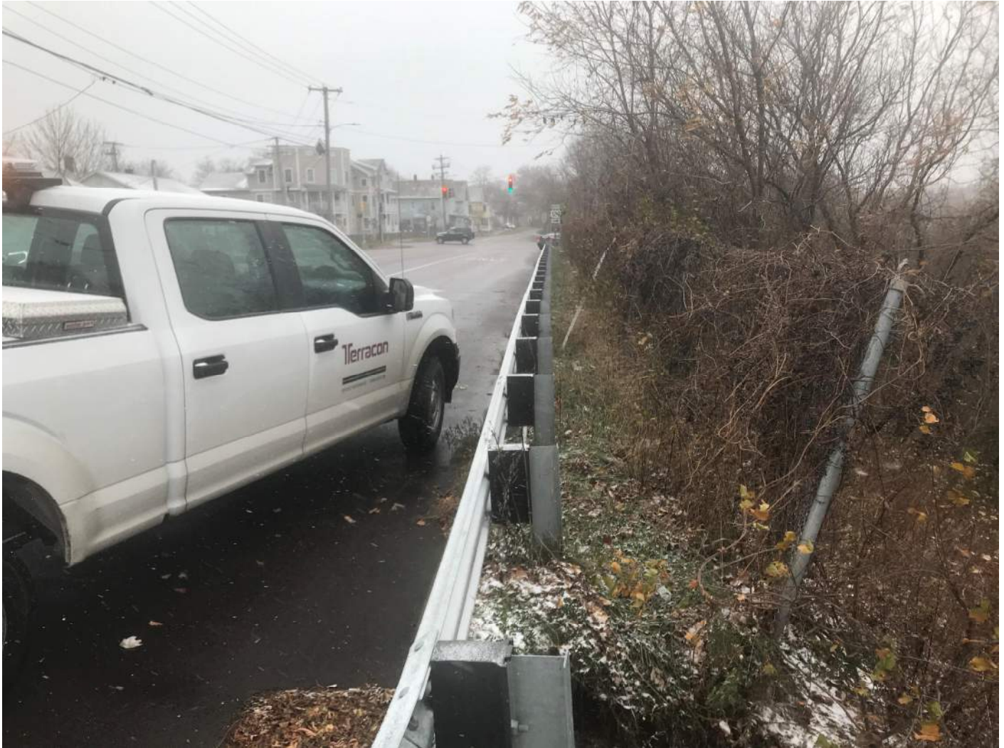
Photograph 10: View to west along Manhattan Drive showing the top of the natural slope on western flank of remediated slope; no transverse stress cracking in pavement and guard rail shows no sign of movement; fence section may have been damaged during remediation of slope
