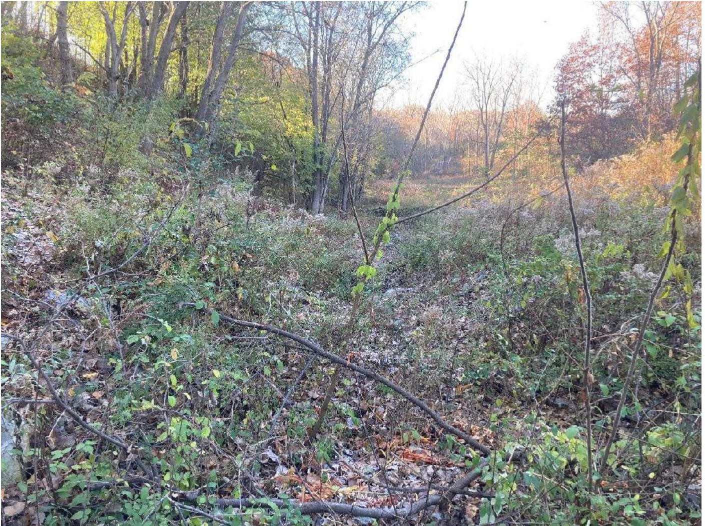
Photograph 2: View to northwest of stone-lined stormwater discharge channel at base of slope and downstream from Culvert 1; drainage designed to discharge to wetlands at top right of photograph; note density of vegetative overgrowth within channel (compare with Photographs 3 and 4).
