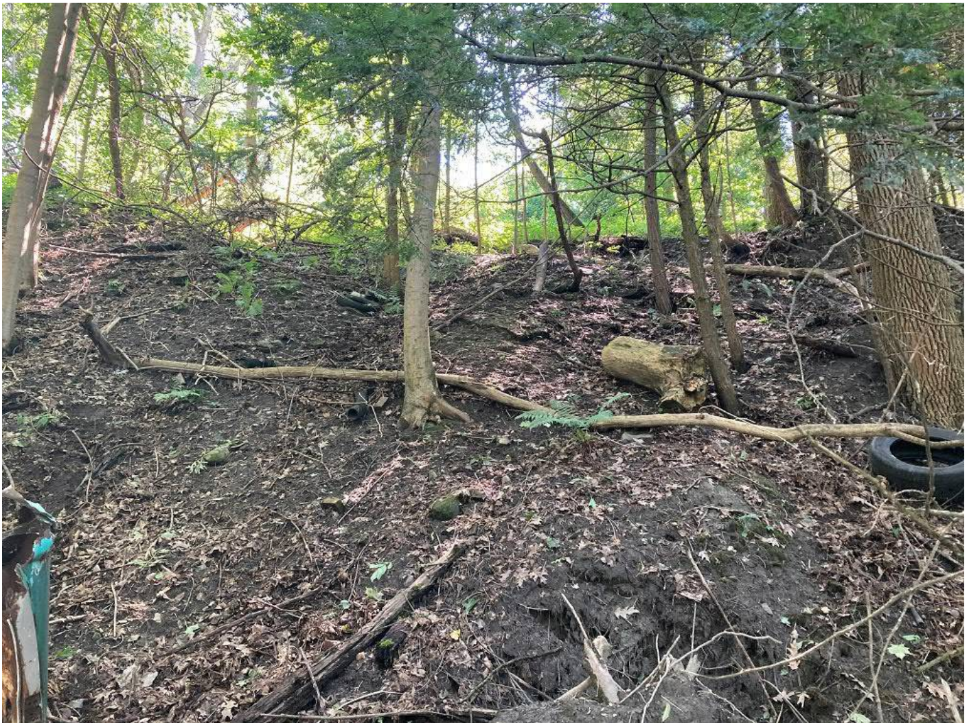
Photograph 8: View to south-southwest towards Burlington Collision showing exposed, unvegetated, historic slump/slide debris; exposed soil mass subject to continual erosion during precipitation.
