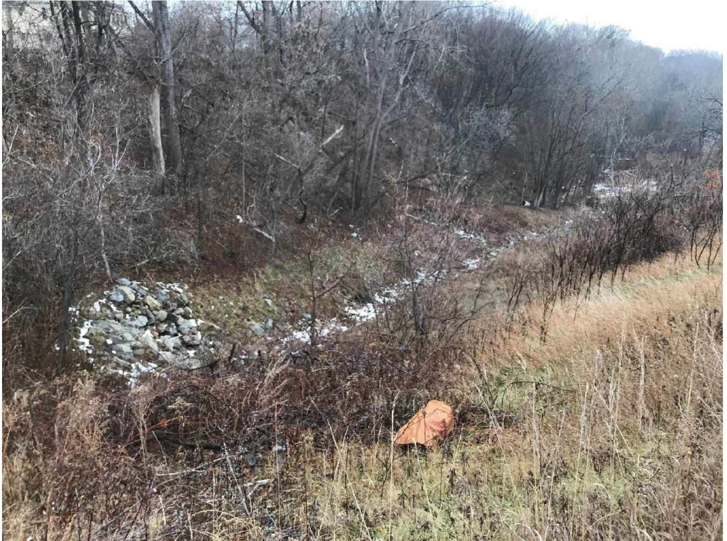
Photograph 4: View to west south-west taken in November 2019 during Hoyle, Tanner & Associates inspection showing well-defined Culvert 1 discharge channel at base of slope.
