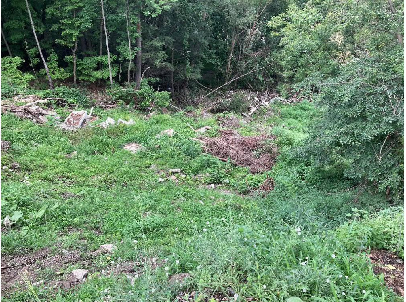
Photograph 26: View to north of overgrown historical slide/slump debris from top of failure scarp between 365 and 389 Riverside Avenue
