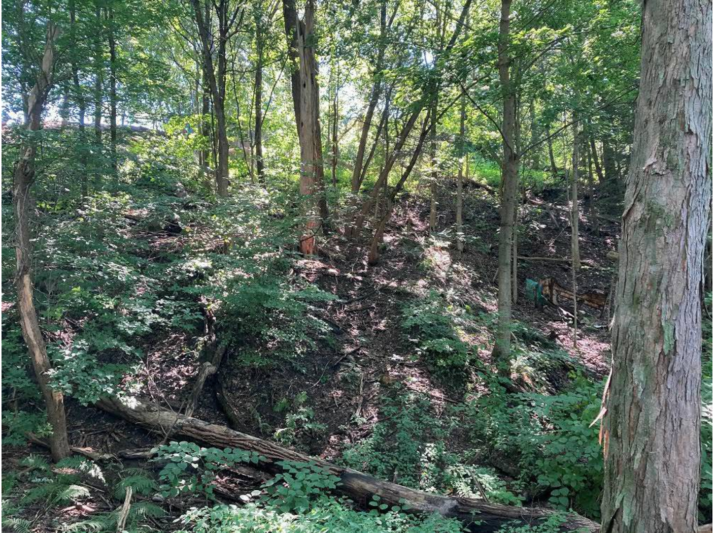
Photograph 10: View to south of historic debris slump downslope from Burlington Collision; location of crown cracks at top of slope east of building at upper left; note leaning trees at center of photo and exposed soil surface subject to continual erosion during precipitation events
