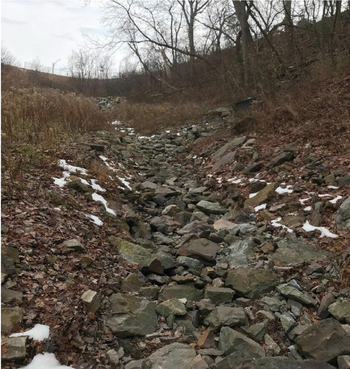
Photograph 3: View to southeast taken in November 2019 by Hoyle, Tanner & Associates of well-lined discharge channel from Culvert 1.
