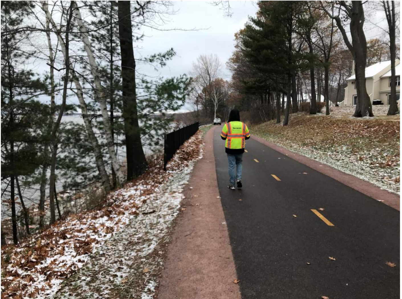
Photograph 9: View to north of bike path at the top of remediated slope; no stress-relief cracking or incipient slumping observed
