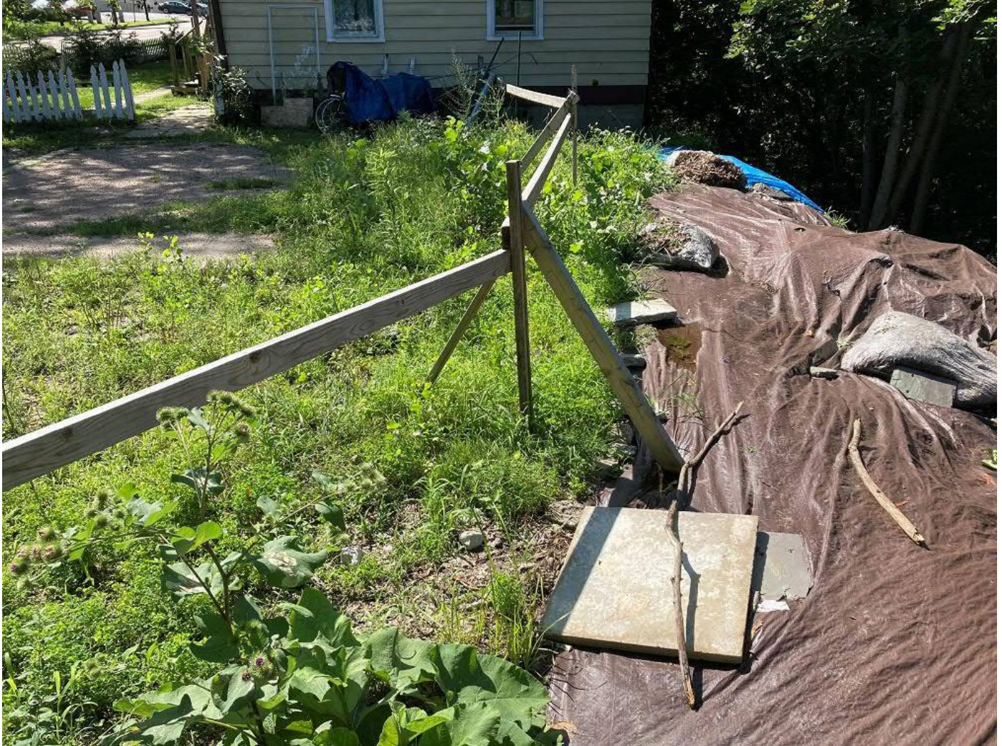
Photograph 16: View to west toward residence showing remediation at top of slope (placement of fabric and rip-rap); no distinct surface cracking or slumping in grassy area south of rip-rap
