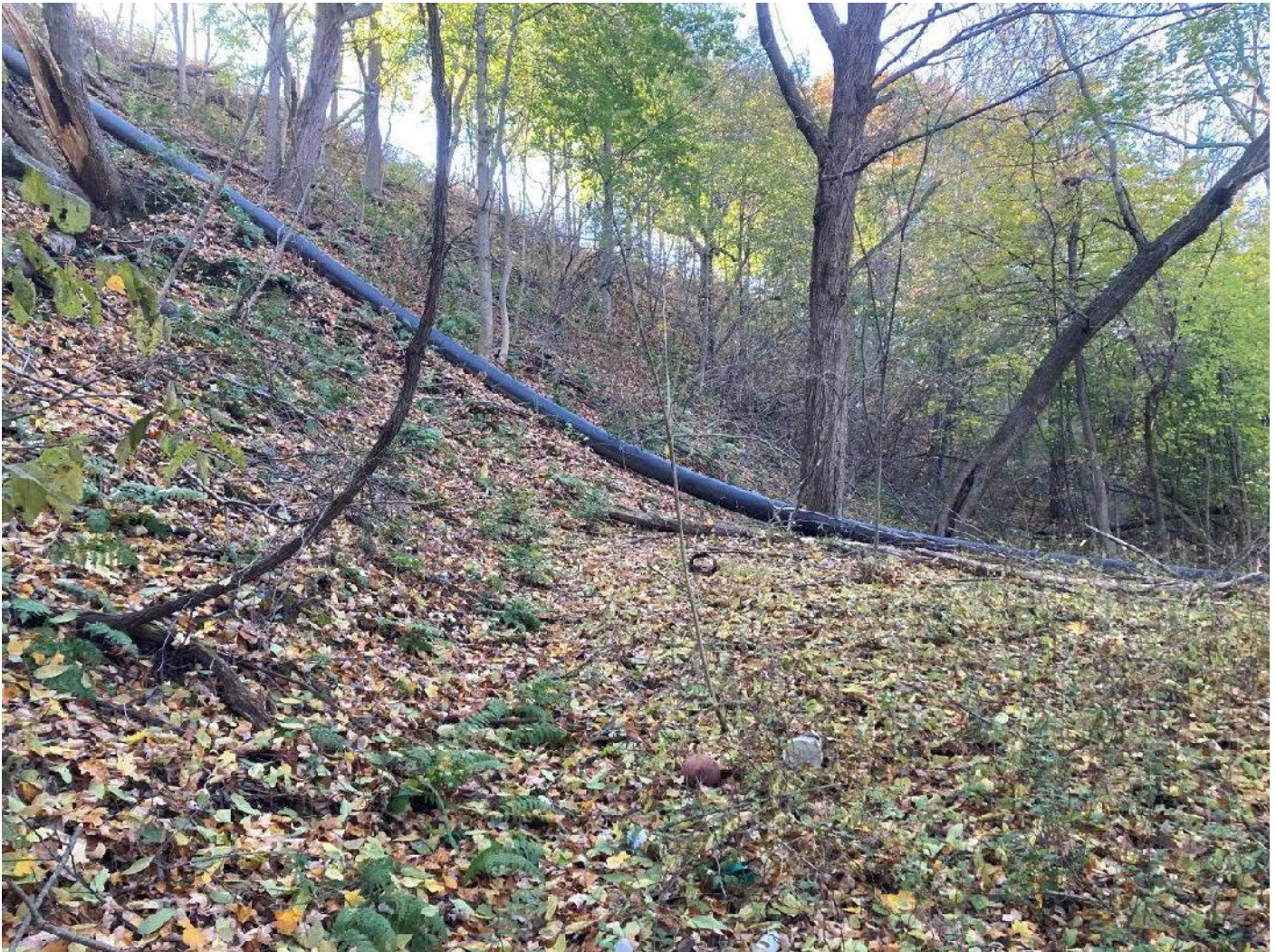
Photograph 13: View to southwest of exposed discharge pipe from Manhattan Drive to Culvert 3.
