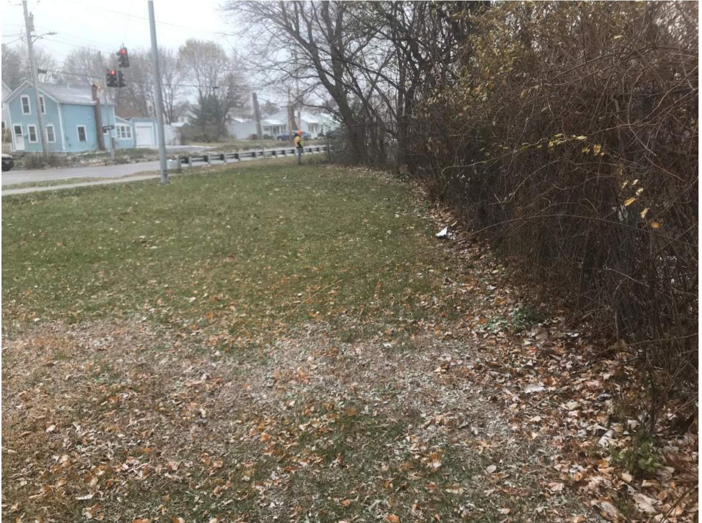
Photograph 13: View to southwest of top of natural slope on eastern flank of remediated slope; no distinct signs of stress or indications of slumping or movement are evident
