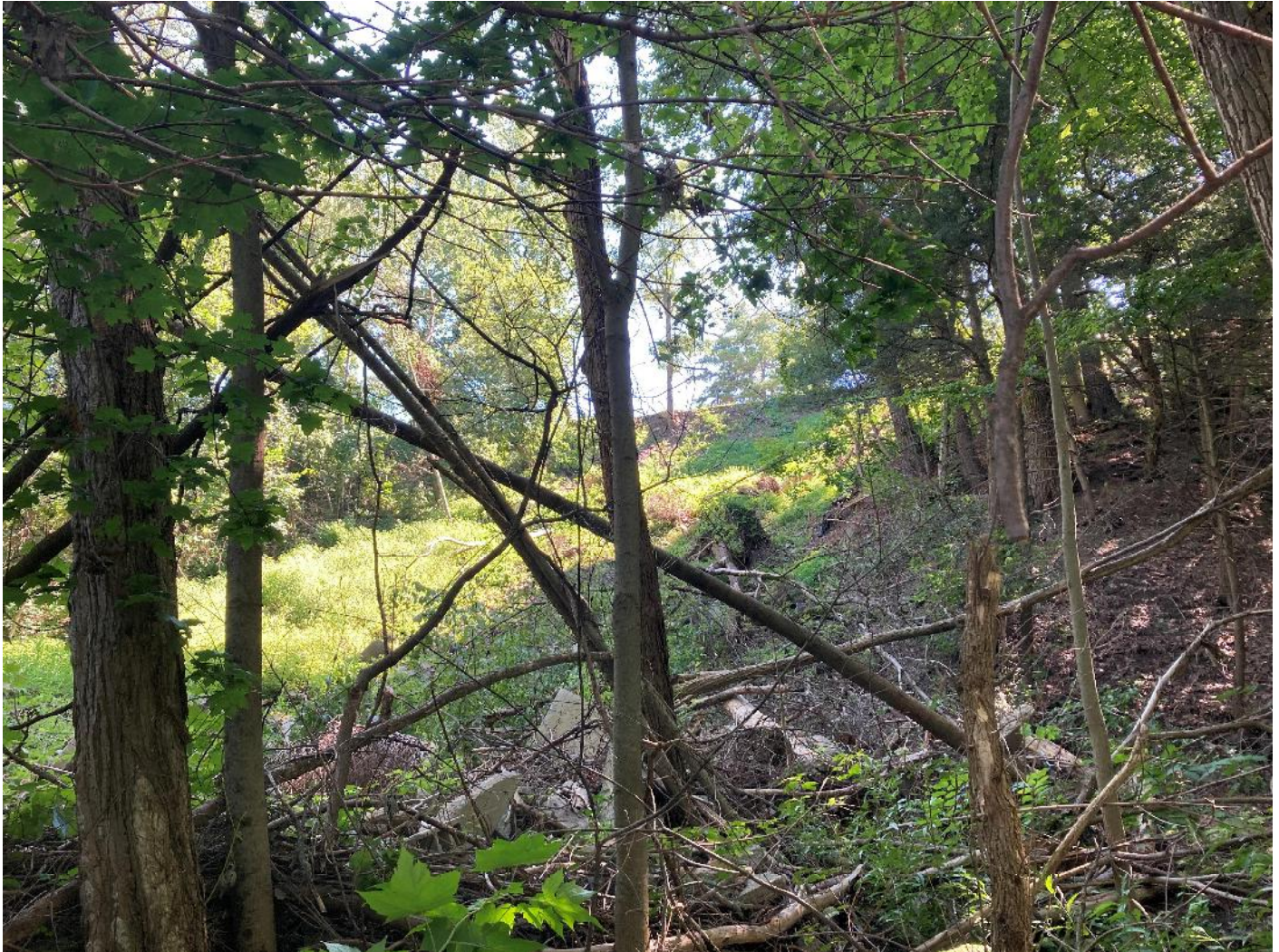
Photograph 22: View to southeast of exposed scarp and slide/slump debris (center of photograph) downslope from area between 389 (private residence) and 365 Riverside Avenue (Hall's Hitches and Welding)
