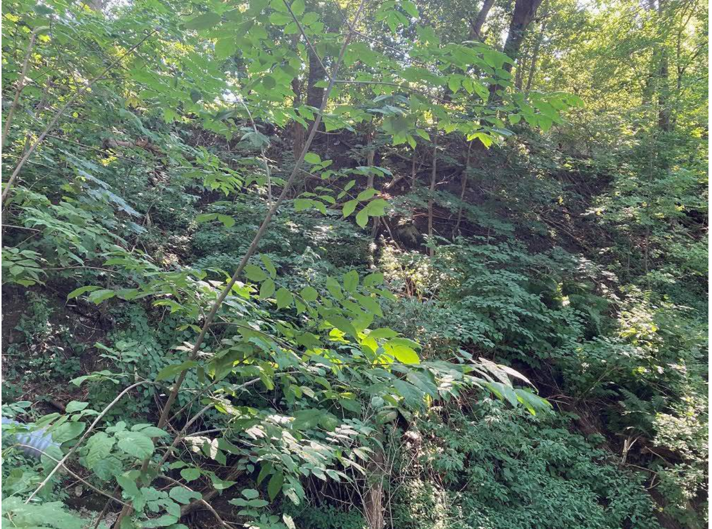
Photograph 16: View to southwest showing exposed soil scarp in slope north of GBG Indian Kitchen parking lot; Kismayo Kitchen (505 Riverside Avenue) at top right; note density of vegetation and mature trees at top of scarp leaning downslope.
