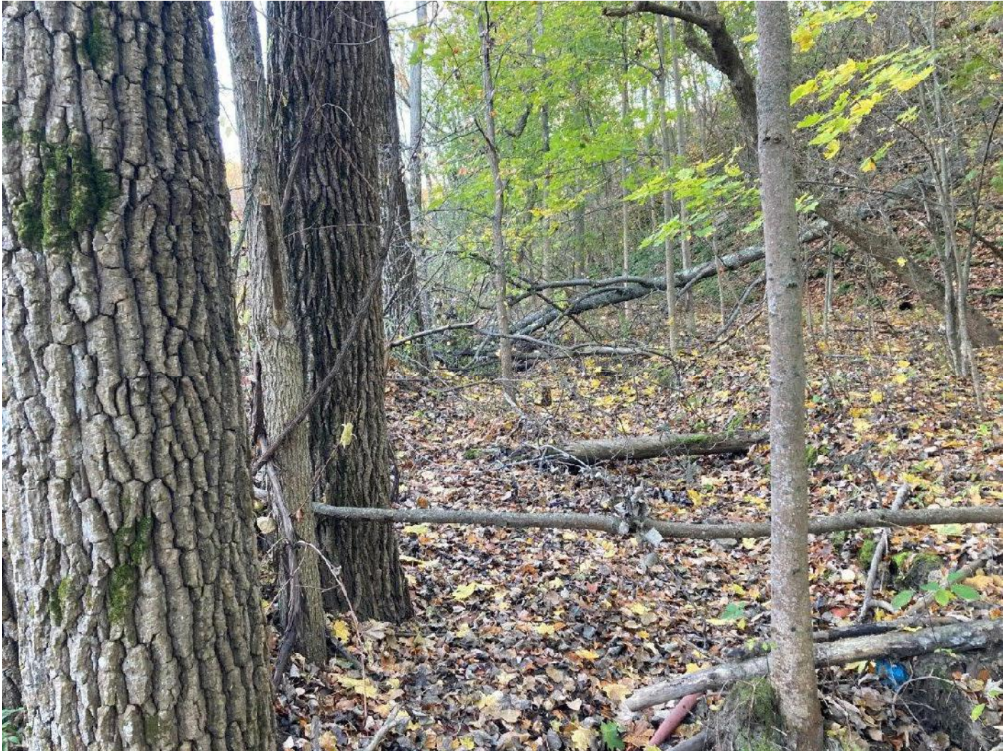
Photograph 16: View to east of unlined discharge channel at toe of slope; note density of overgrowth as compared to Photograph 17.
