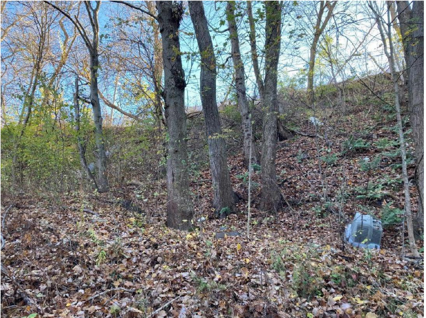
Photograph 6: View to south-southeast toward Manhattan Drive of portion of slope to the west of Culvert 2 discharge pipe (right-center of photograph).
