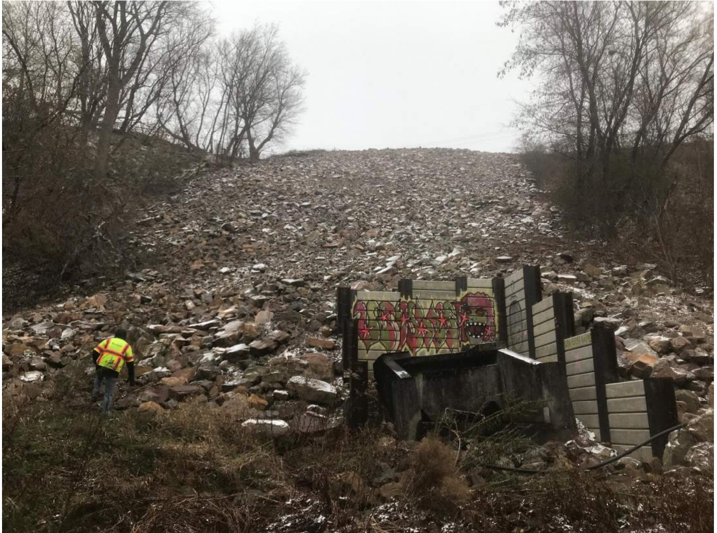
Photograph 1: View to south showing remediated section of slope with boulder rip-rap; stormwater drainage outlet shown in foreground; natural vegetated slopes occur on flanks of remediated slope
