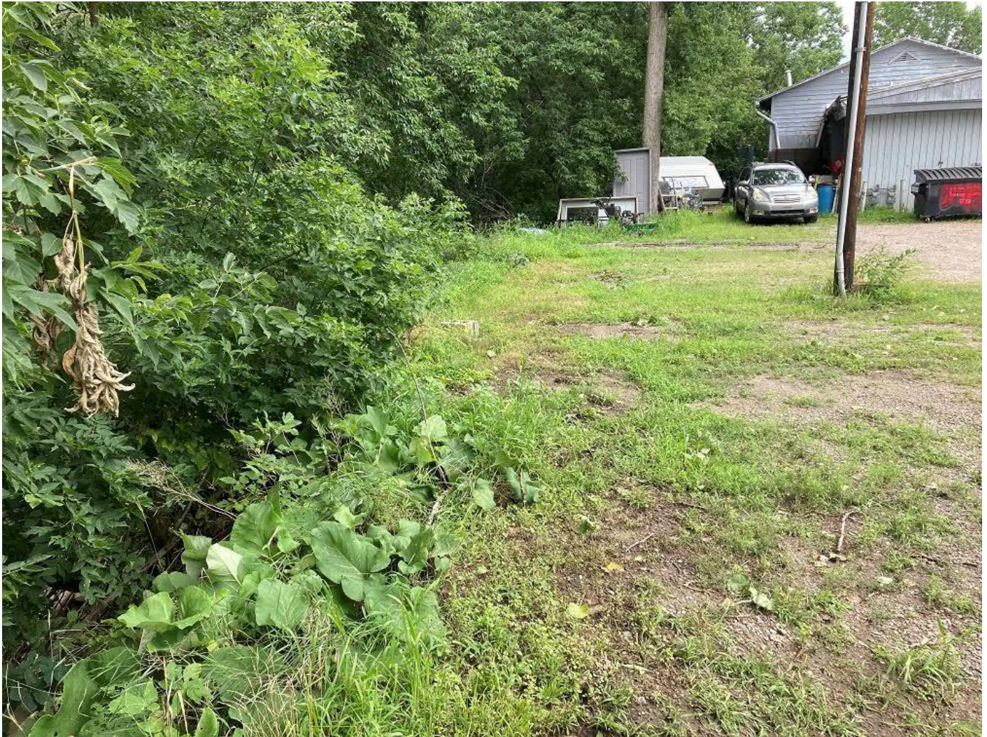
Photograph 27: View to east towards Hall's Hitches building, east of failed slope, showing stable surface platform (i.e. no distinct slumping or crown cracking); possible beginning traces of surface slumping top center of photograph; soil scarp obscured and covered by vegetation at left of photograph
