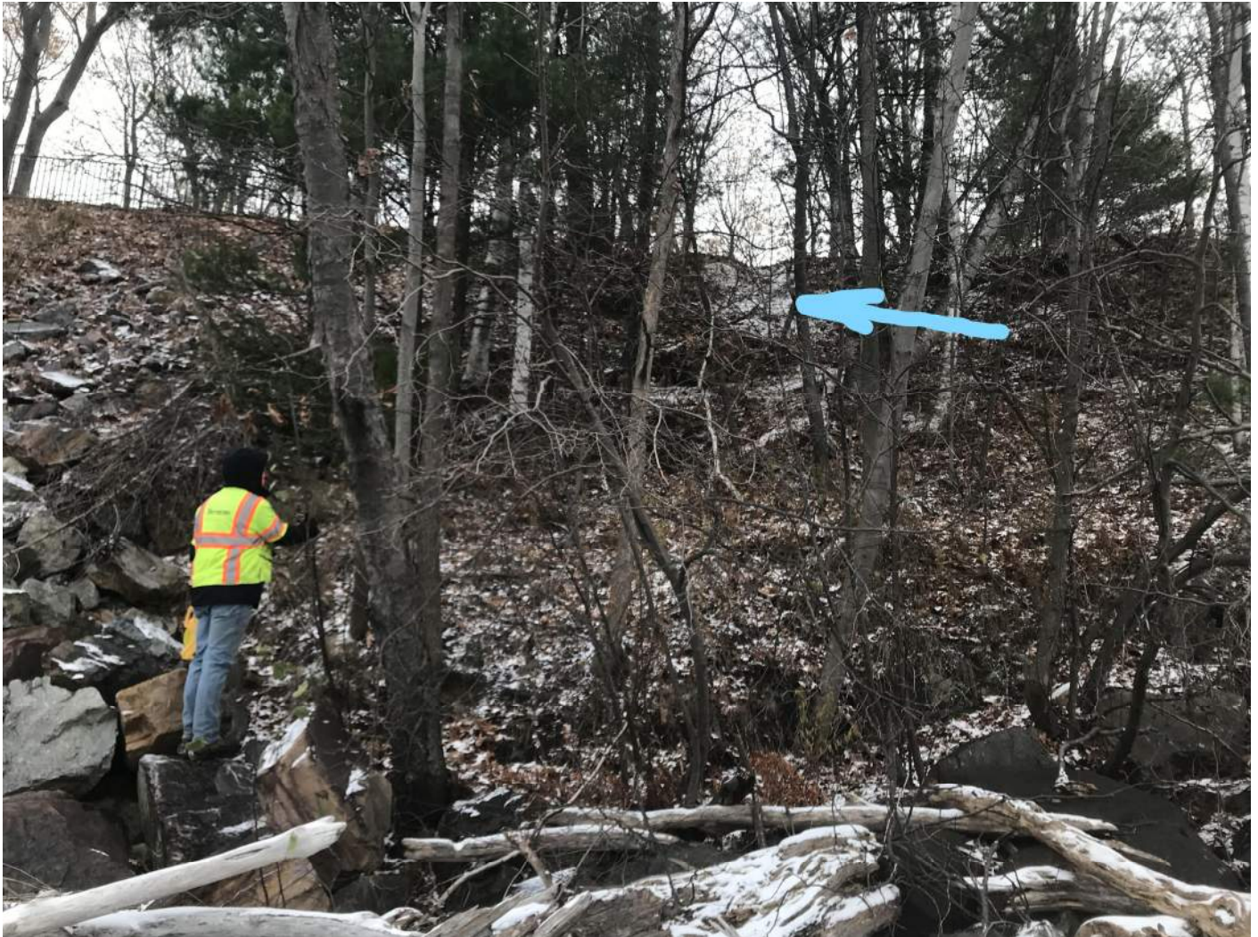
Photograph 7: View to southeast; incipient gullying at top of natural slope caused by surface water run-off
