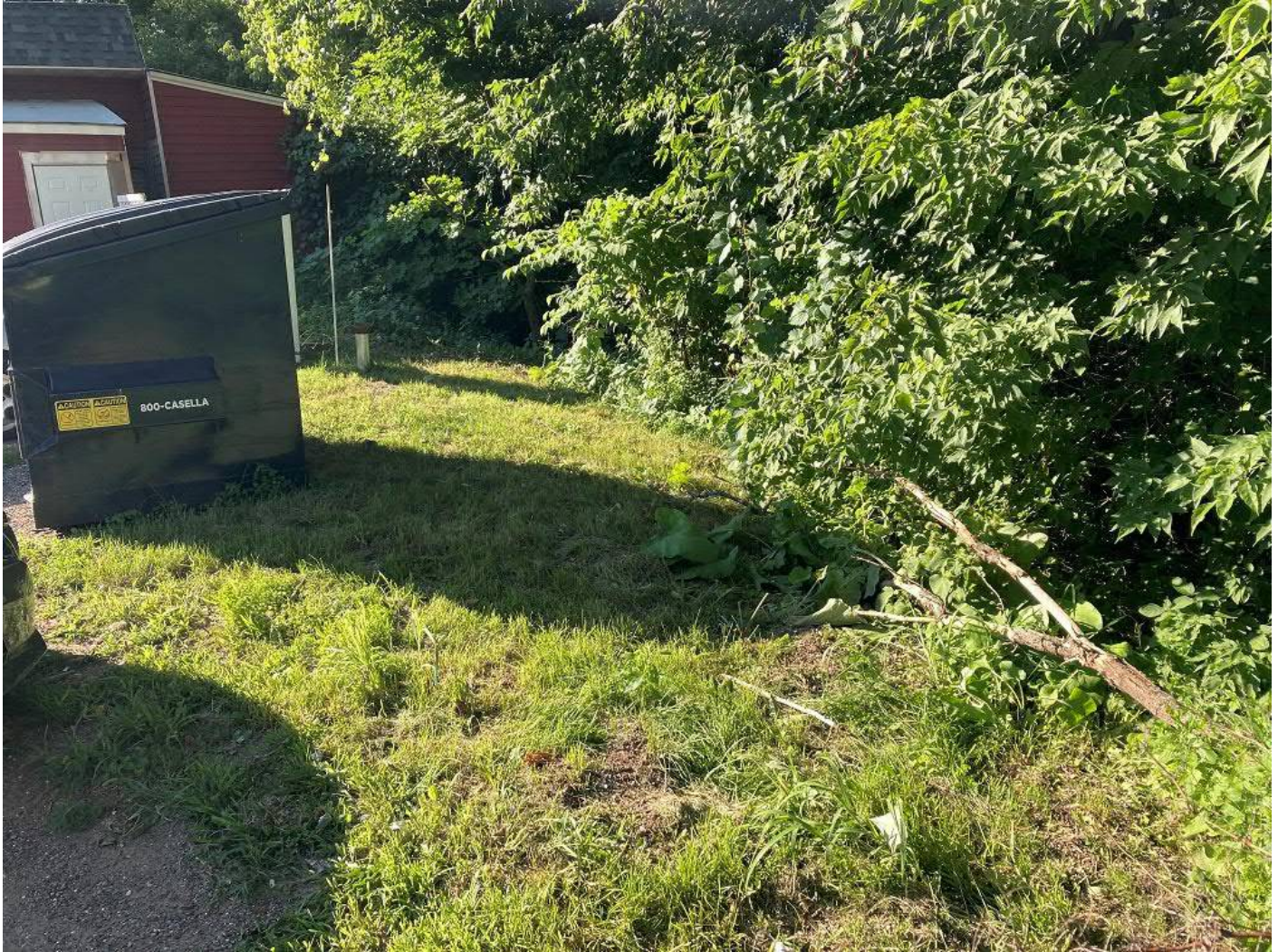
Photograph 4: View to west-northwest of east side of Kismayo Kitchen building, showing slightly irregular ground surface that appears stable; note monitoring well top left; soil scarp at center and center right obscured by vegetation.
