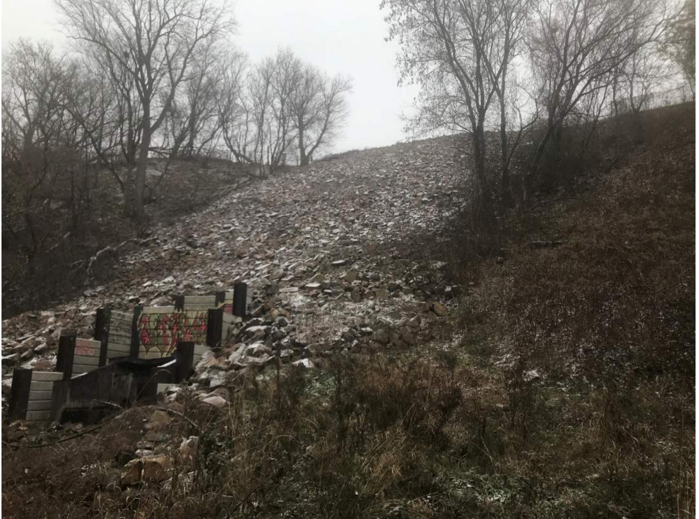
Photograph 2: View to southeast of remediated slope and natural vegetated slopes on eastern and western flanks
