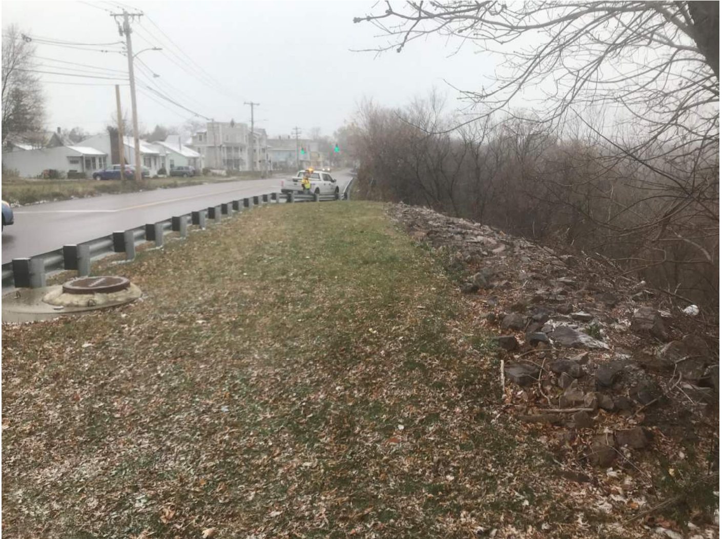
Photograph 9: View to west along Manhattan Drive showing the top of the remediated slope and absence of transverse cracks and slumps indicative of movement
