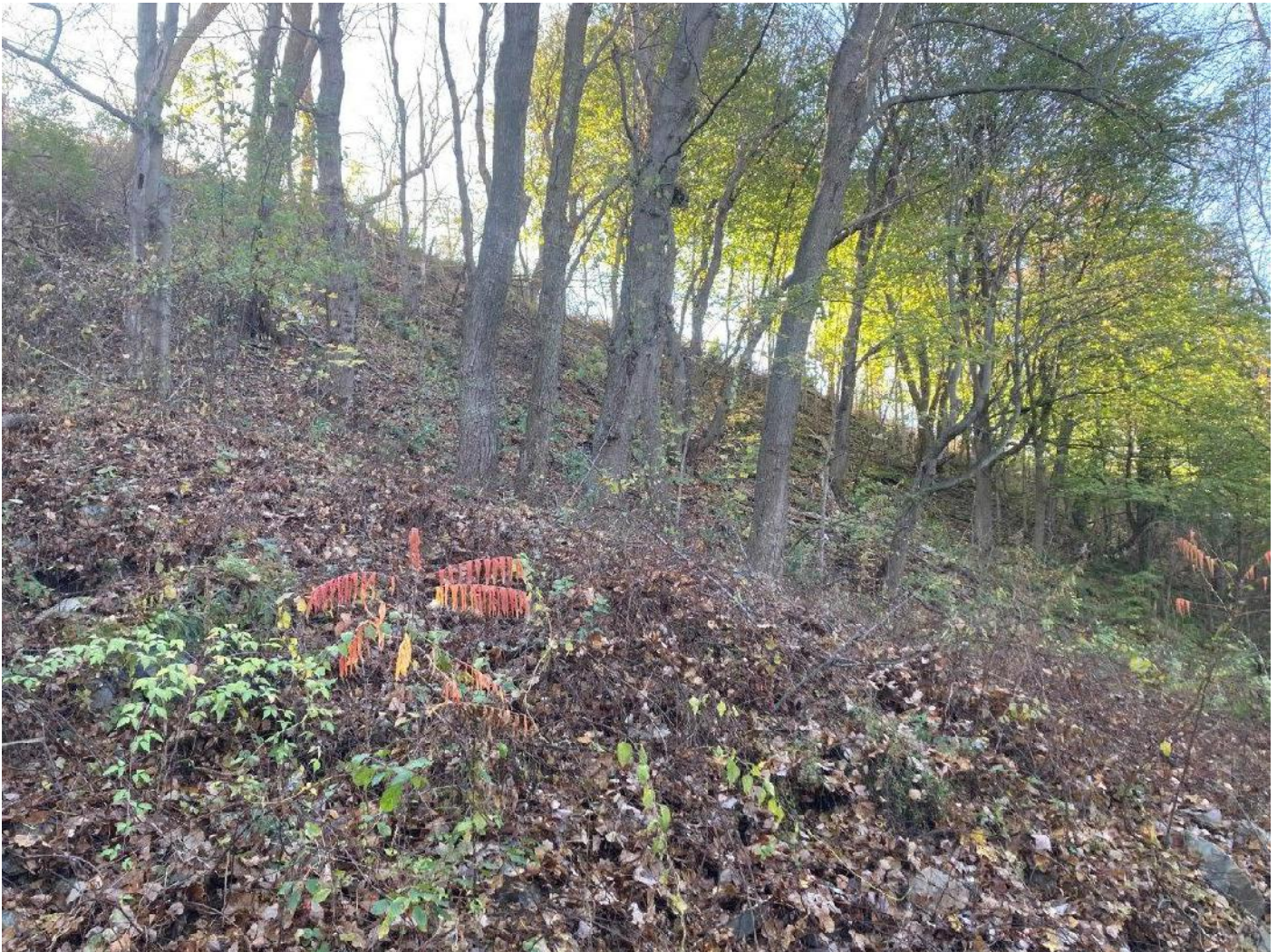
Photograph 7: View to southwest toward Manhattan Drive showing slope west of Culvert 2; stone-lined discharge channel from Culvert 1 at toe of slope in foreground; note lack of distinct lean of trees mid-slope.
