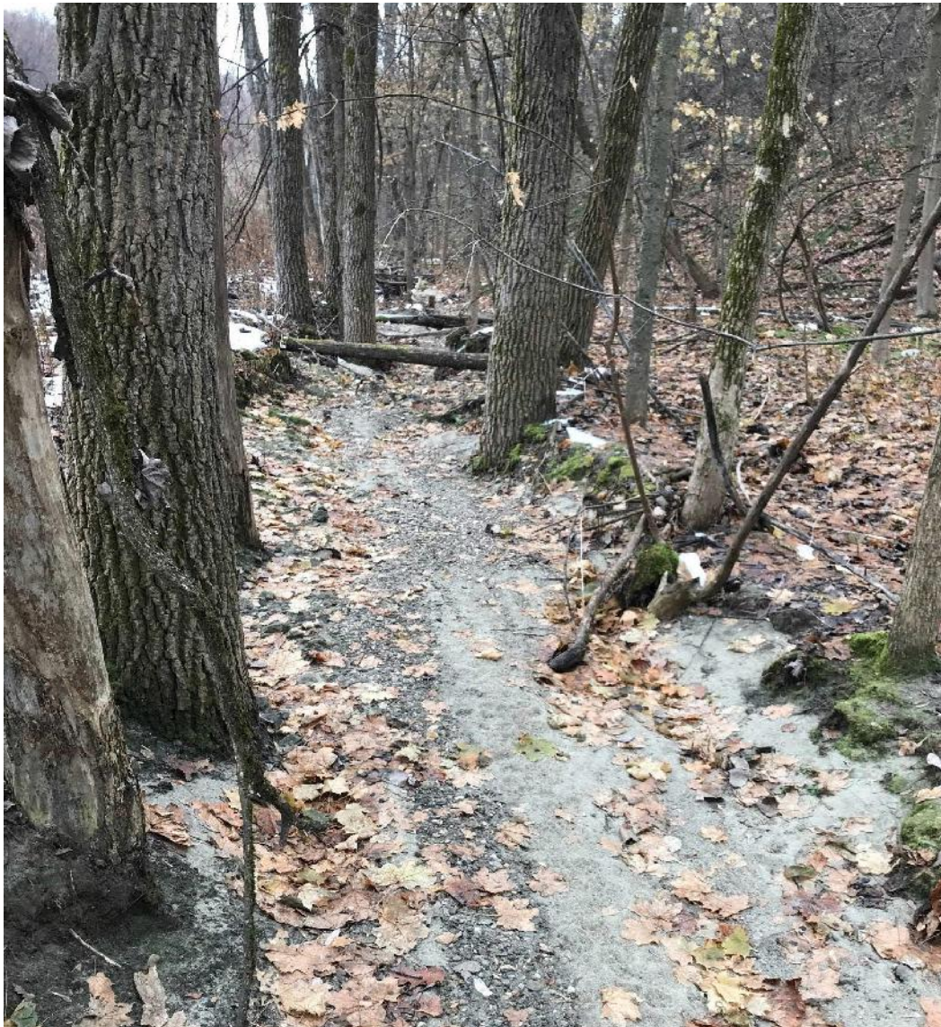
Photograph 17: View to east of unlined discharge channel at toe of slope; note lack of overgrowth and sediment infilling channel (compare to Photograph 16).
