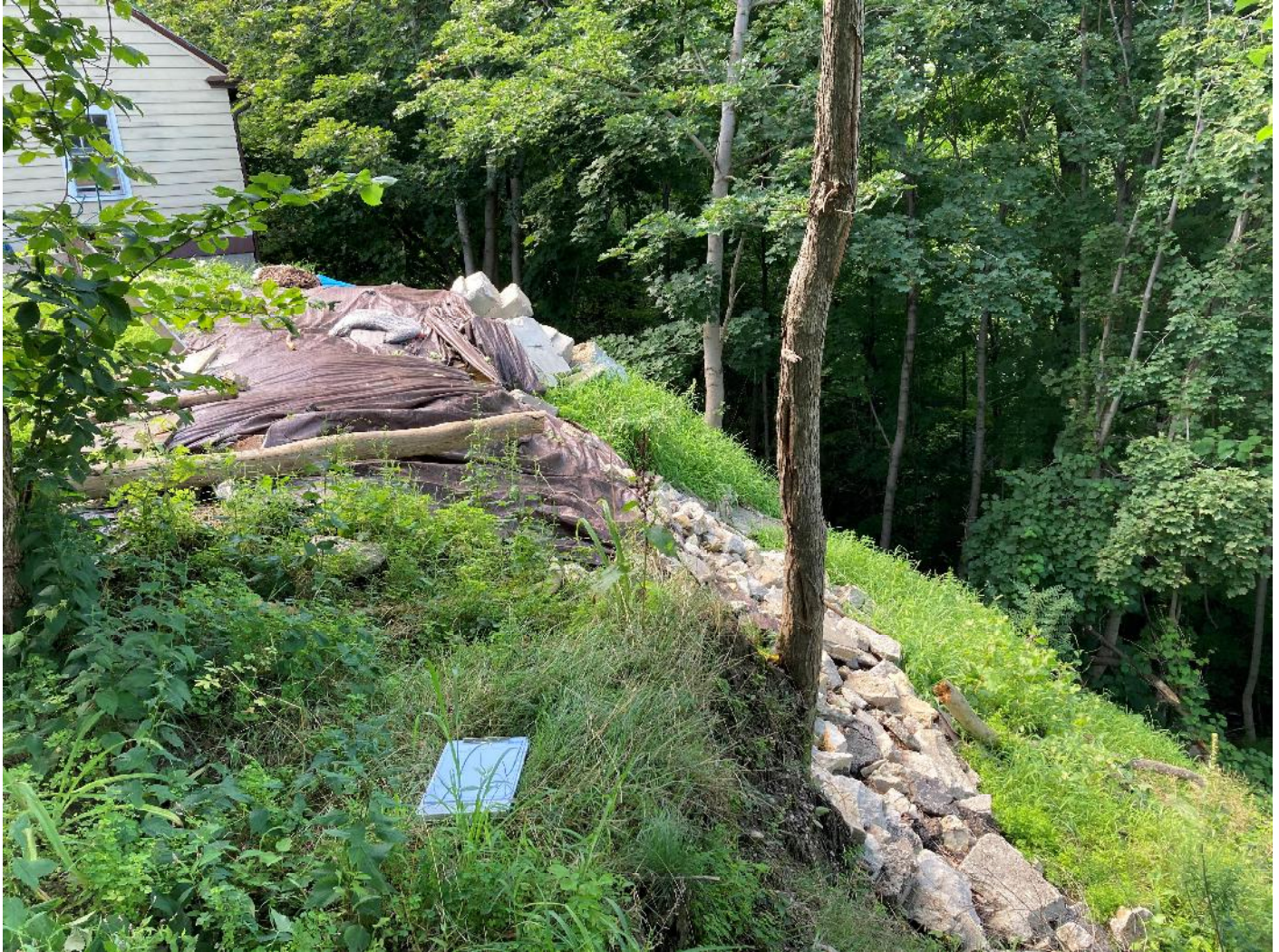
Photograph 17: View to west northwest, additional view of rip-rap armor at top of slope east of residence
