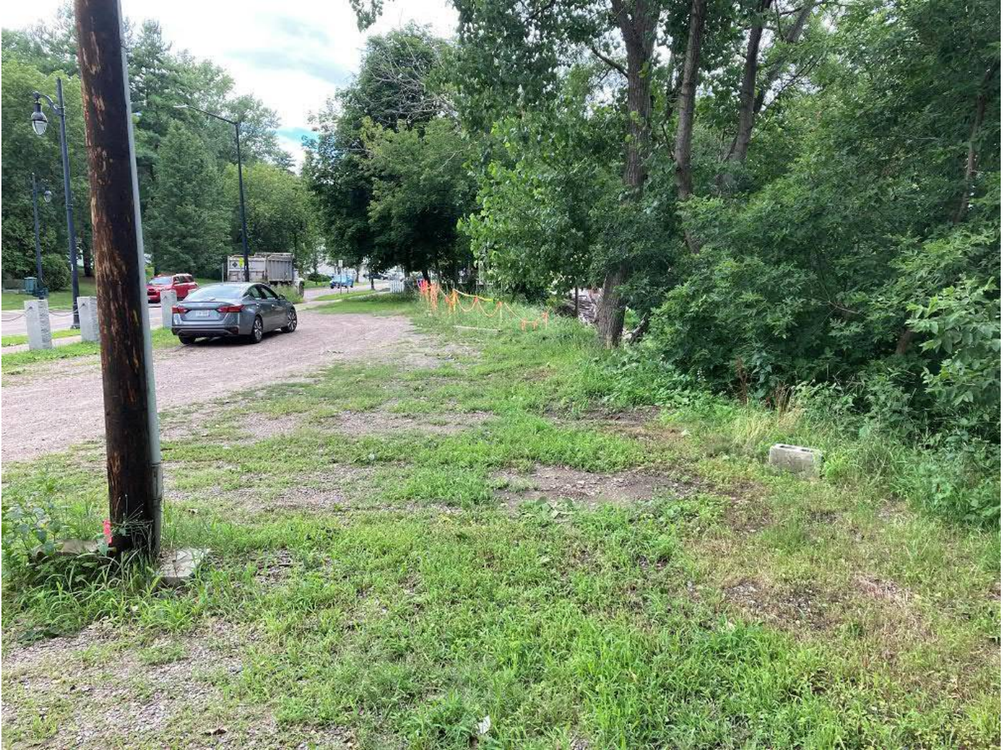
Photograph 23: View to west of top of slope between 365 Riverside Avenue (Hall's Hitches) and 389 Riverside Avenue (private residence – top center) showing stable platform at top of slope to left; incipient slumping possible at bottom-right and center-right of photograph; failed slope to right of stakes and flagging; exposed soil scarp obscured by vegetation at center-right of photograph.
