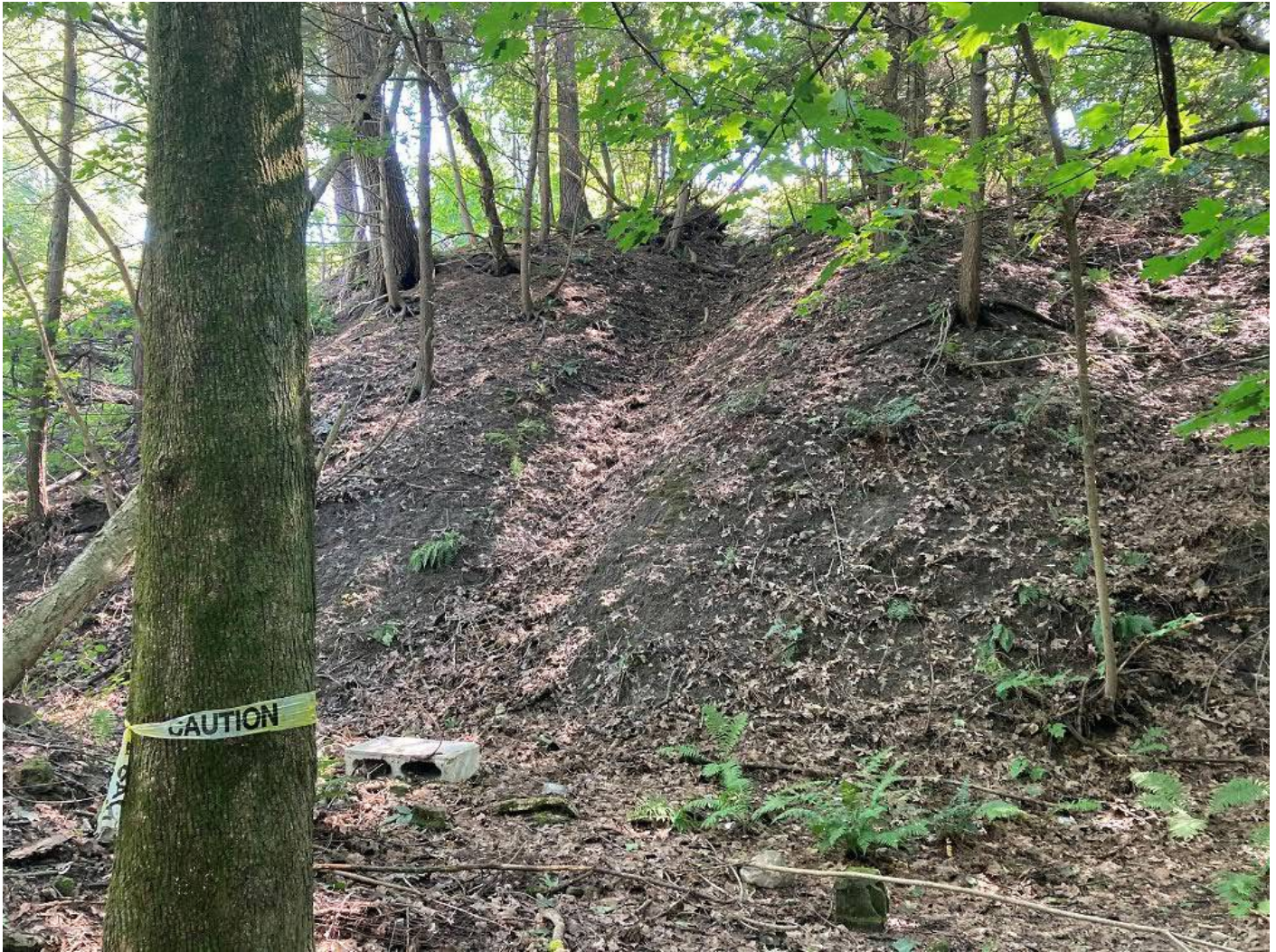
Photograph 21: View to south of exposed historic soil slump debris downslope from residence at 389 Riverside Avenue; exposed soil subject to continual erosion during precipitation events; note gully formation from surface runoff at center and right of photograph
