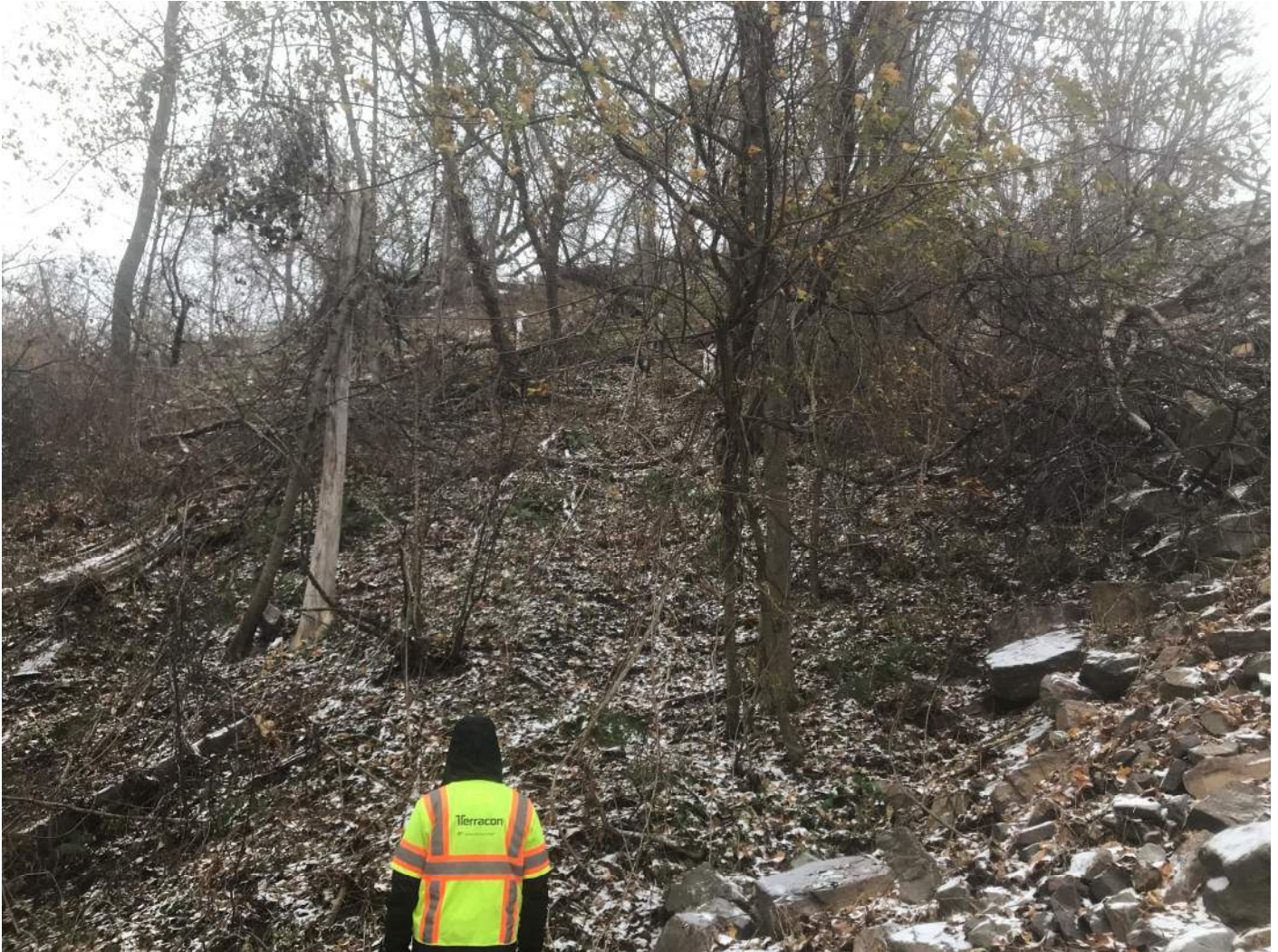
Photograph 4: View to south-southeast of natural vegetated slope on eastern flank of remediated slope
