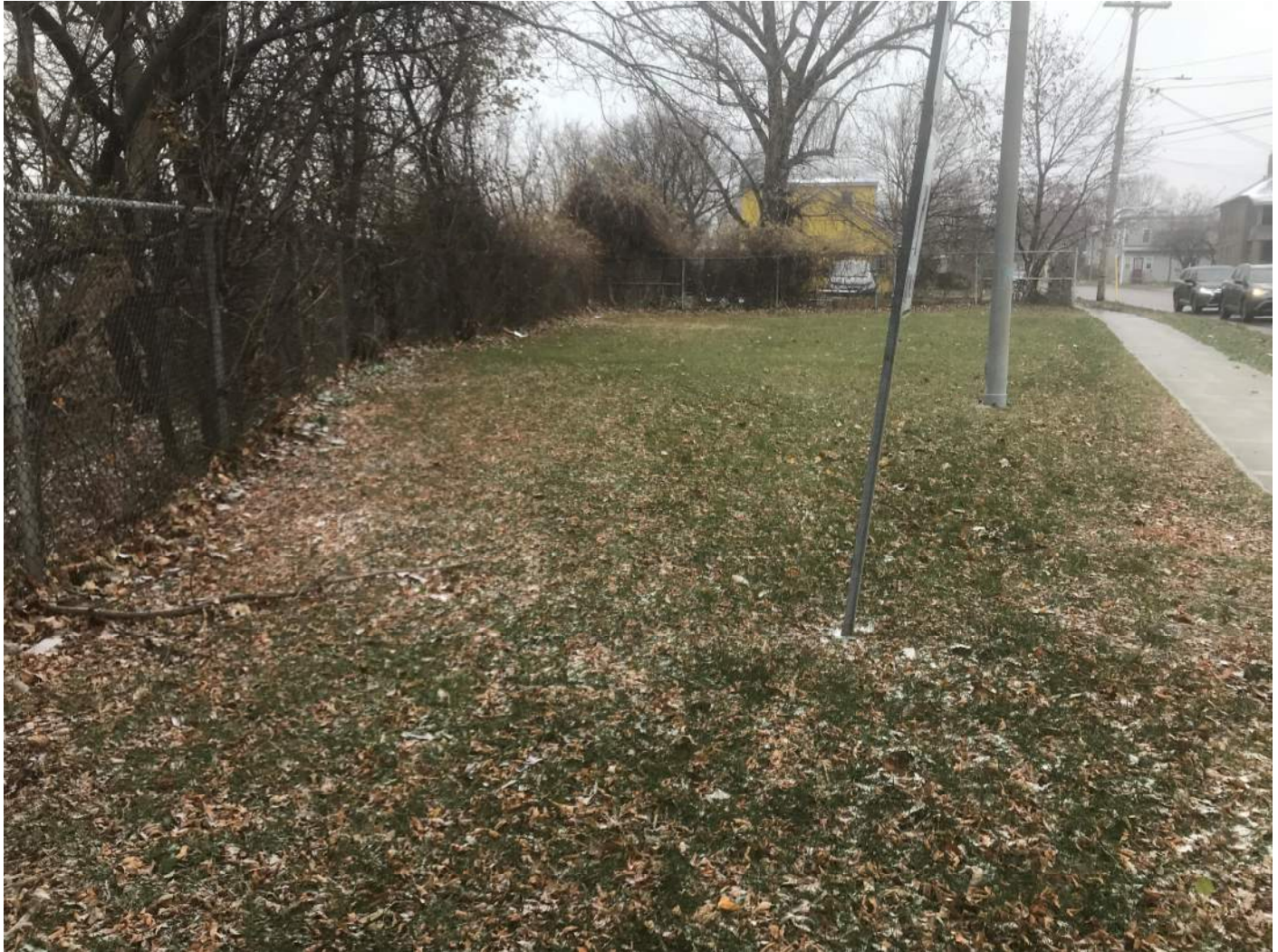
Photograph 14: View to east showing top of natural slope on eastern flank of remediated slope; no distinct signs of stress cracking, slumping or movement evident
