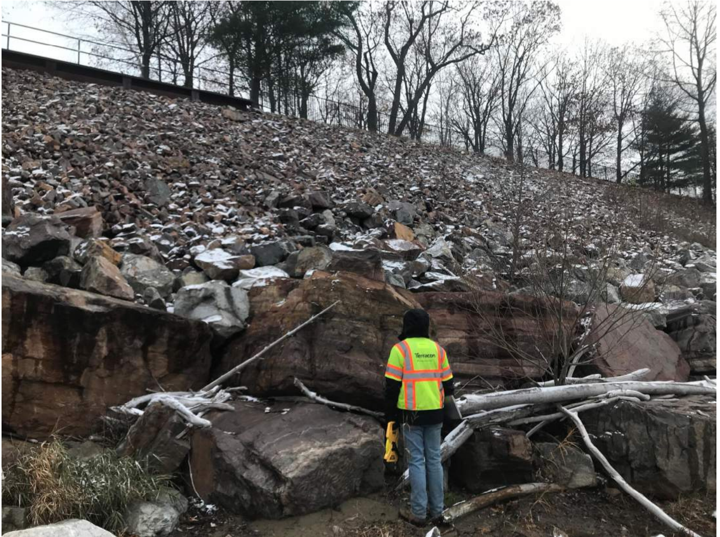
Photograph 2: View to east of central portion of remediated slope showing cobble and boulder rip-rap armor and large basal blocks; bike path is located beyond fence; slope appears stable
