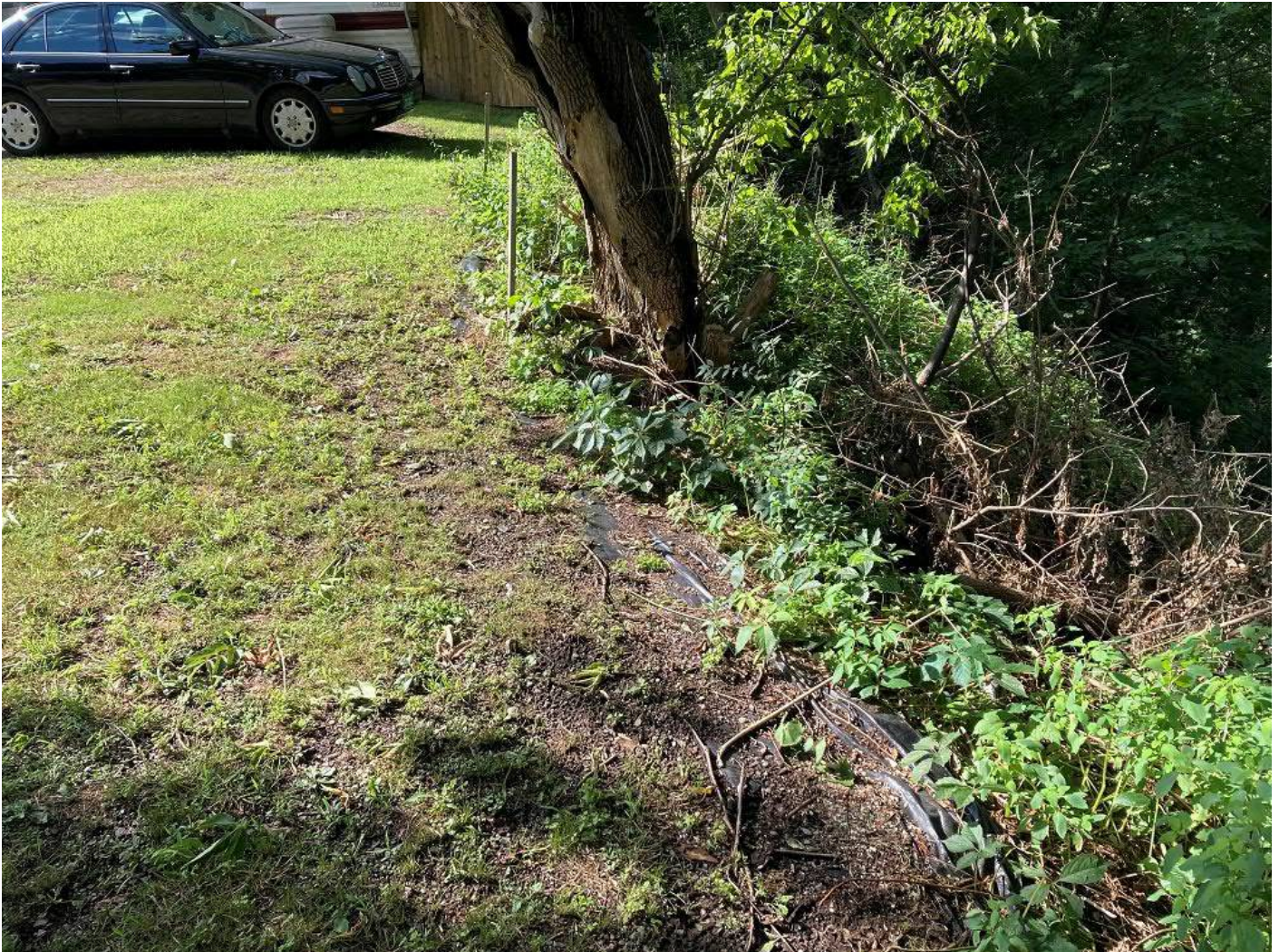
Photograph 21: View to northwest from eastern portion of Michael's Auto Sales property showing remediation implemented by landowner, including placing of geotextile fabric and pea-stone ballast; soil scarp occurs beyond and obscured by vegetation to right.
