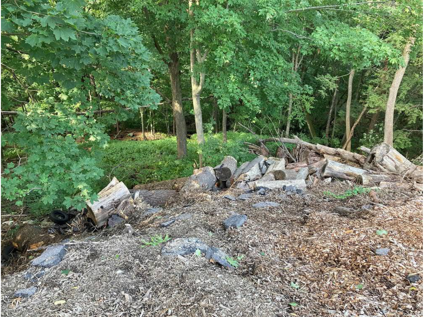
Photograph 7: View to north downslope from crown cracks at top of slope east of Burlington Collision building; logs appear to be placed to stabilize slide; overgrown historic slump/slide debris apparent beyond logs;
