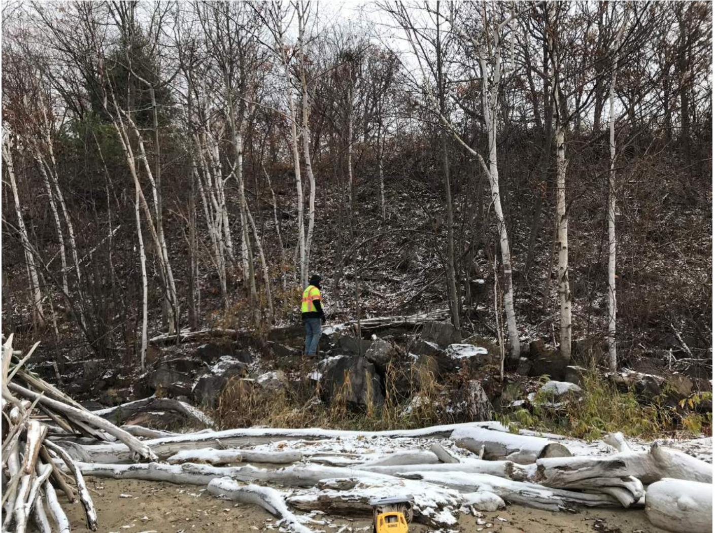
Photograph 4: View to south of vegetated natural slope on south flank of remediated slope
