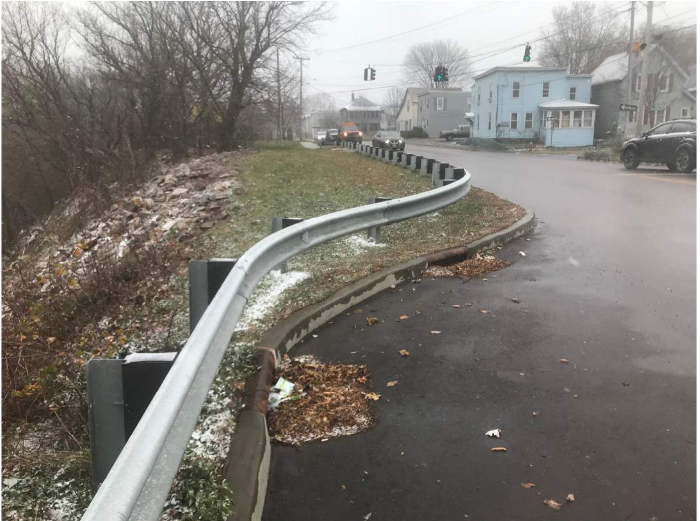
Photograph 12: View to east along Manhattan Drive showing top of remediated slope; pavement and grassy areas show no signs of distress or transverse cracking indicative of movement; guard rail appears stable and shows no sign of movement
