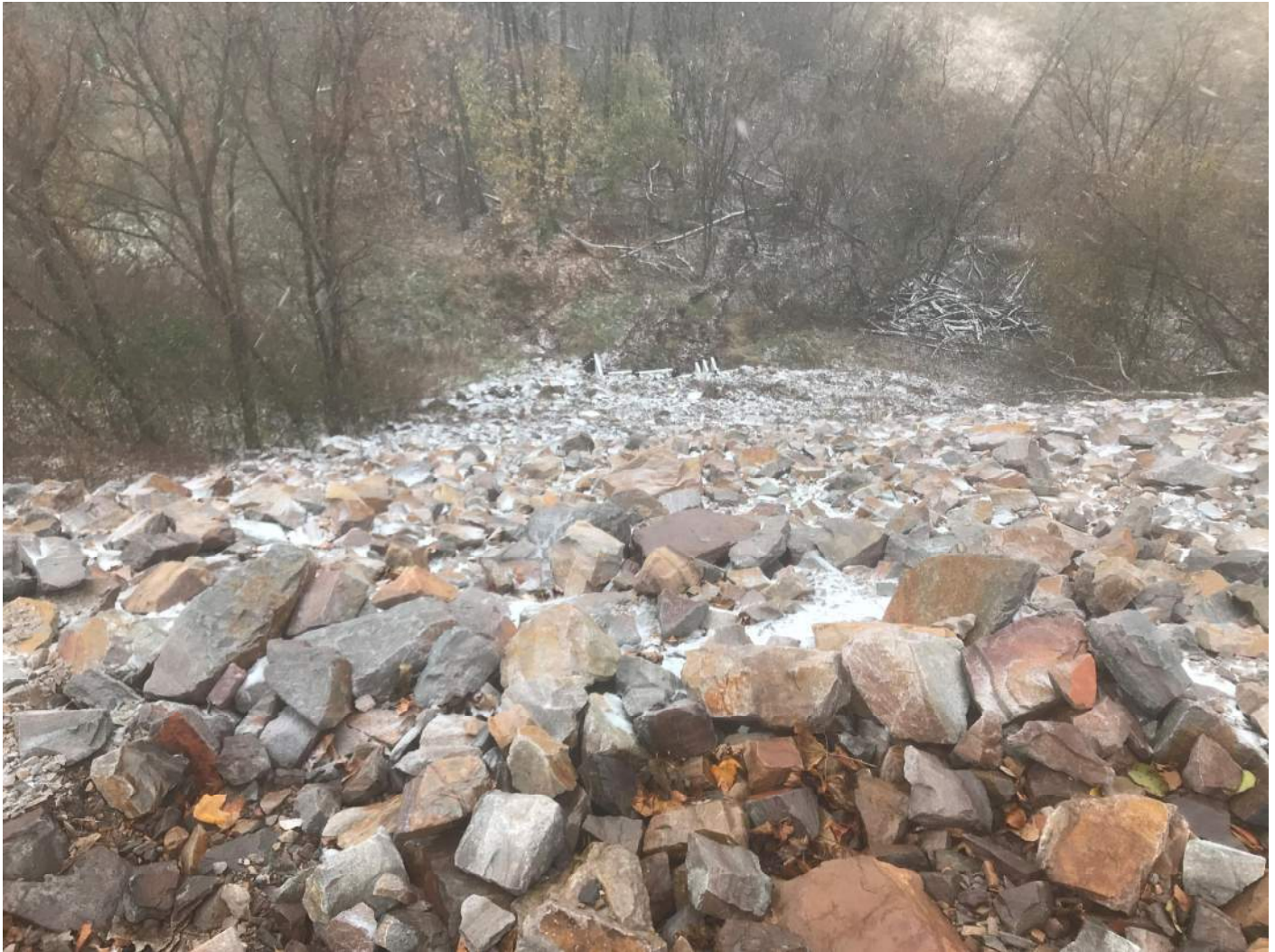
Photograph 11: View to north showing stability, nature and size of rip-rap armor on remediated slope
