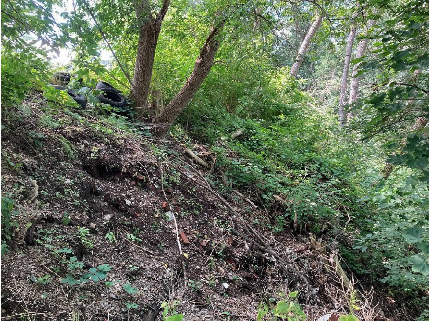
Photograph 30: Additional view to west of eroded slope between 365 and 317 Riverside Avenue; note brick fragments and density of vegetation to west; (photograph taken from 317 Riverside Avenue property – Bluebird BBQ west parking area)
