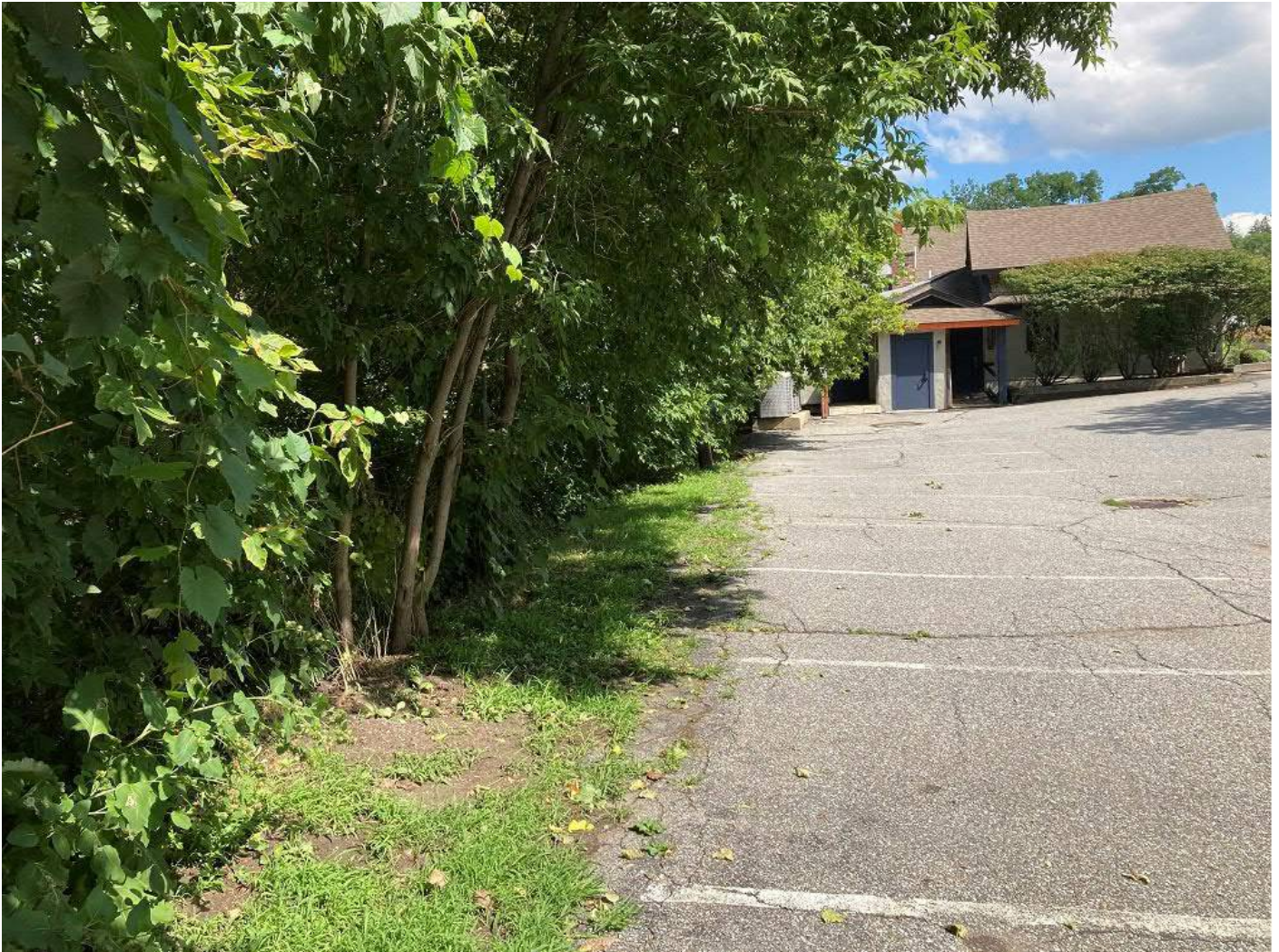
Photograph 1: View to east, toward Bluebird BBQ building from boundary between 317 and 365 Riverside Avenue properties, showing top of slope and absence of distinct surface expression of slump formation or crown cracking; stressed pavement cracks are a possible indicator of ongoing creep; note catch basin at right center of photograph; washout and gully formation from excess surface flow can be seen at bottom left of photograph
