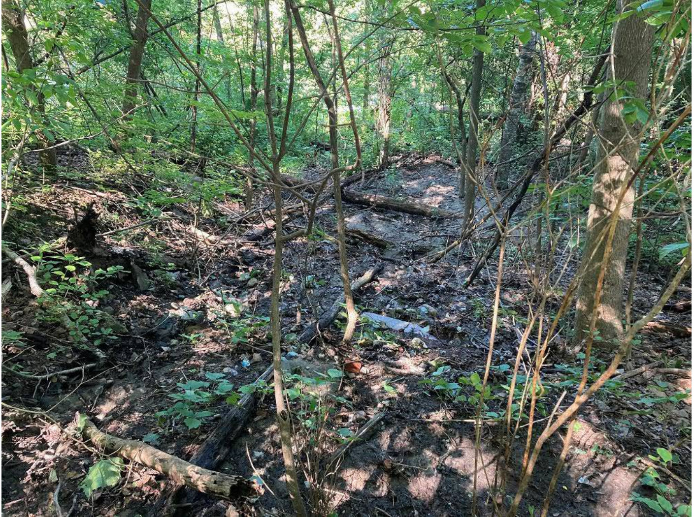
Photograph 14: View to north downslope from near position of Photograph 13 showing surface erosion effects from upslope surface water discharge
