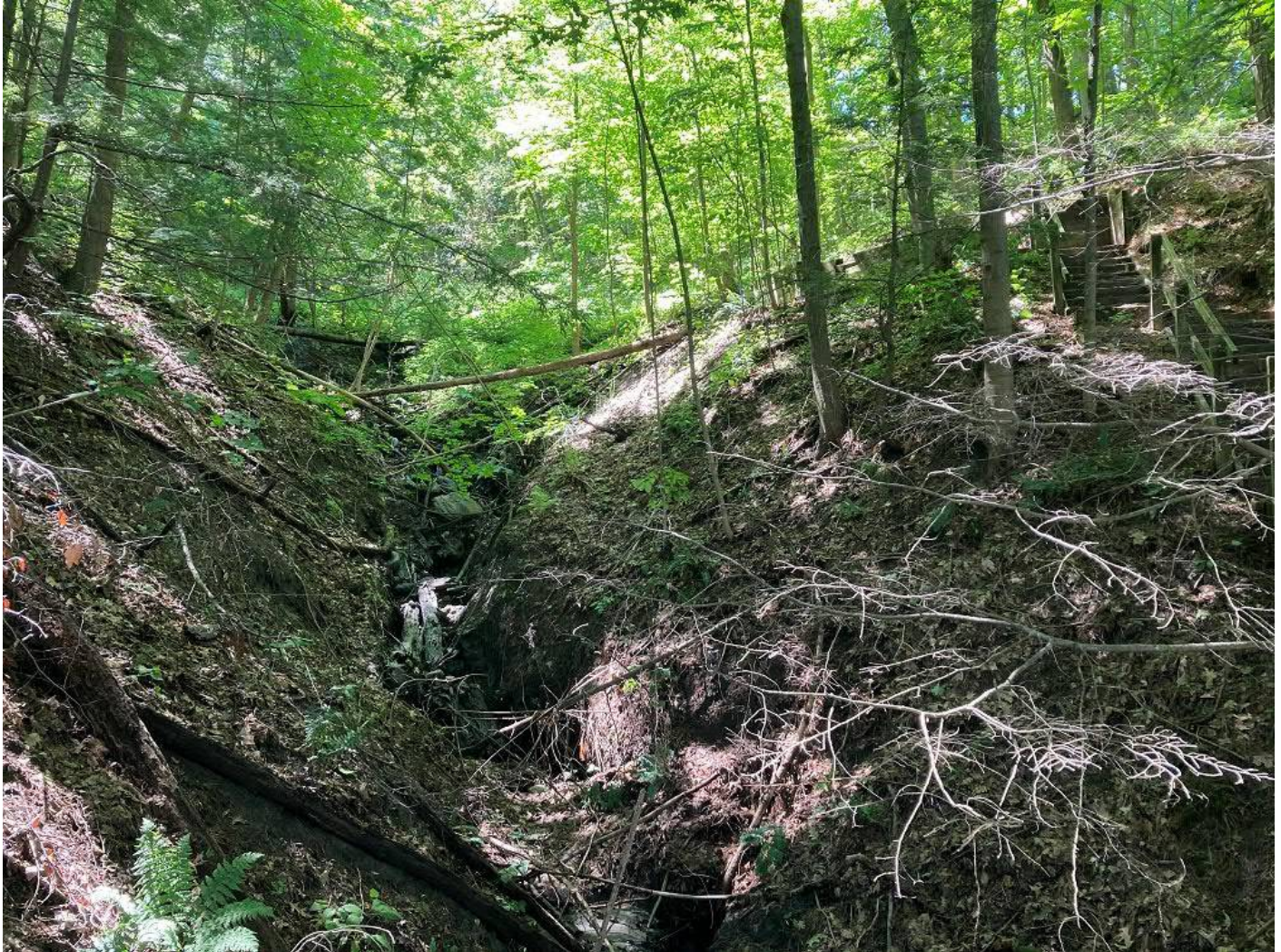
Photograph 5: View to south southwest, downslope from and north of 505 Riverside Avenue, showing erosional gully formed by runoff and/or discharge from top of slope; unvegetated slopes subject to continued erosion during precipitation events; note stairs to right leading from Intervale Road to River Walk trail
