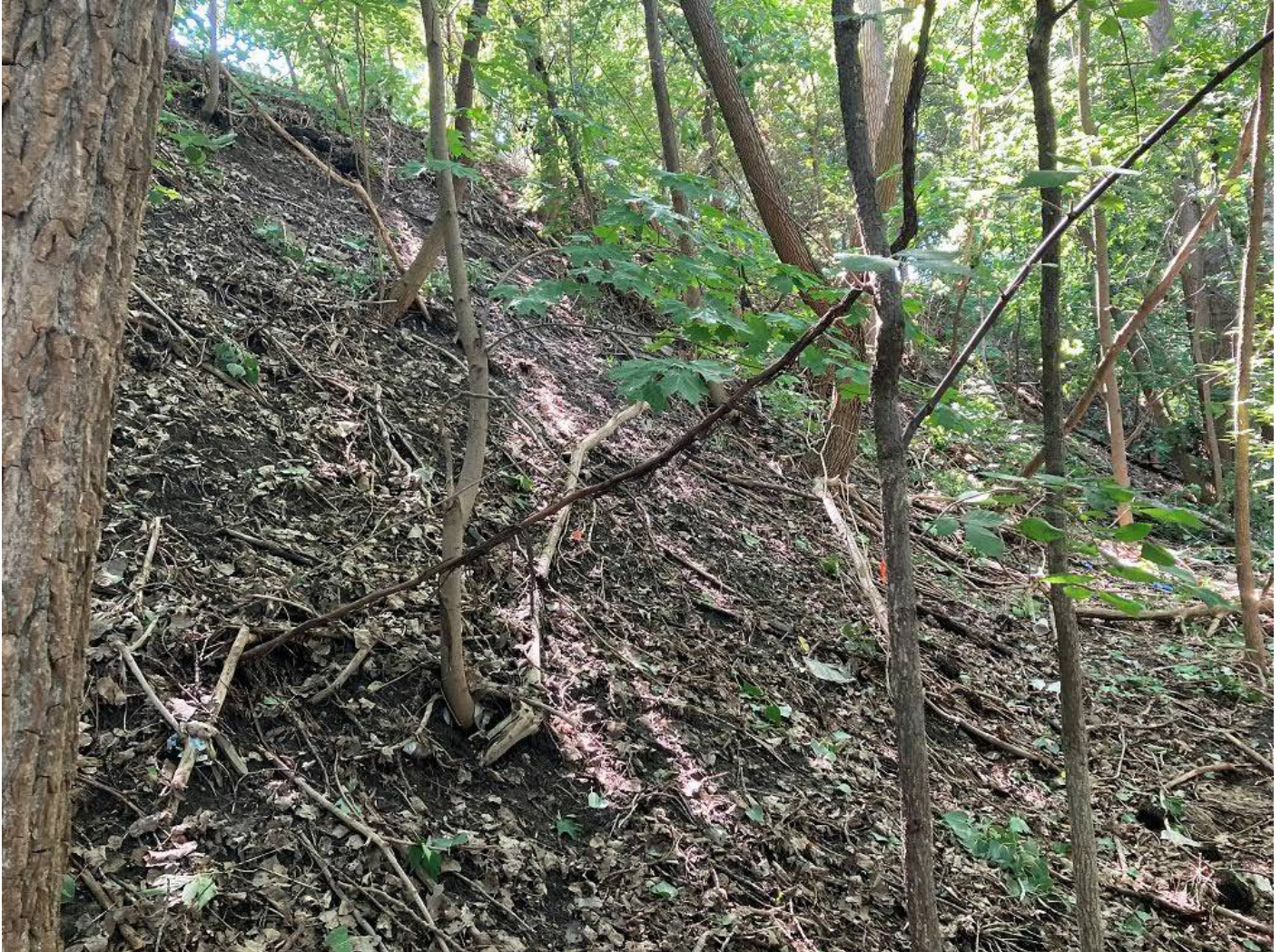
Photograph 11: View to southwest of top of slope just to the west of the Bluebird BBQ building showing soil surface exposed to continual erosion during precipitation events; soil scarp present at top left of photograph
