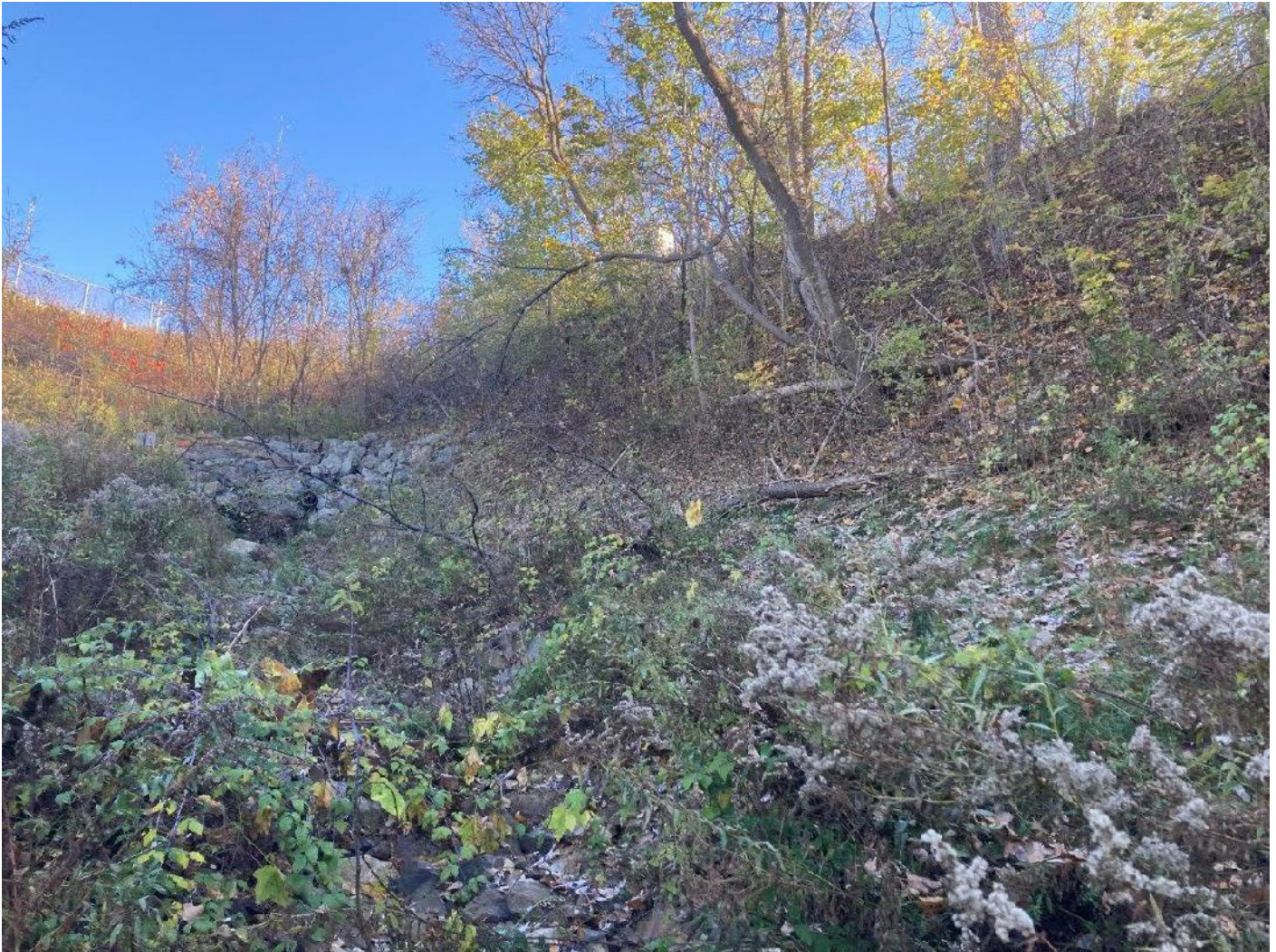
Photograph 1: View to southeast, toward intersection of Manhattan Drive and Route 127 showing stormwater discharge point (designated herein as Culvert 1) and stone-lined drainage channel.
