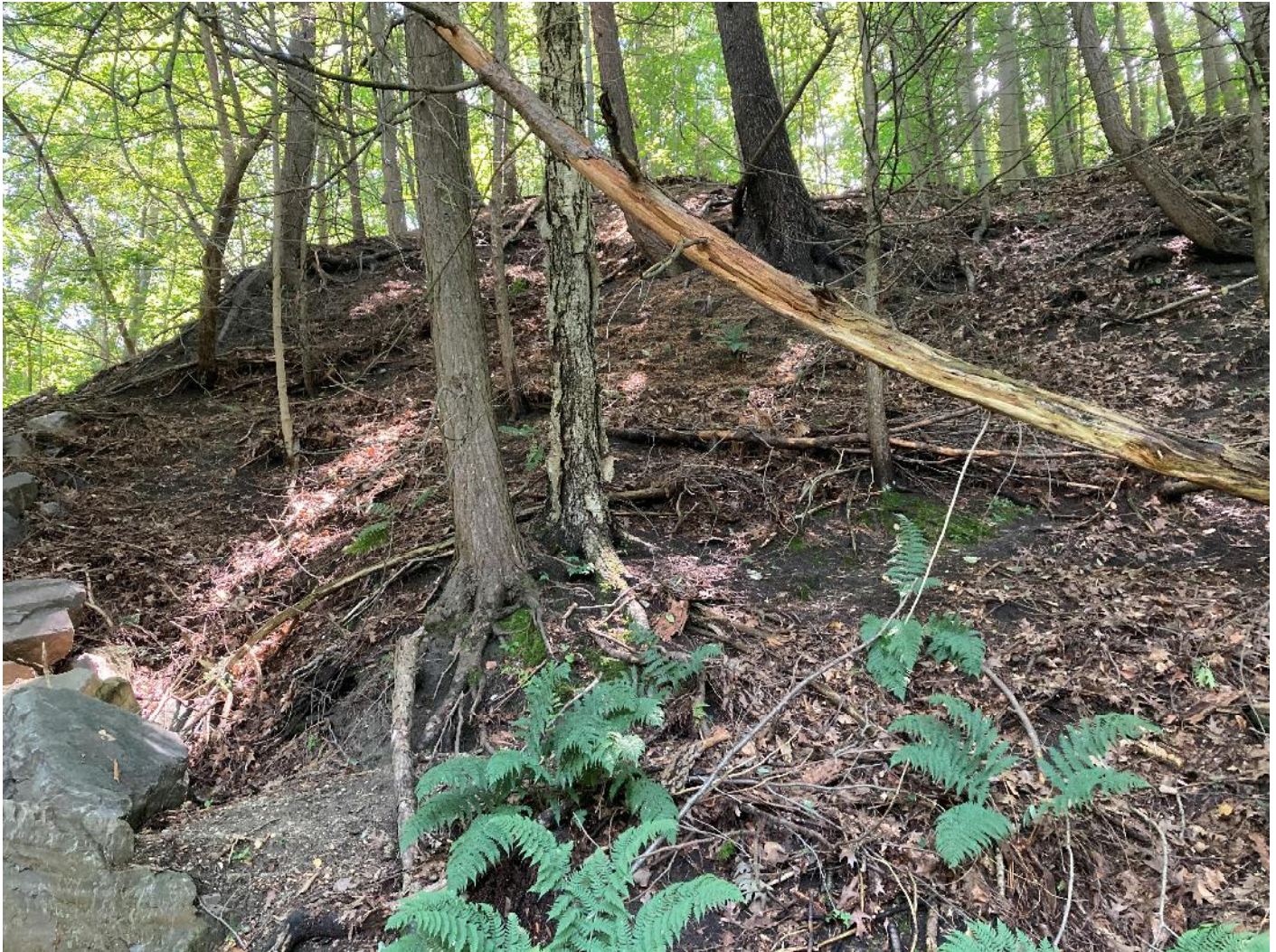
Photograph 26: View to southeast downslope from Michael's Auto Sales; gullies evident top right and top left provide conduit for surface flow; poorly vegetated slope continues to erode during precipitation events
