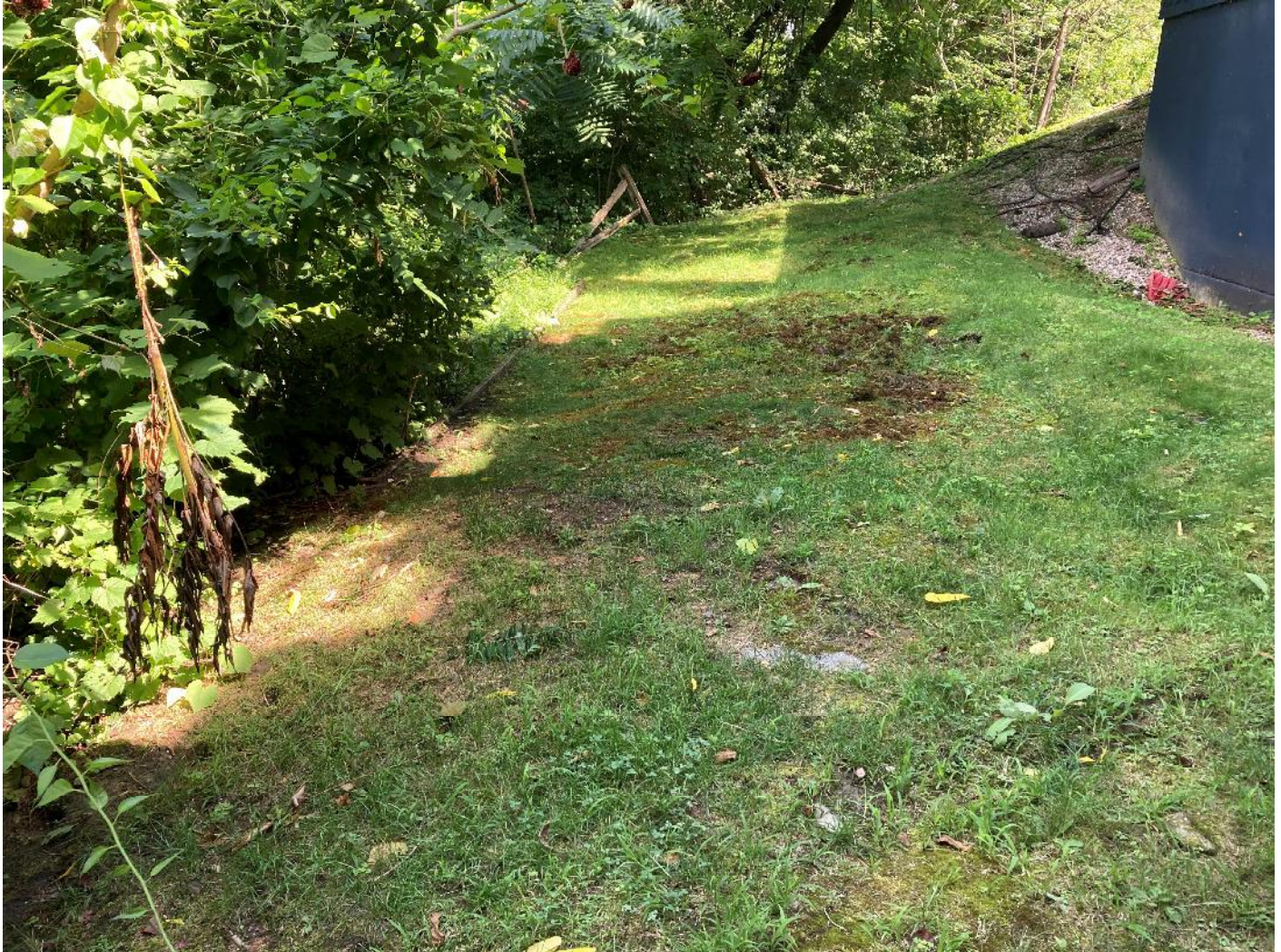
Photograph 7: View to east behind Bluebird BBQ building showing well vegetated stable platform with no evidence of surface cracking or slumping; however, note failed fence at top center of photograph
