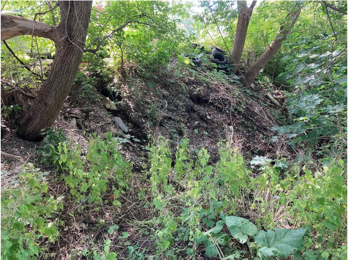
Photograph 29: View to southwest of eroded slope at eastern boundary between 365 Riverside Avenue and 317 Riverside Avenue (Bluebird BBQ); brick fragments within mass indicate historic filling; note gully formation at left and lean of trees at extreme left and top right; exposed soil subject to continual erosion and gully formation during precipitation events (photo taken from 317 Riverside Avenue property).
