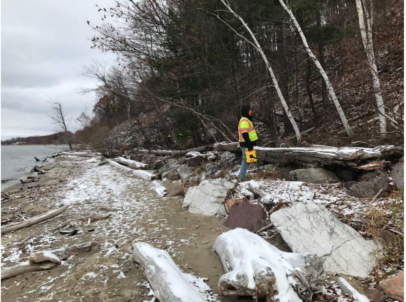
Photograph 5: View to north; base of natural slope on southern flank of remediated slope; remediated slope is shown in the background; note lean of birch trees down-slope indicative of slope creep
