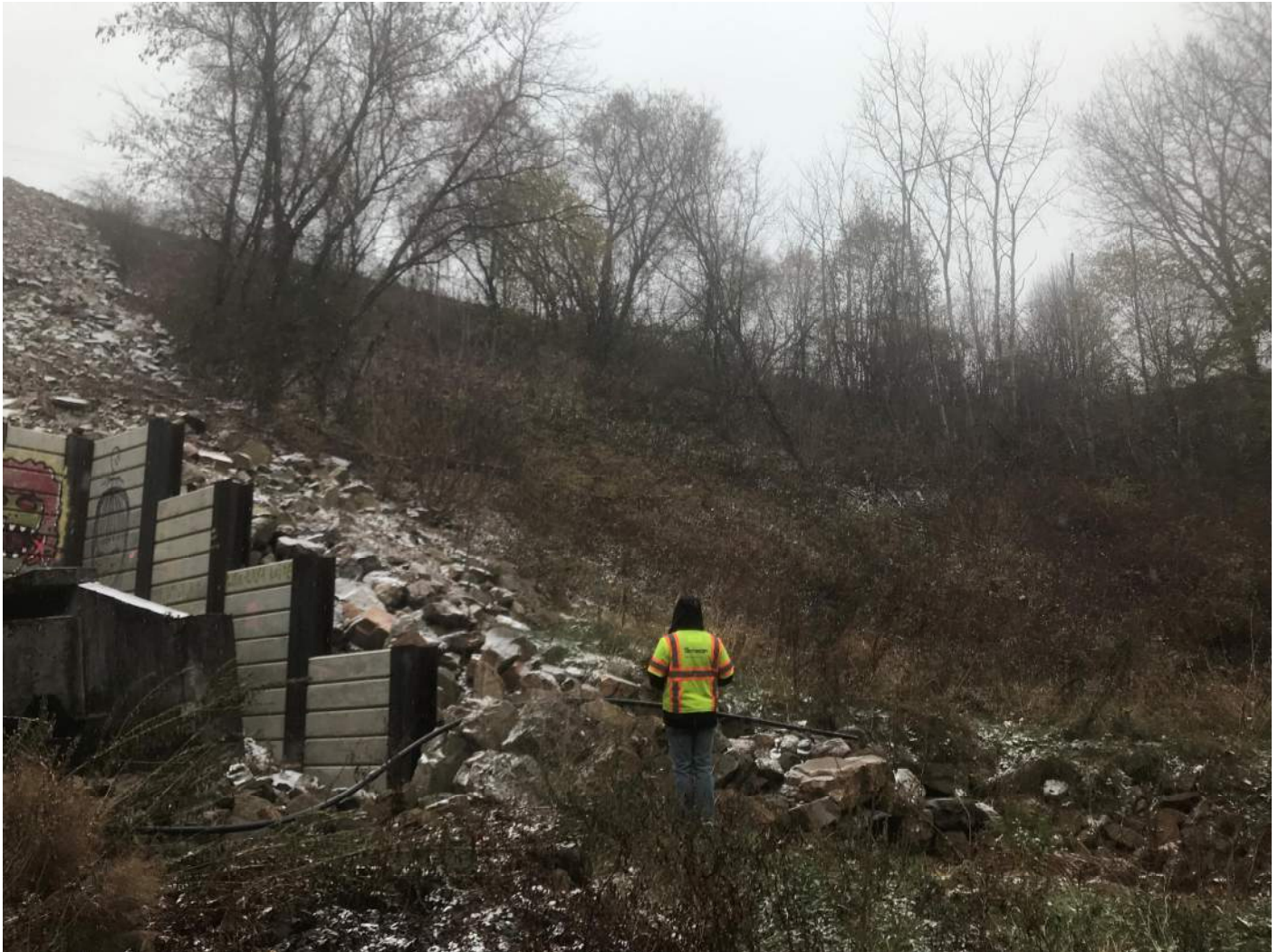
Photograph 7: View to southwest of natural vegetated slope on western flank of remediated slope; stormwater drainage outlet is shown left foreground
