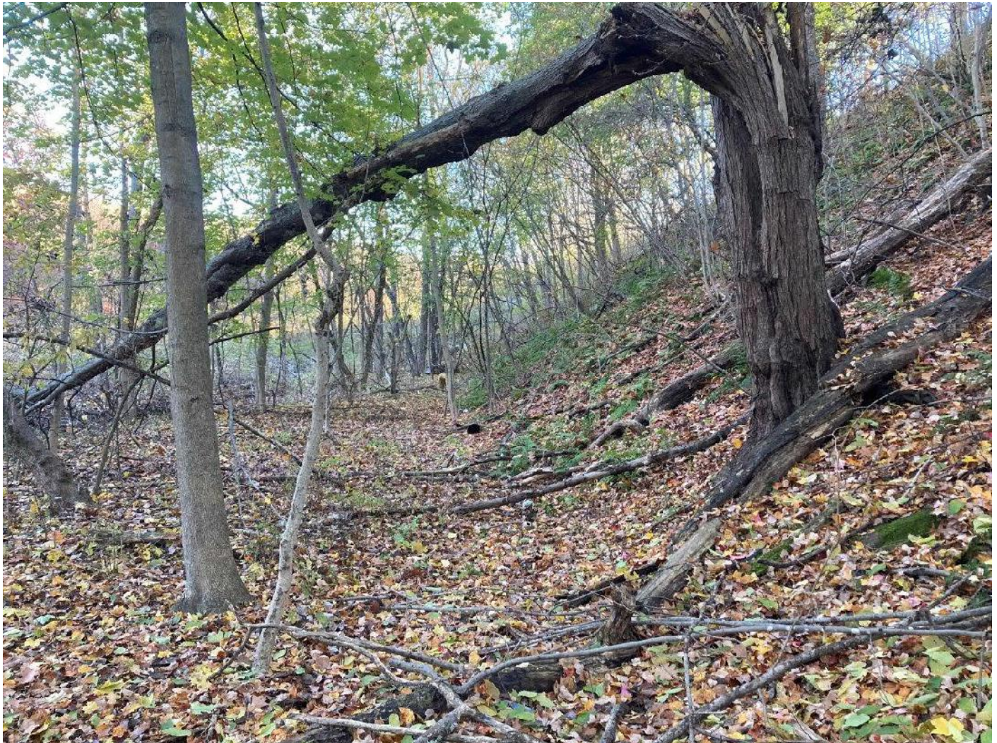
Photograph 11: View to east showing toe of slope west of Culvert 2 and east of Culvert 3; unlined discharge channel from Culverts 1 and 2 at left-center of photograph.
