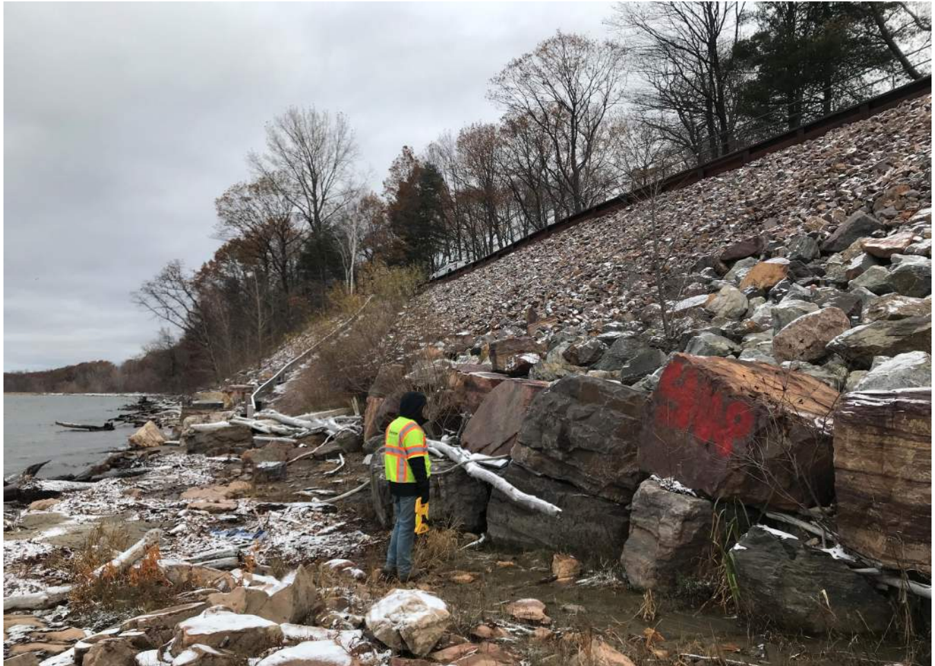
Photograph 1: View to north of northern section of remediated slope showing boulder and cobble rip-rap armor and large basal blocks; natural vegetated slope located to north of remediated area, and bike path at top of slope
