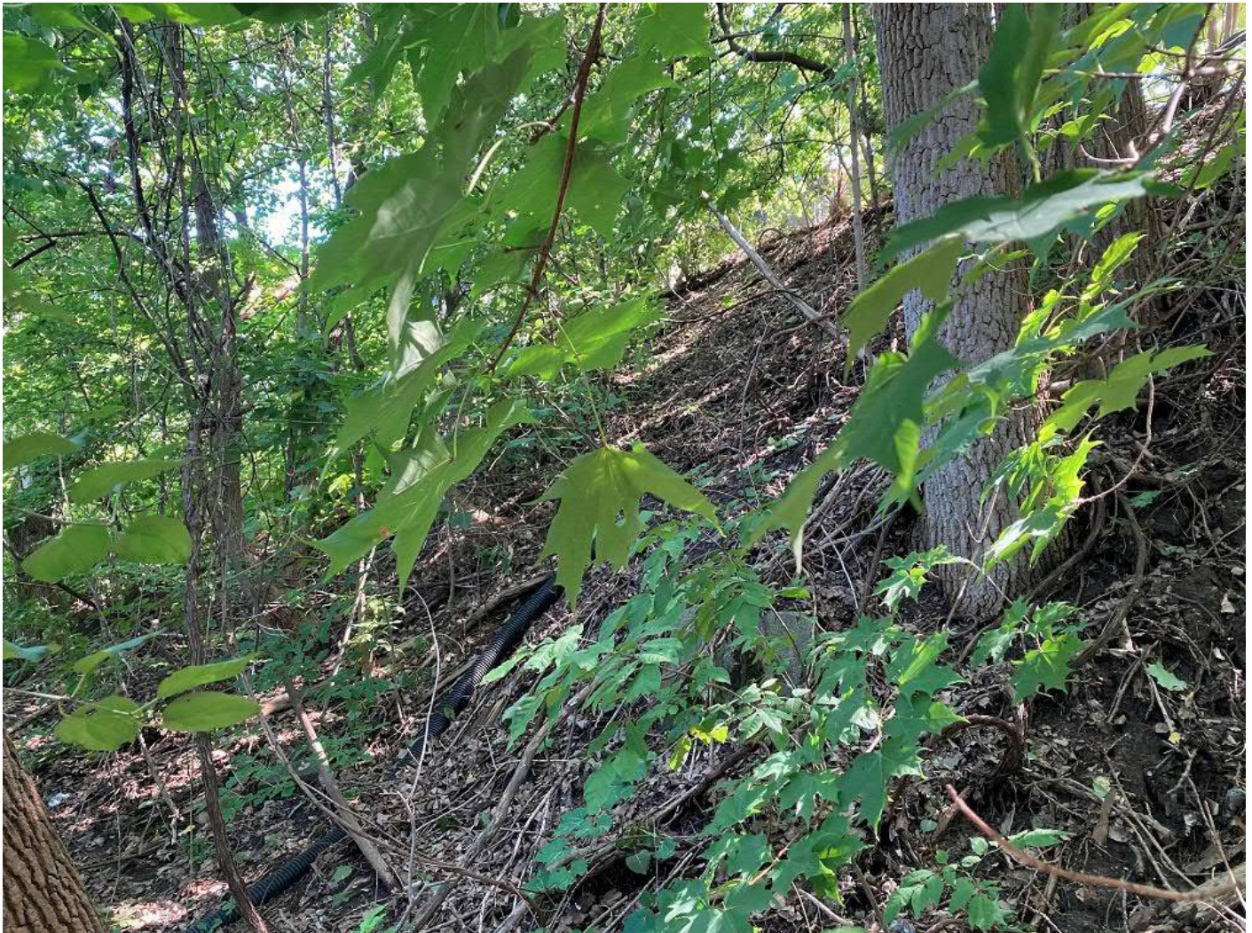
Photograph 12: View to southeast of exposed slope behind Bluebird BBQ building; exposed surface soil subject to continual erosion during precipitation events; note discharge hose left foreground; ongoing discharge downslope facilitates continual erosion of exposed surface soil
