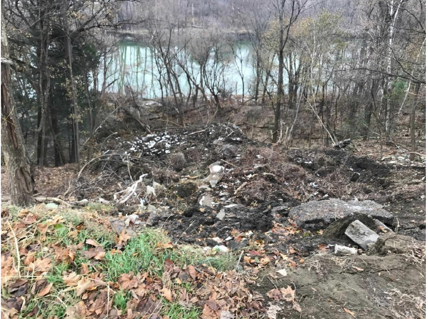
Photograph 19: View to north between 389 and 365 Riverside Avenue showing slide debris in December 2019 during inspection by Hoyle Tanner Associates; Photo 17 above shows same view taken in August 2020.
