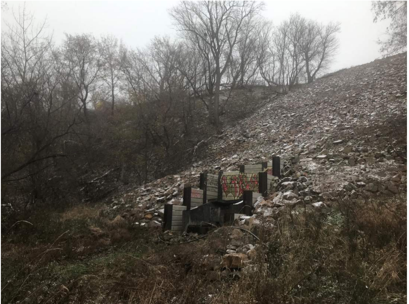
Photograph 3: View to southeast of remediated slope and natural vegetated slopes on eastern flank; stormwater drainage outlet in foreground
