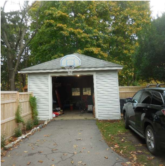
PHOTO 1: South Side - Note slight wracking of building to the left (west) side
