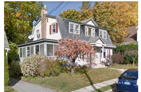
Principal structure, 40 Kingsland Terrace
