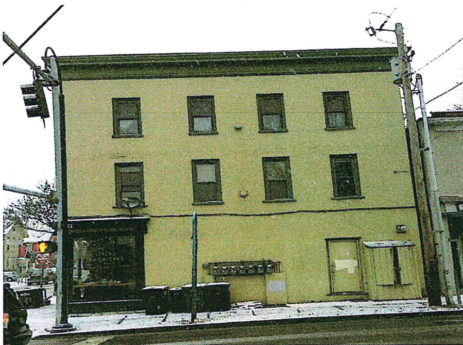
Date Taken: January 12, 2015 By: Marc A. O'Grady Direction: Northerly Identification: Southerly side of the building
