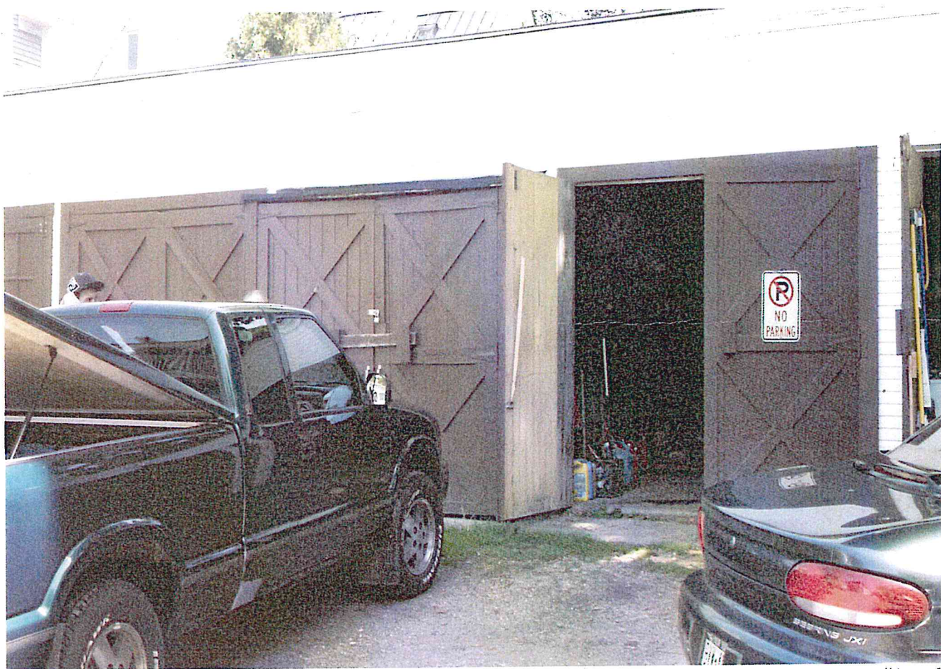
Storage of materials relating to repair and maintenance for other rental properties. Garage spaces #1 and 2 (southern edge of garage) are used for storage and maintenance space for all properties owned by Mr. Burns. Change of use from garage (conforming use) to private storage, without zoning approval.
