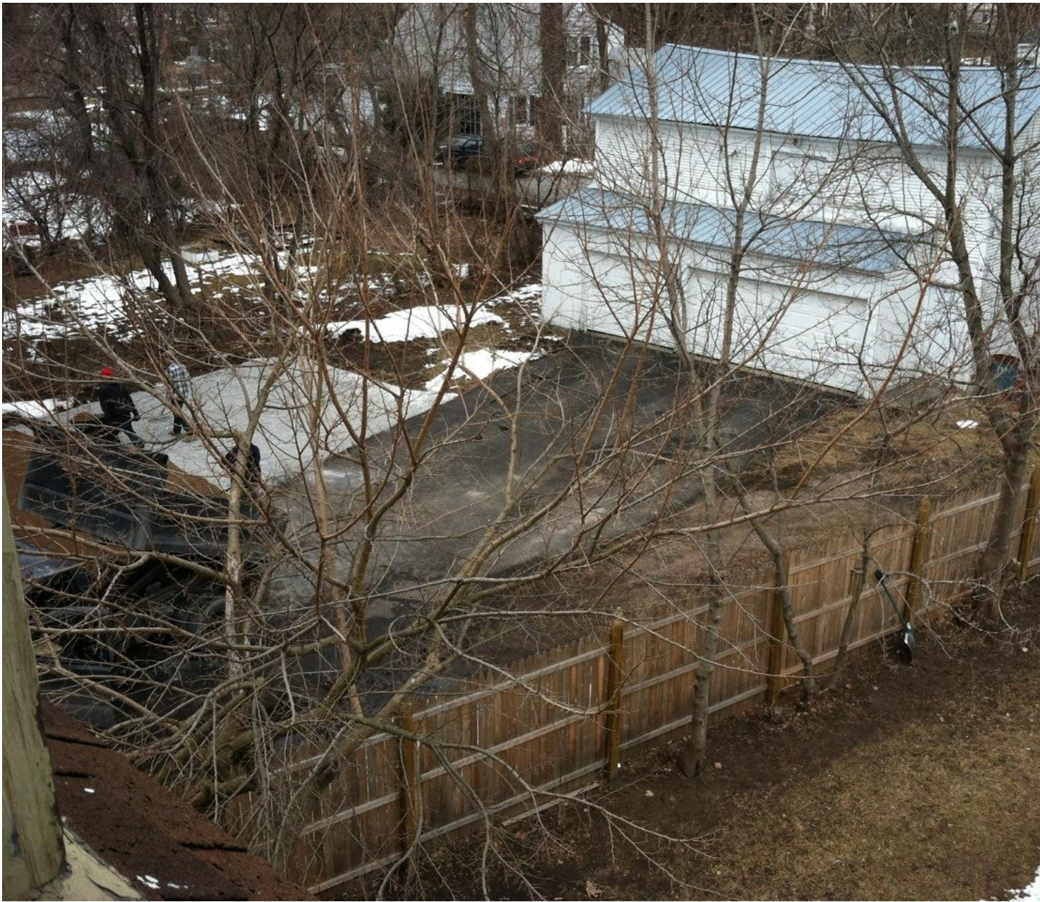
March 7, 2013 – dump truck in driveway of Property dumping gravel. Area south of driveway shows signs of disturbance but not parking.
