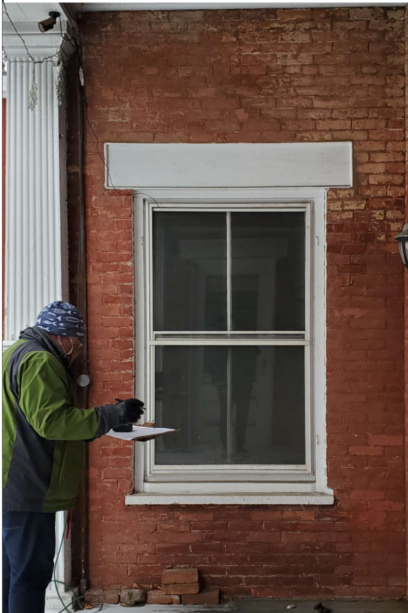
1-17 NORTH (FRONT PORCH)
