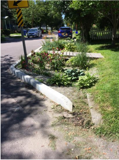
Mansfield Ave greenbelt bioretention system
