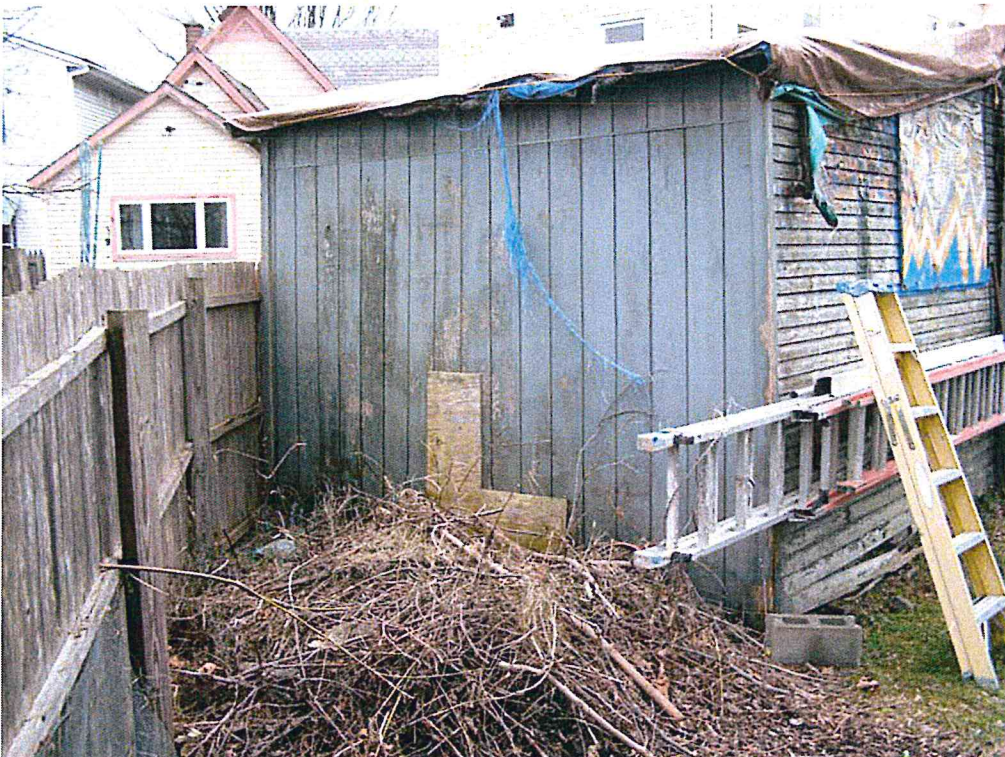
Photo 2 – West wall of the shed.
