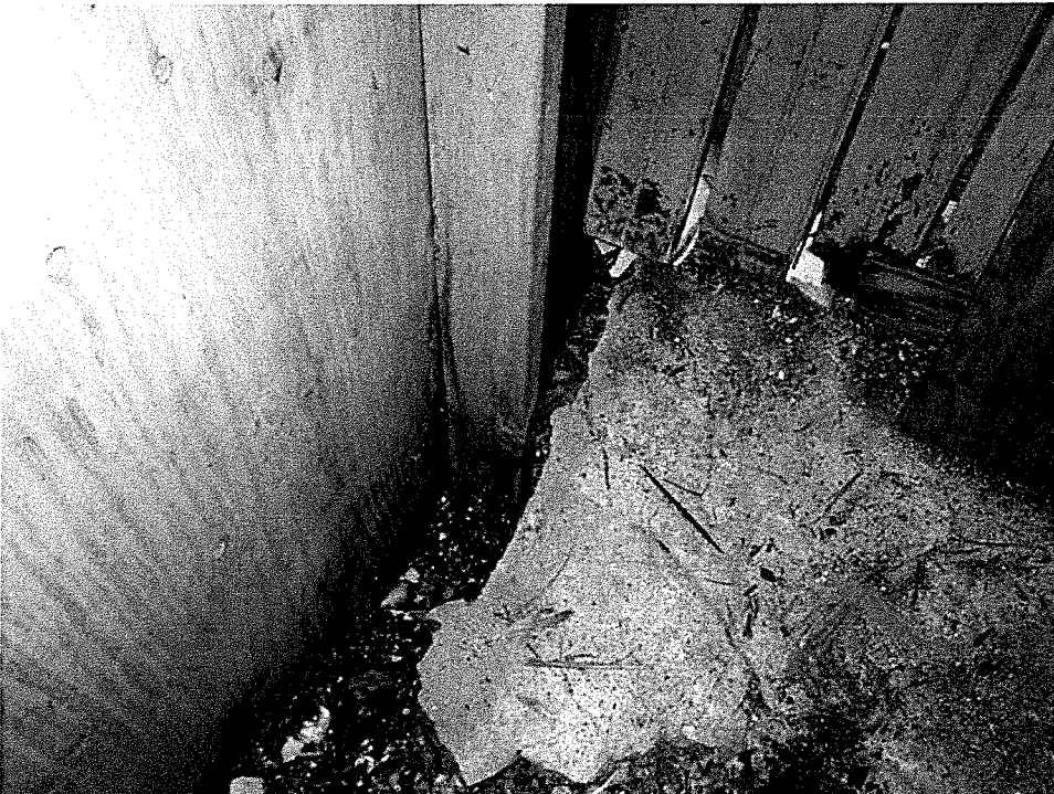
Photo 8 – Base of west wall looking towards the northwest corner.
