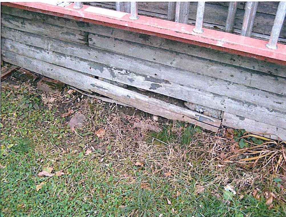
Photo 6 – South wall of shed.
