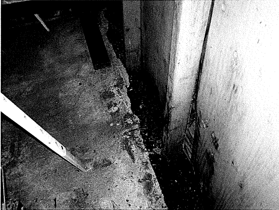
Photo 7 – Base of west wall of the shed. The wall is a bearing wall for the roof framing. There is not apparent foundation under the studs. The bottoms of the studs are rotted due to contact with the ground.
