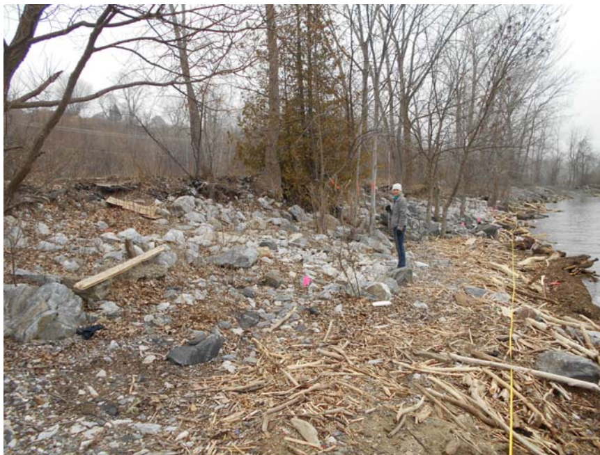
Photograph 2. View of shoreline just south of jetty in Urban Reserve. Actively eroding and receding shoreline can be seen at the top of the armor, photo left (Date: 3/16/16).
