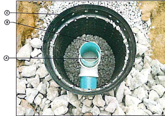
EXAMPLE OF AN OUTFLOW STRUCTURE
