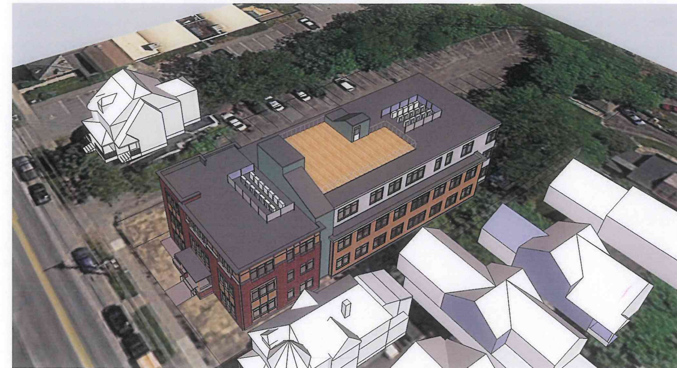
Aerial from Northwest
