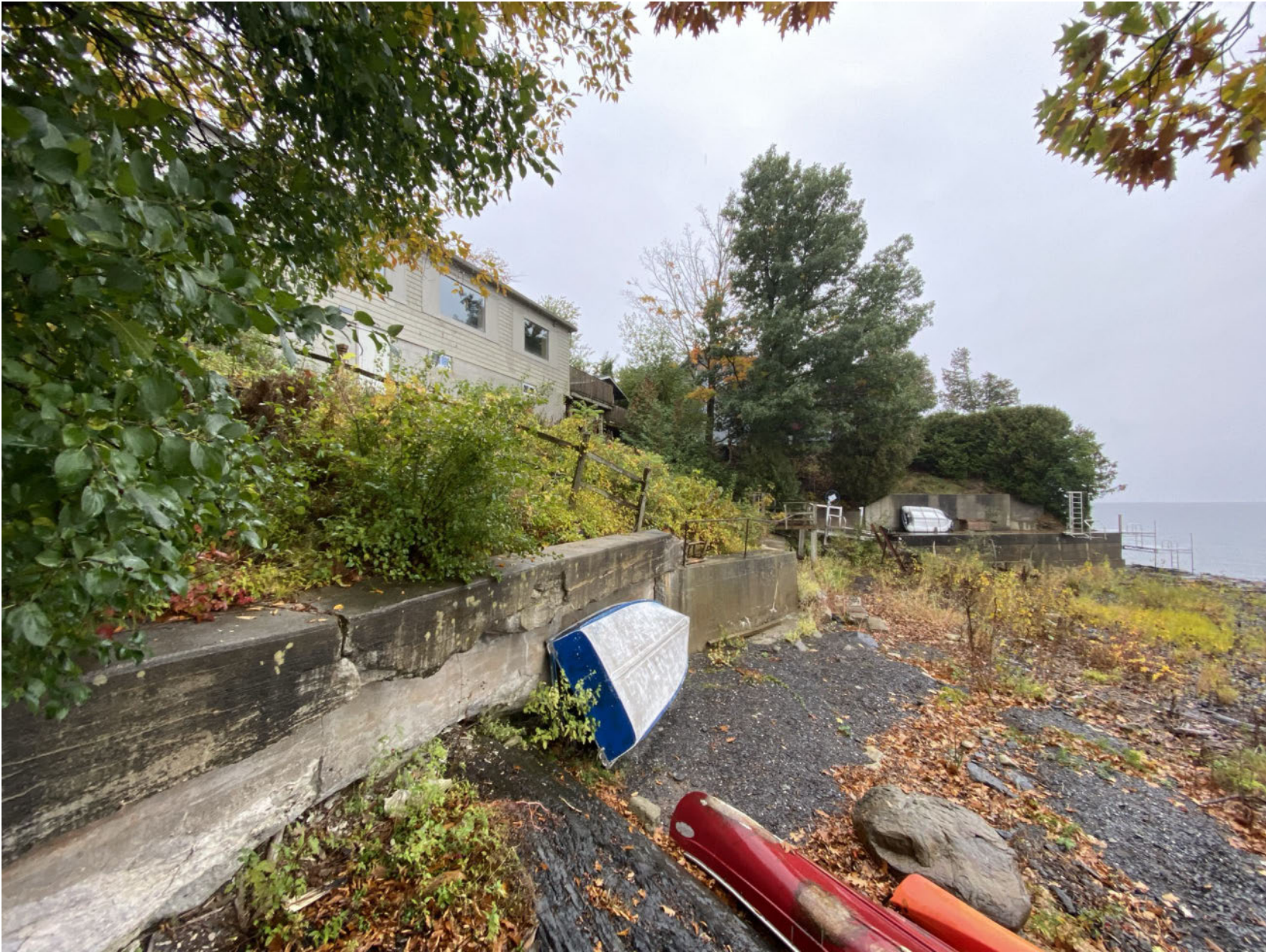
LOCATION 4 - LOOKING SOUTHWEST
