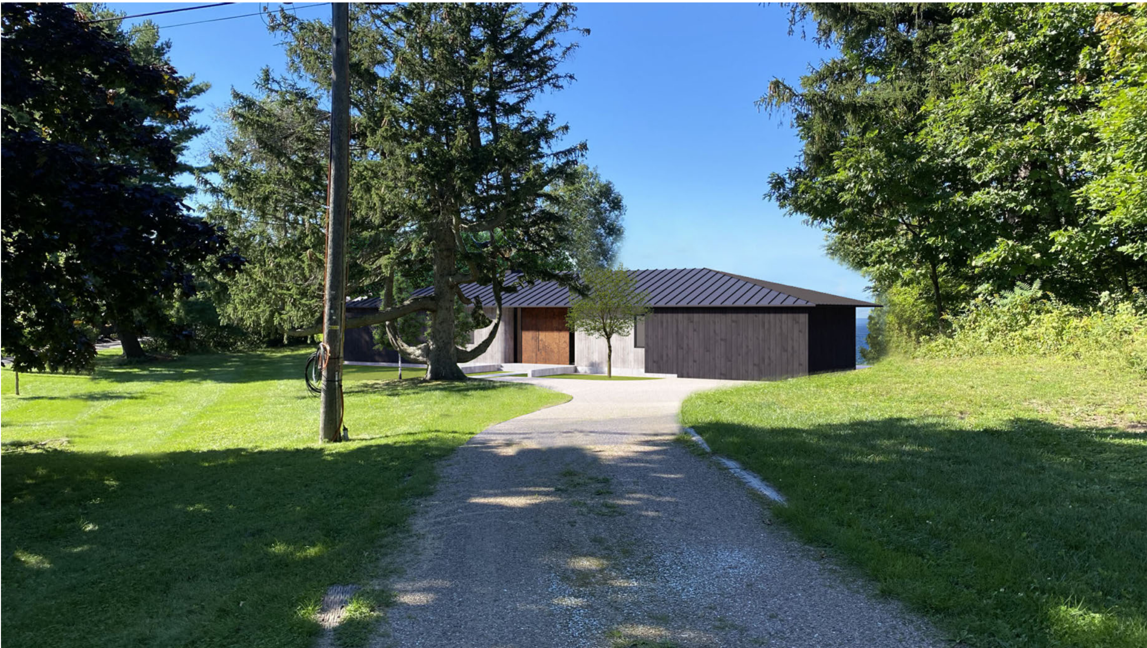
SOUTH FACADE - LOOKING WEST FROM DRIVEWAY APPROACH
