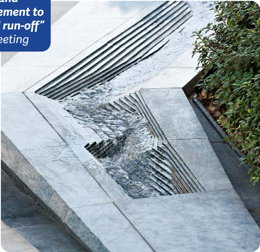
Sculptural reveals of stormwater that act as runnels during storm events
