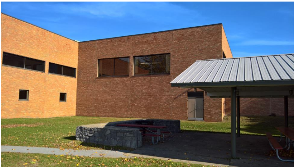
WATER TREATMENT PLNT AND PAVILION
